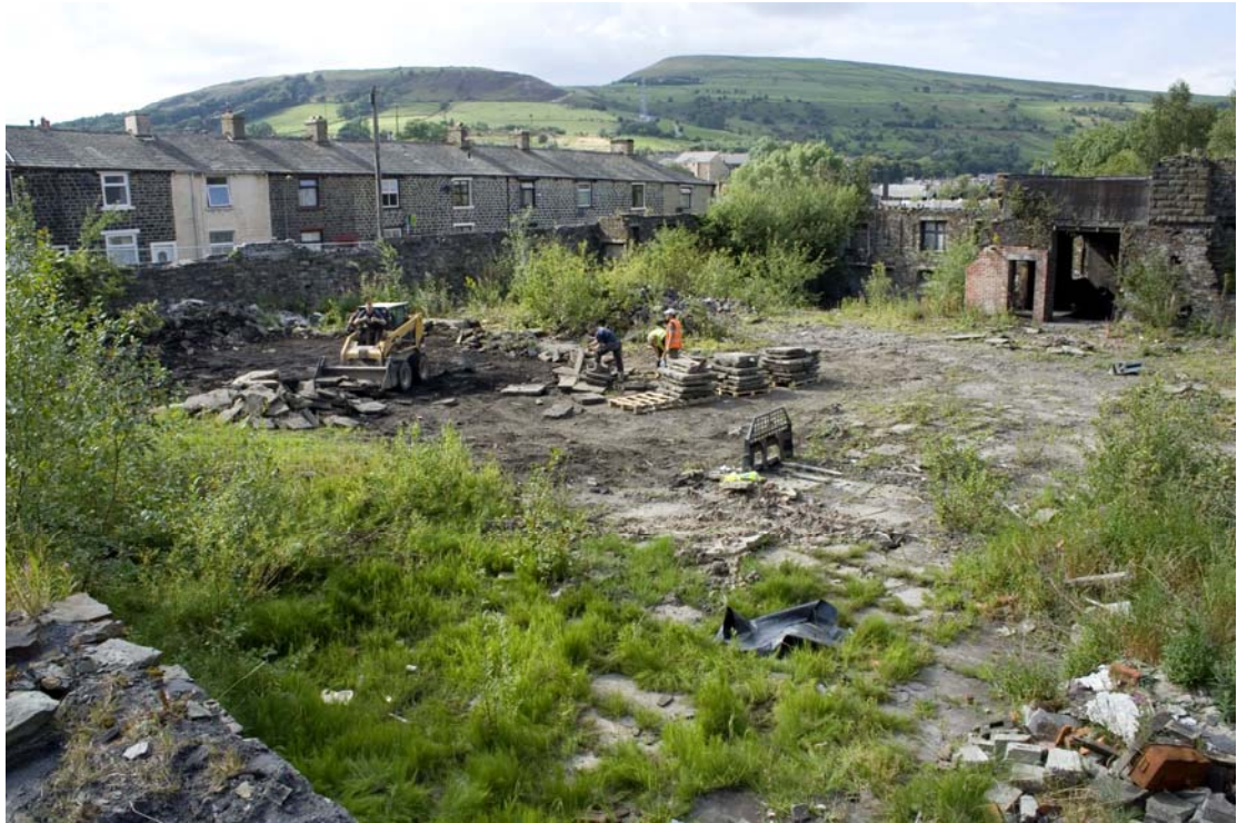
Plate 23: Removal of the flagged floor within the weaving shed, looking west
