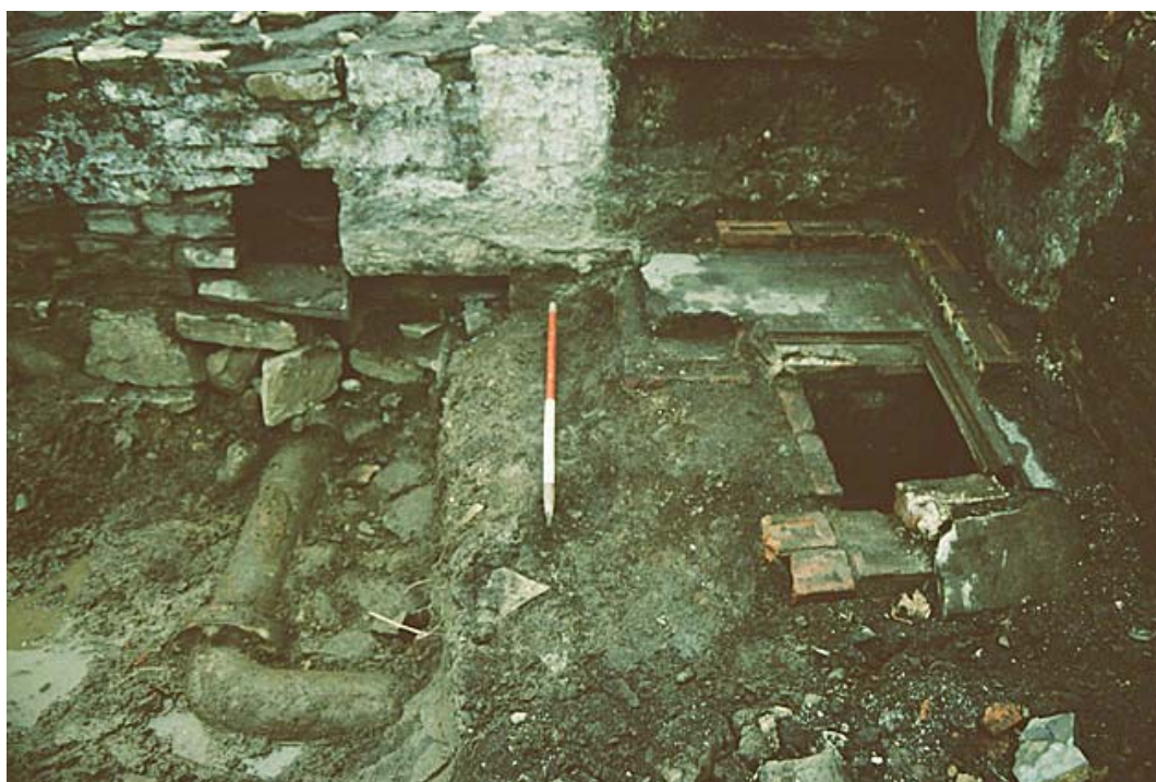
Plate 43: Exterior area, at the north-eastern end of wall 46 showing pipe 62 and manhole, looking north-east
