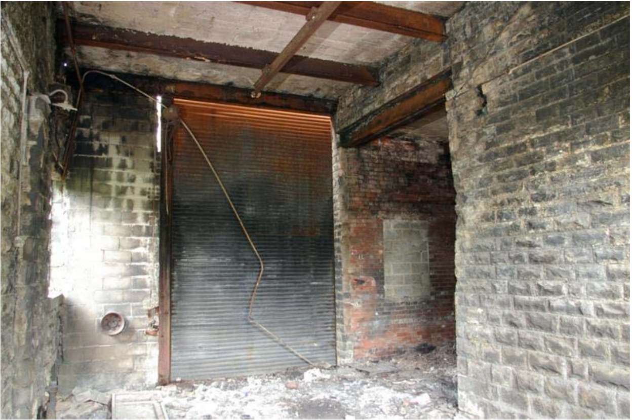
Plate 13: Interior of the loading bay, facing north
