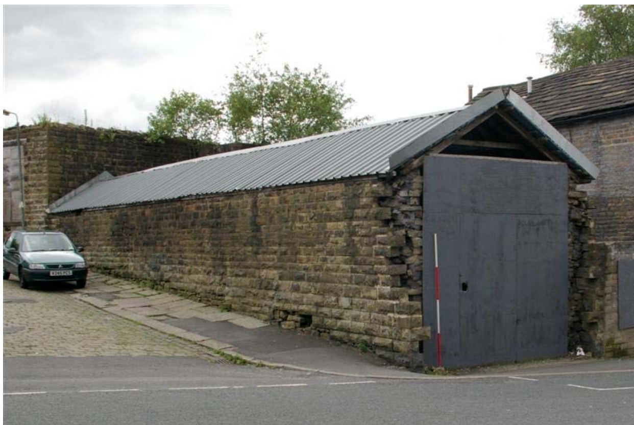
Plate 21: Boiler house, facing south
