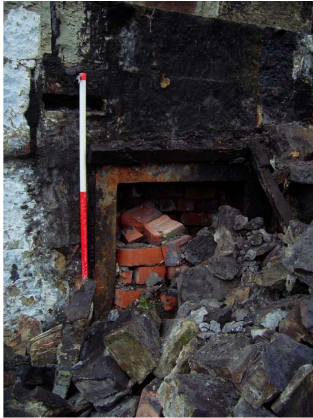
Plate 25: Bearing box within the south-eastern wall of the engine house, looking north
