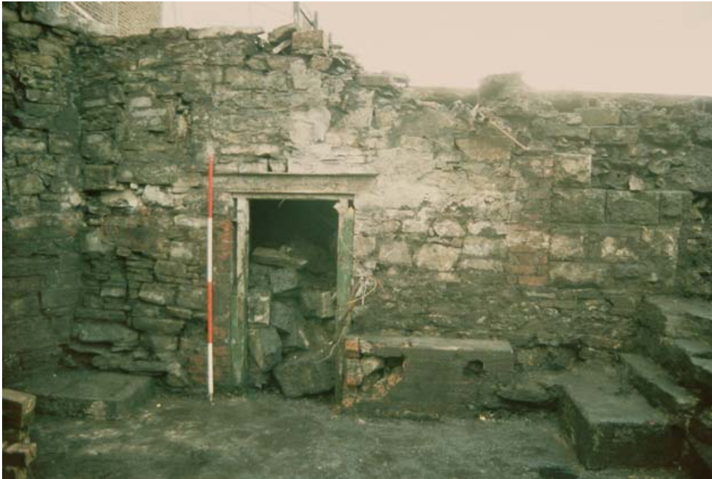
Plate 40: North-west-facing elevation of wall 50 within the economiser building, looking south-east
