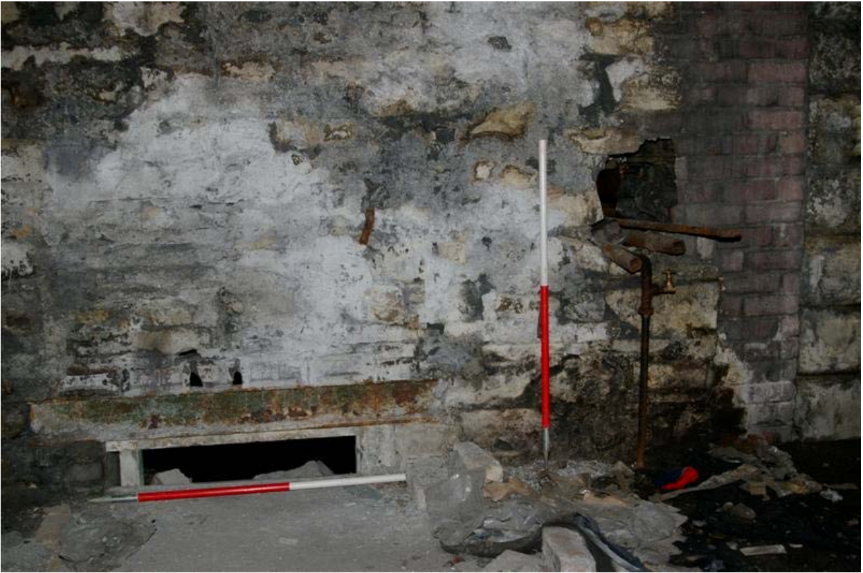
Plate 19: Apertures in the south wall of the economiser house
