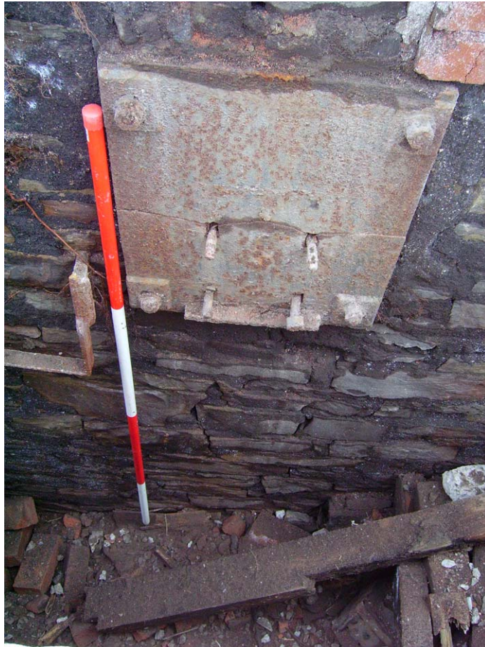
Plate 35: Metal plate 67 attached to wall 51 , looking south
