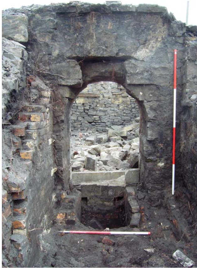
Plate 26: South-west-facing elevation of the interior of the chimney, looking north-east
