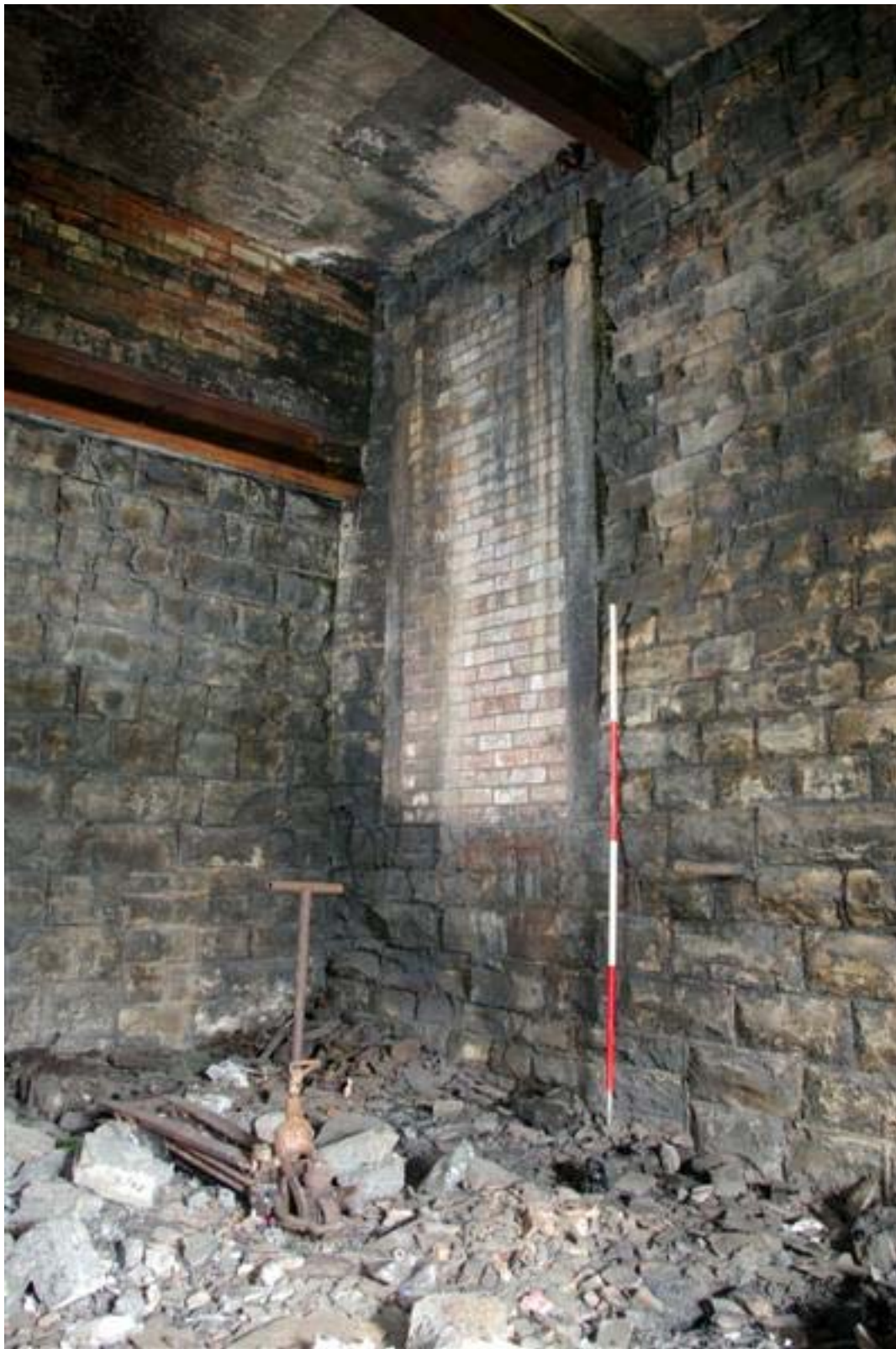
Plate 14: Blocked window the loading bay
