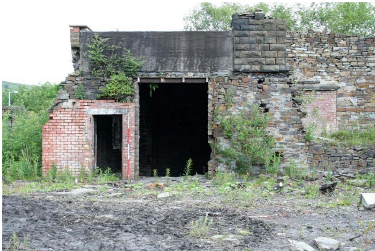
Plate 11: South elevation of the loading bay
