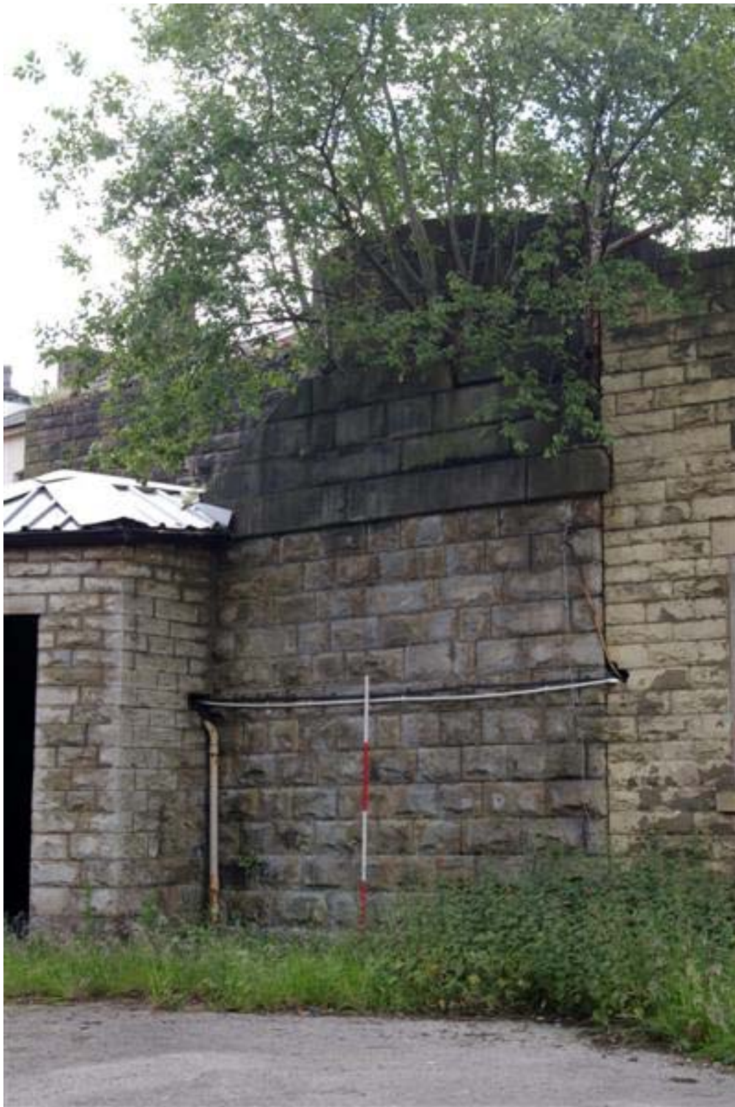
Plate 22: The chimney base
