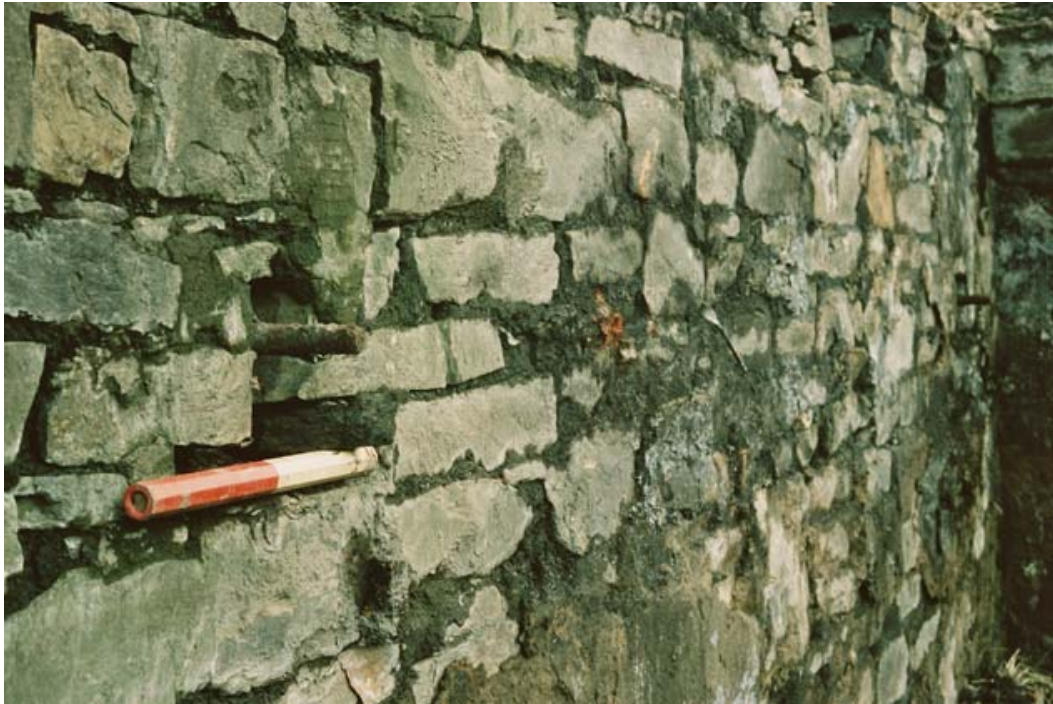
Plate 27: Metal fittings in eastern wall of weaving shed for supporting line shafting
