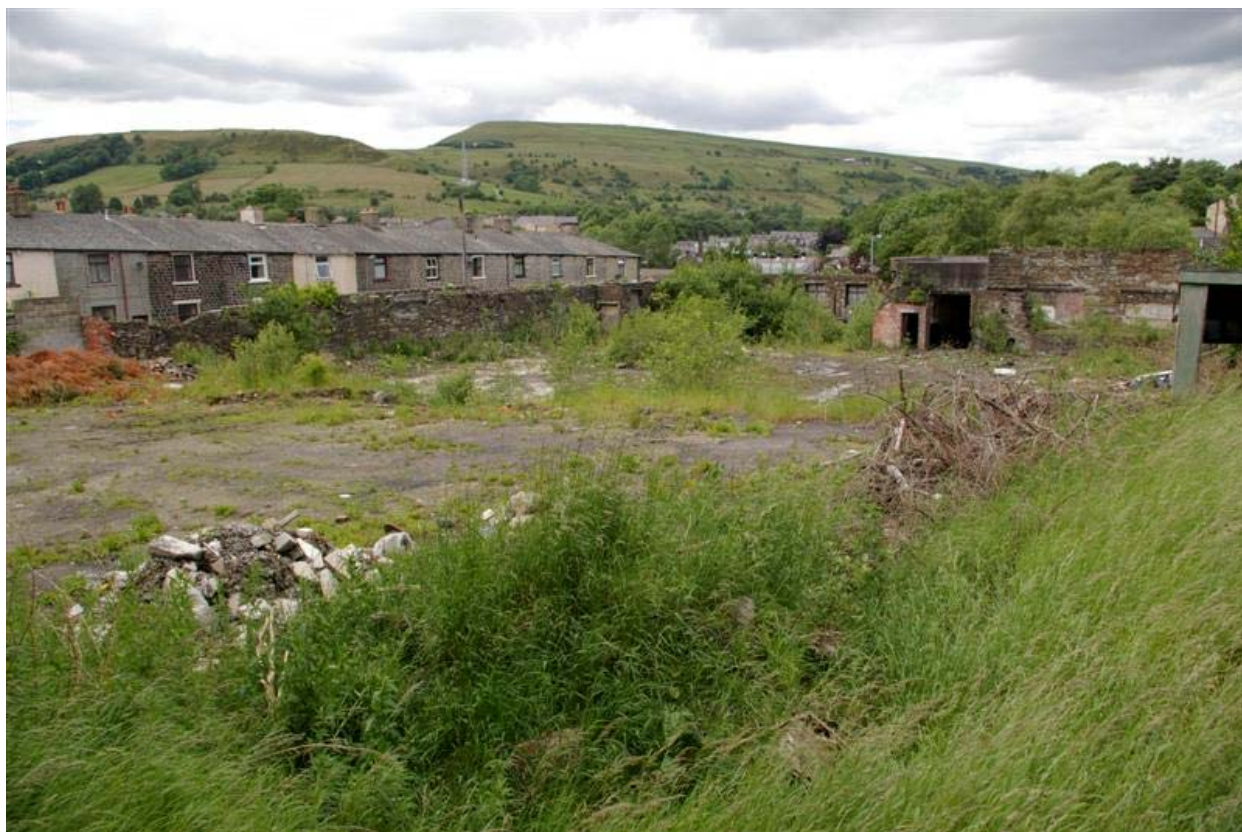
Plate 2: General view of the site facing north-west
