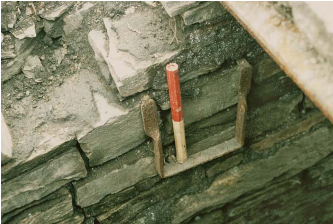
Plate 34: Rung 65 attached to wall 51, looking south
