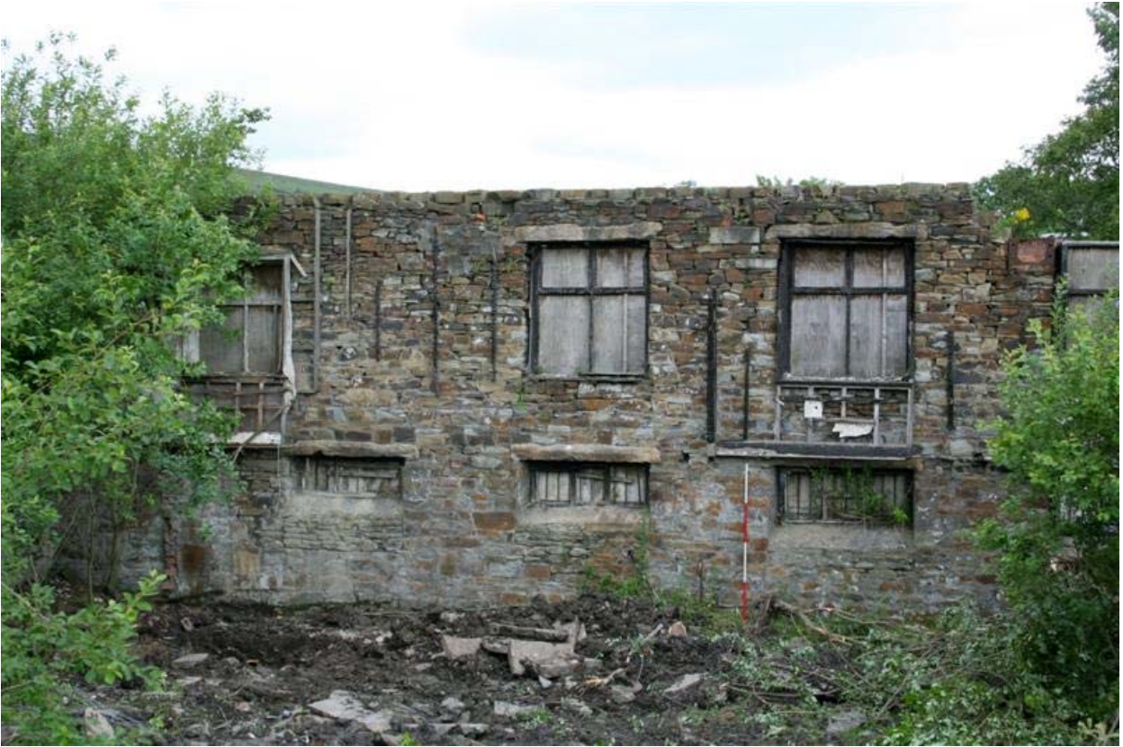
Plate 7: Internal view of the north wall of the spinning block
