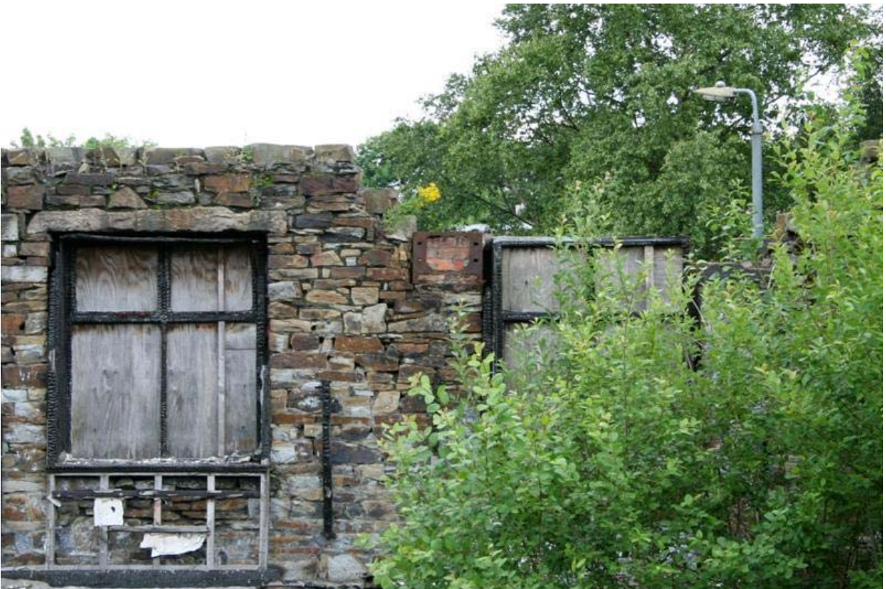
Plate 8: Bearing box (centre) in the internal elevation of the north wall of the spinning block
