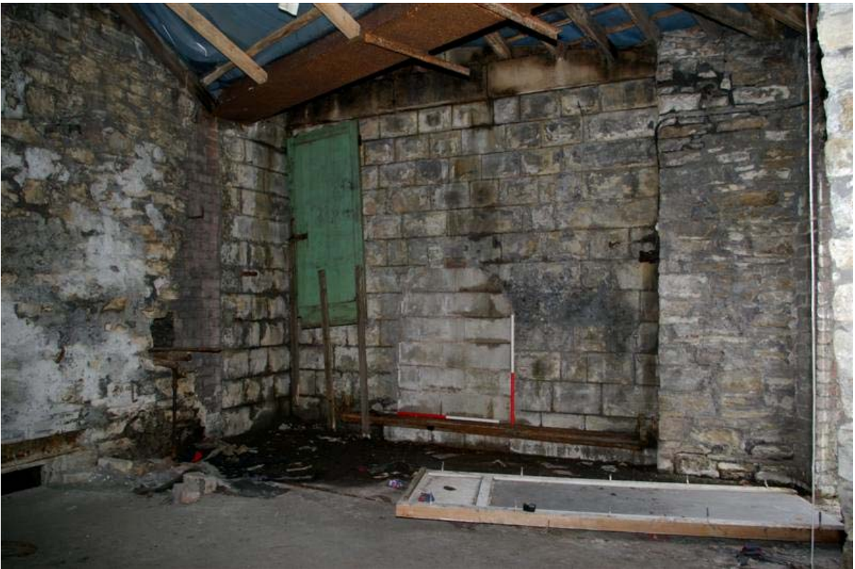
Plate 18: Arched aperture in the economiser house
