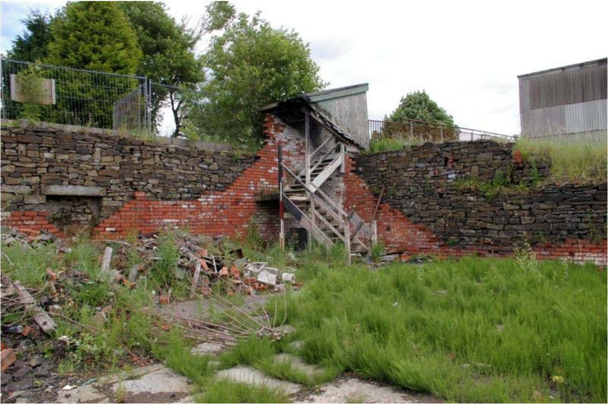
Plate 9: Internal view of the east and south walls of the weaving shed, together with stairs, showing brick lining of the stone walls
