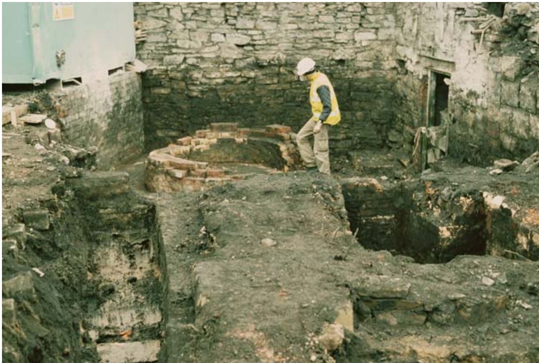
Plate 36: Working shot of the economiser house showing a doorway into the engine house, looking east
