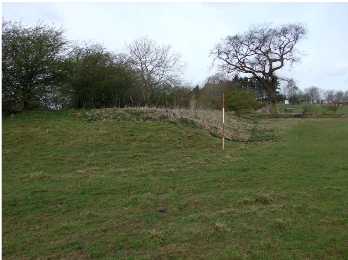
Plate 14: Site 11 , dismantled North Eden Railway/North Eastern Railway, Darlington Section, Eden Valley Branch
