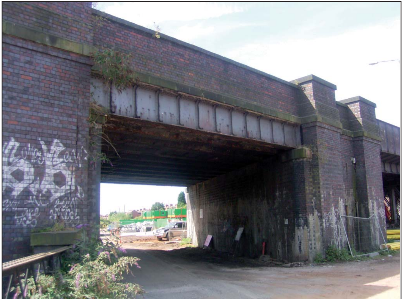
Plate 6 : Span 3 View to South-West
