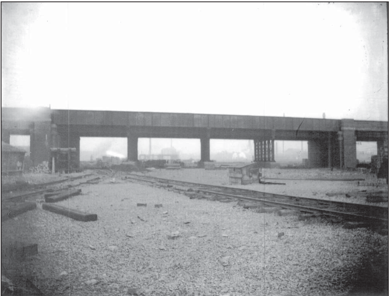
Plate 2 : Spans 4-7 View to North c.1897-1903 by S.W.A. Newton
