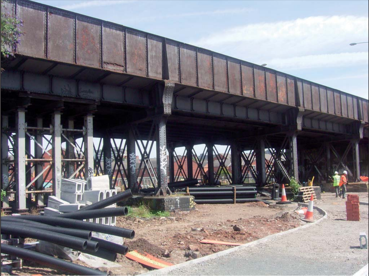
Plate 8 : Spans 4 to 7 View to North West
