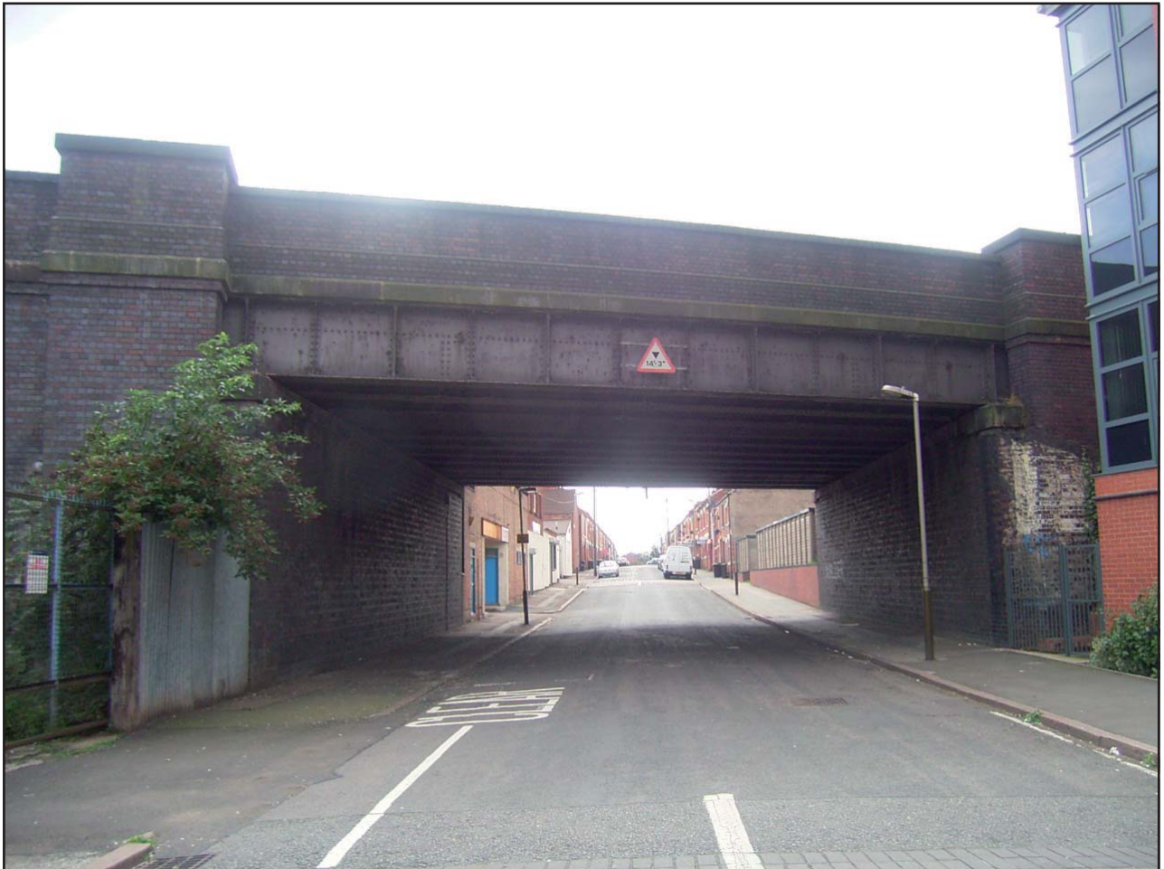
Plate 14 : Span 12 View to South
