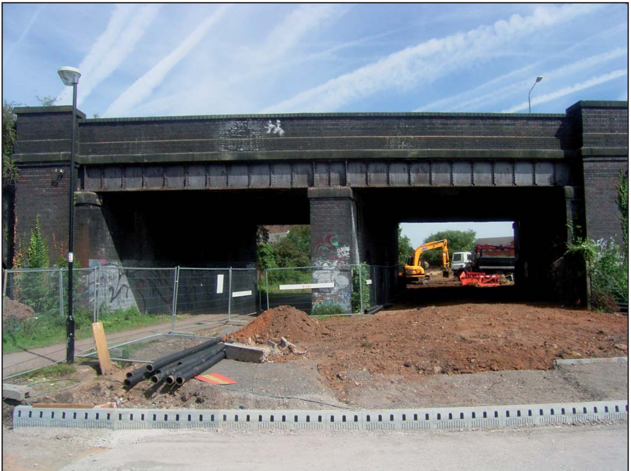
Plate 10 : Spans 8 & 9 View to North
