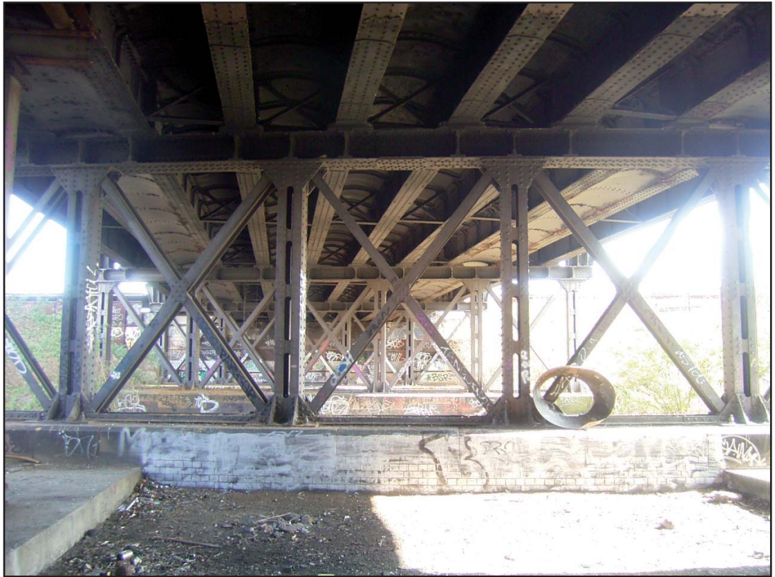
Plate 9 : Spans 4 to 7 Internal Structure
