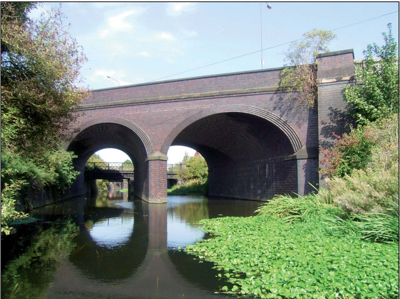
Plate 4 : Spans 1 & 2 View to North
