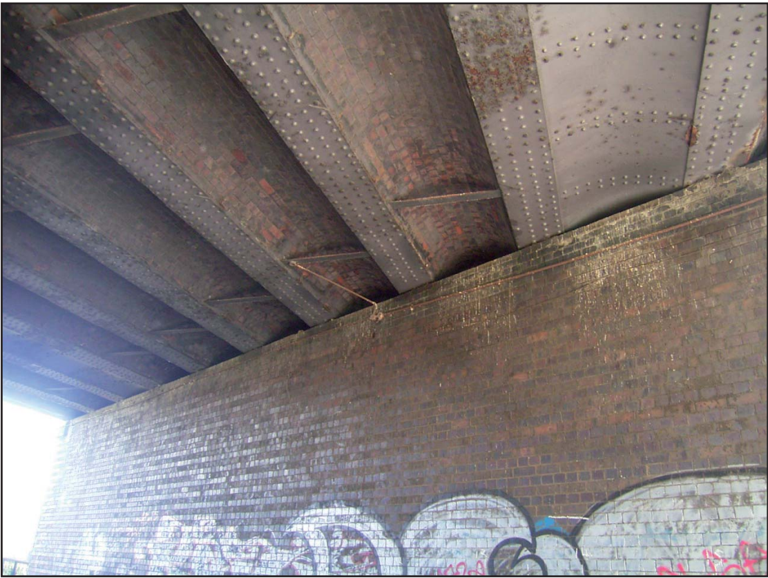
Plate 7 : Span 3 Showing Girders and Brick Jack Arches
