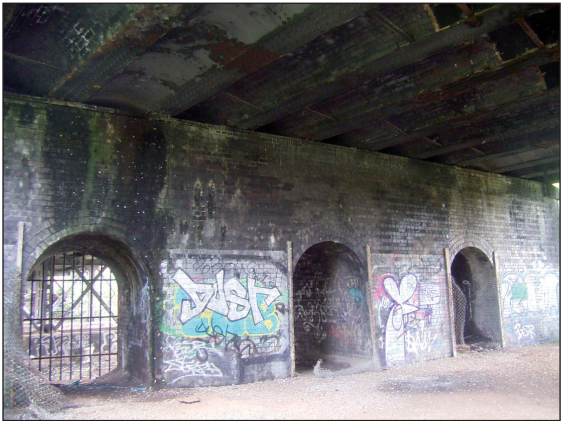
Plate 11 : Spans 8 & 9 Showing Safety Refuges
