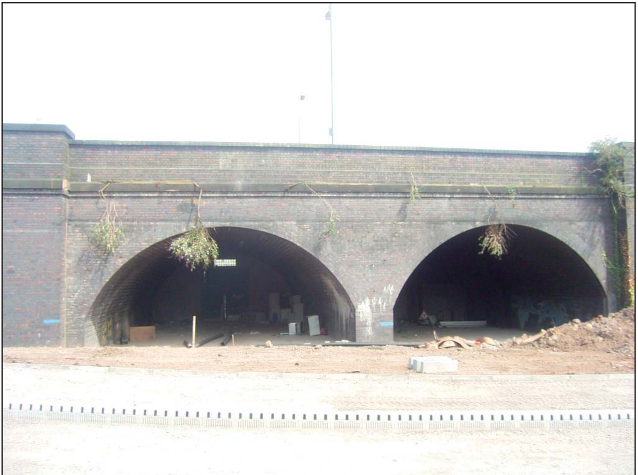
Plate 12 : Spans 10 & 11 View to North
