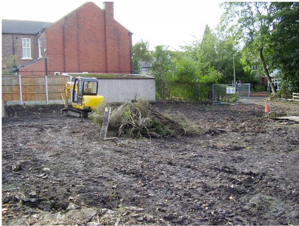
Plate 1: General south-facing view across the site
