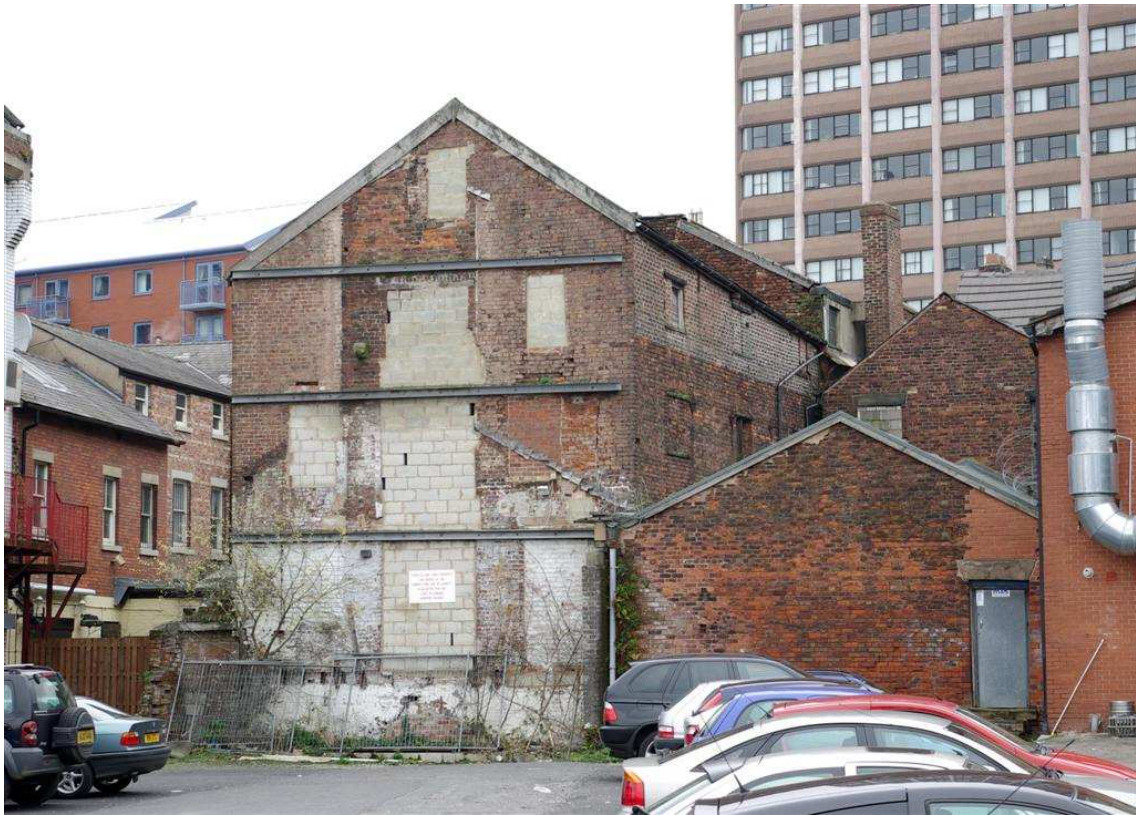
Plate 31: The rear of No. 131a Church Street
