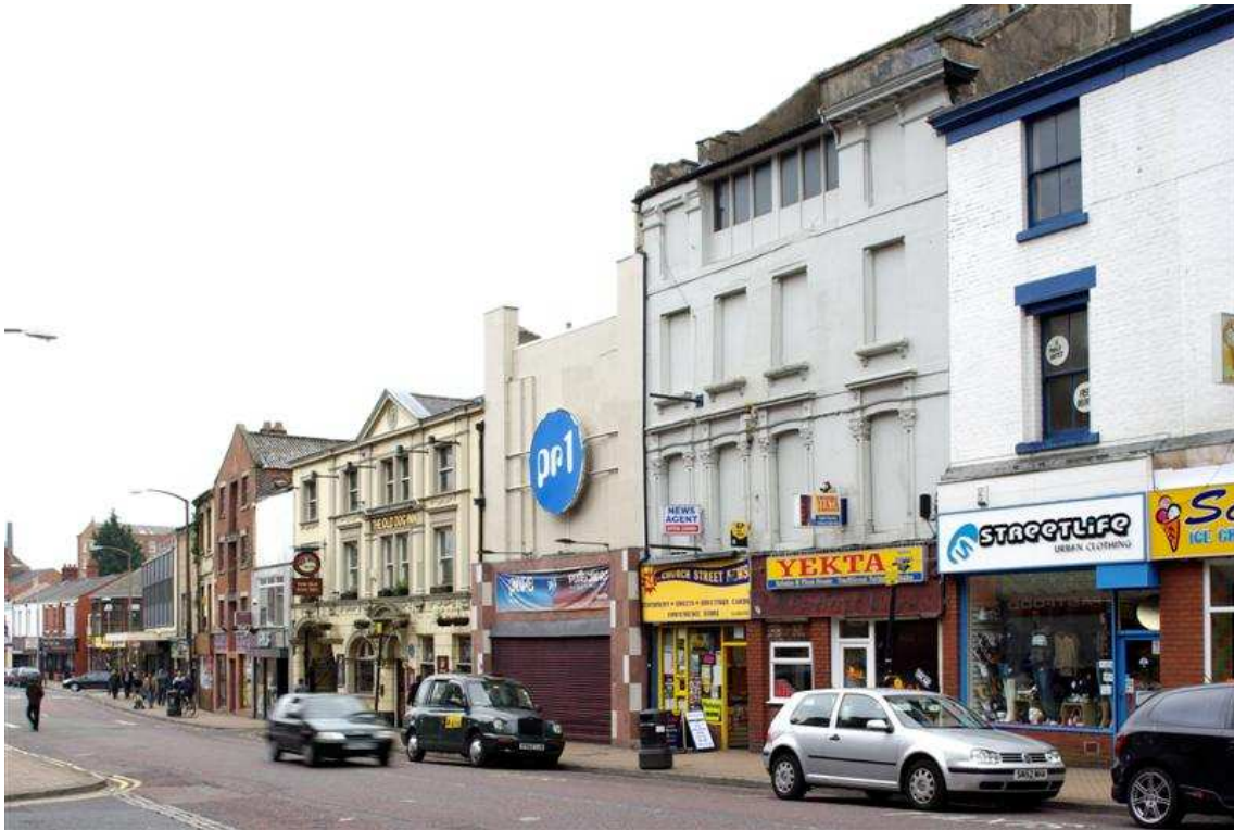
Plate 1: General view of 130-136 Church Street, facing east
