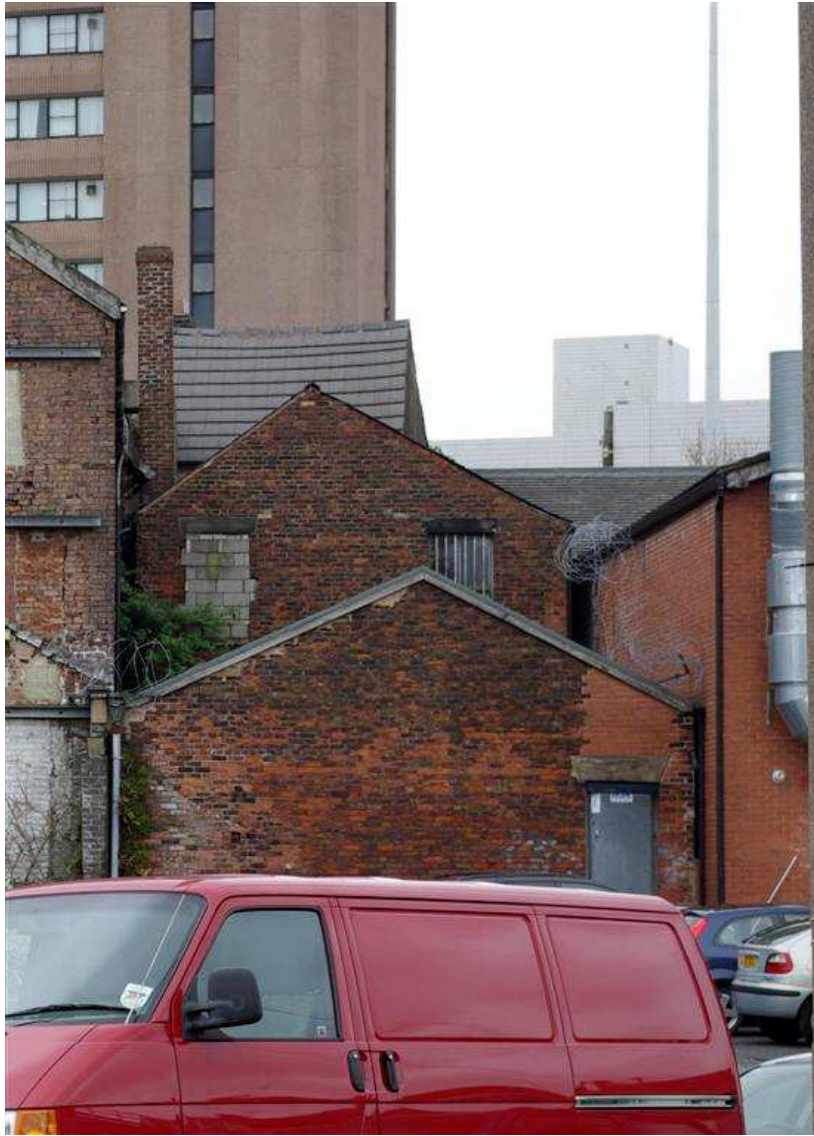
Plate 29: The rear of No. 131 Church Street
