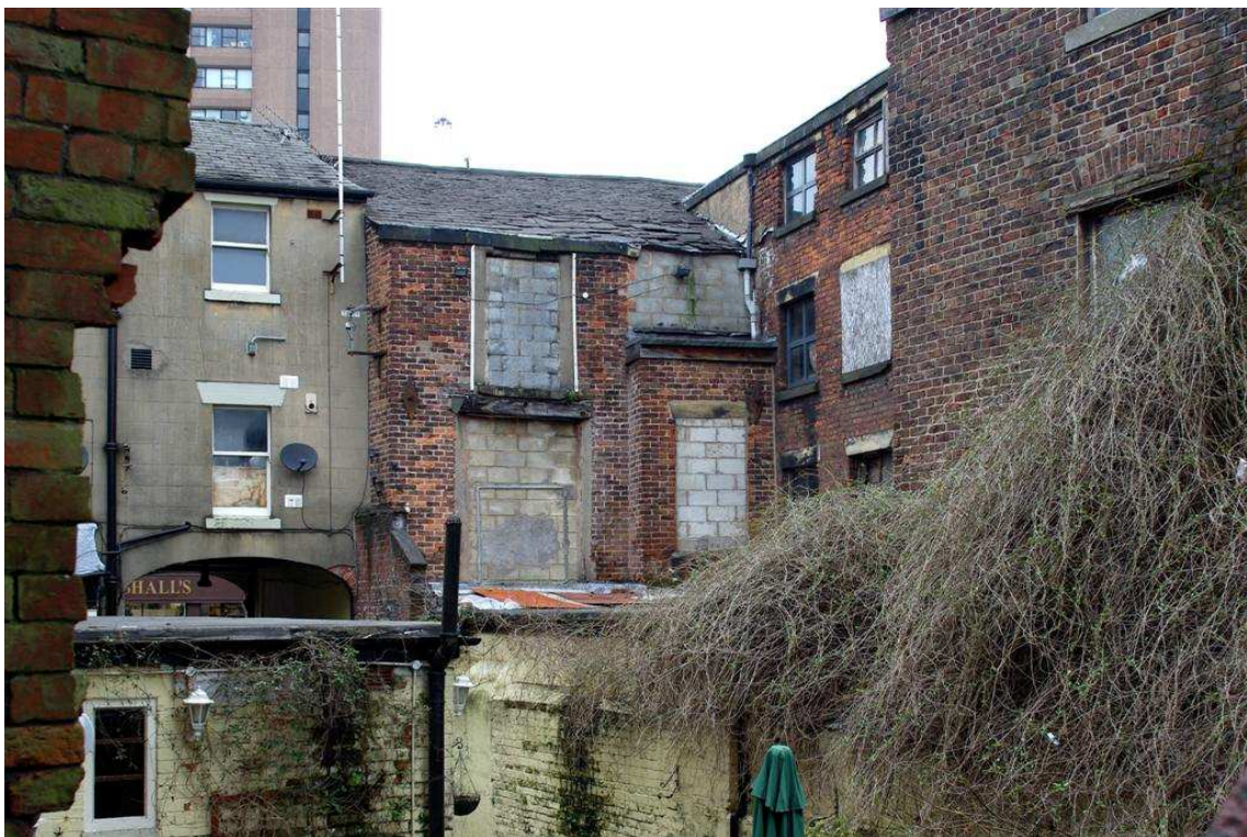
Plate 32: The rear of Nos. 131 and 132 Church Street
