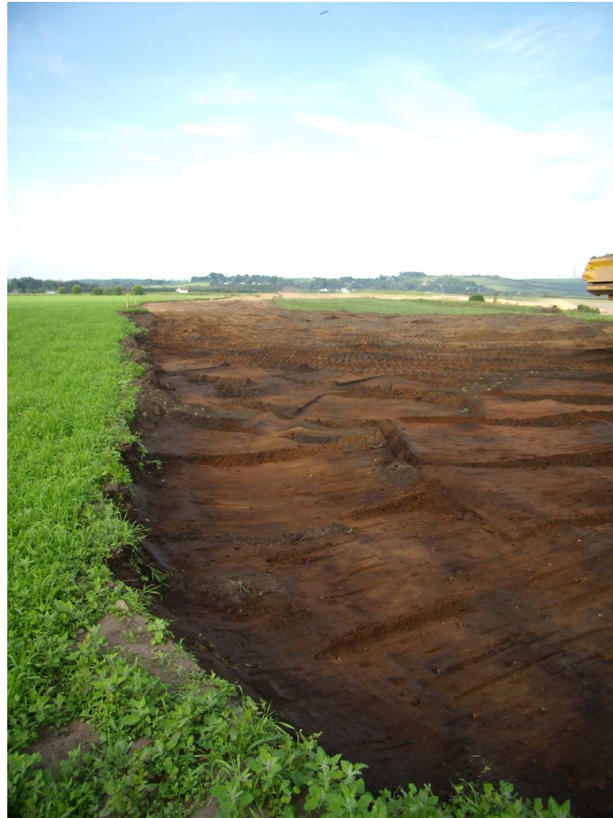
Plate 1: General view of topsoil strip, facing south-west
