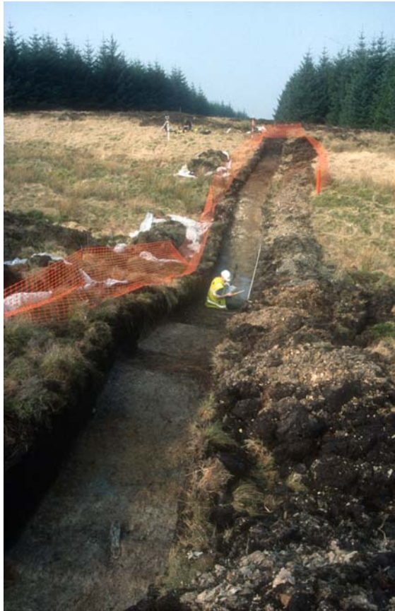
Plate 1: Working shot of trench, looking west.
