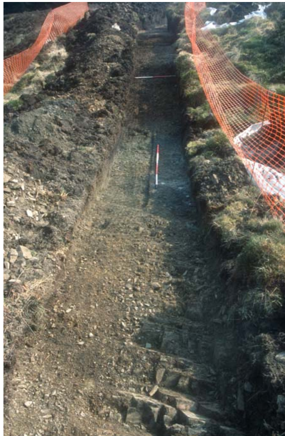
Plate 2: Centre of excavated trench, looking east.
