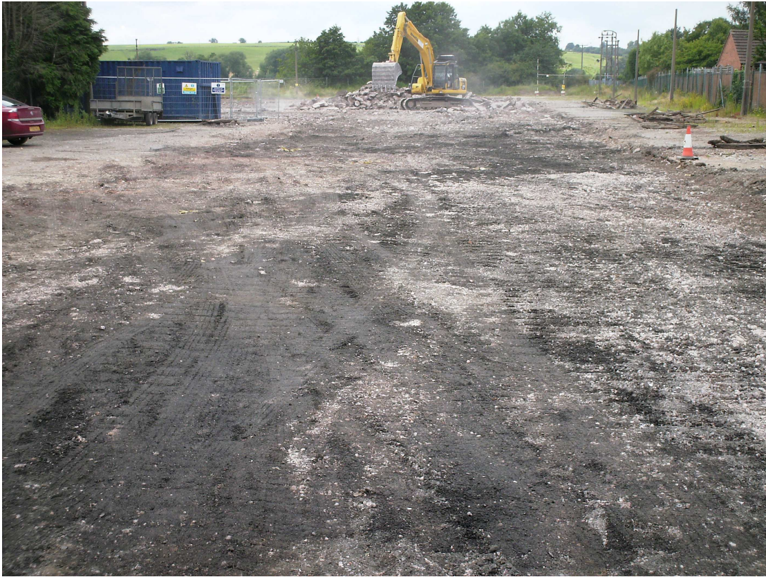
Plate 1: Concrete surface removed from western plot
