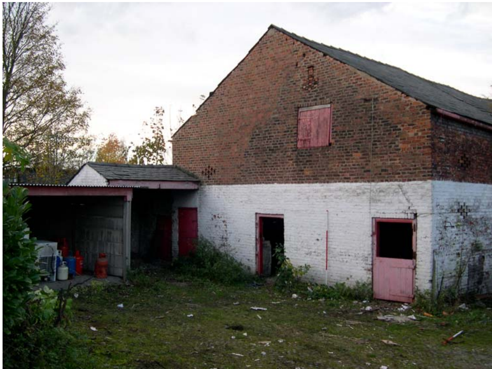
Plate 15: The south elevation of the barn ( Building Two )
