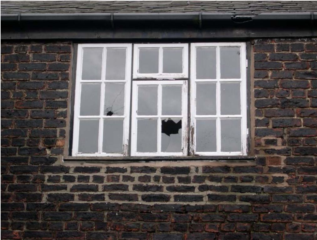
Plate 5: Detail of the rebuild around one of the inserted ventilator casements
