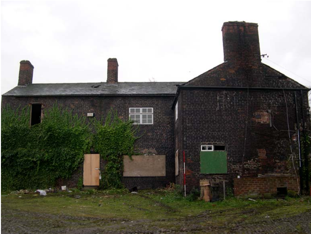
Plate 1: The rear (south) elevation of the farmhouse, with the rear wing to the right
