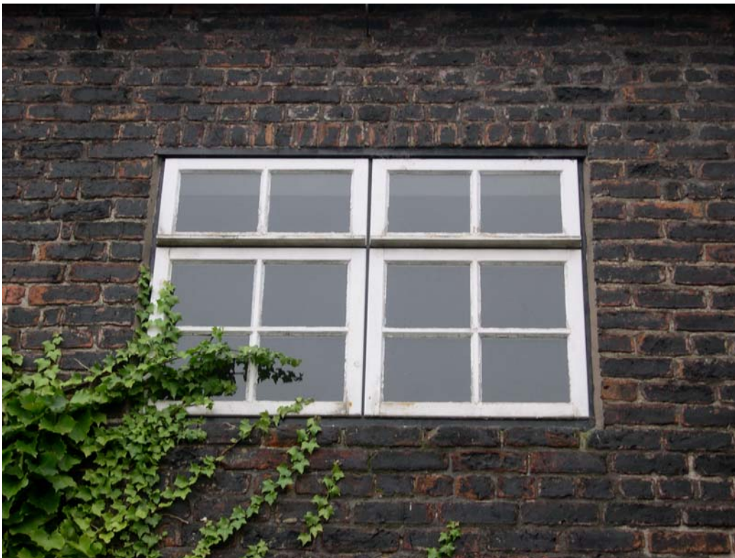
Plate 6: Detail of the original brick rubbers, overlying one of the inserted modern casements
