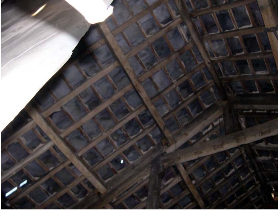
Plate 18: The queen-post truss at the south end of the barn, featuring a king-tie and collar of reused timber
