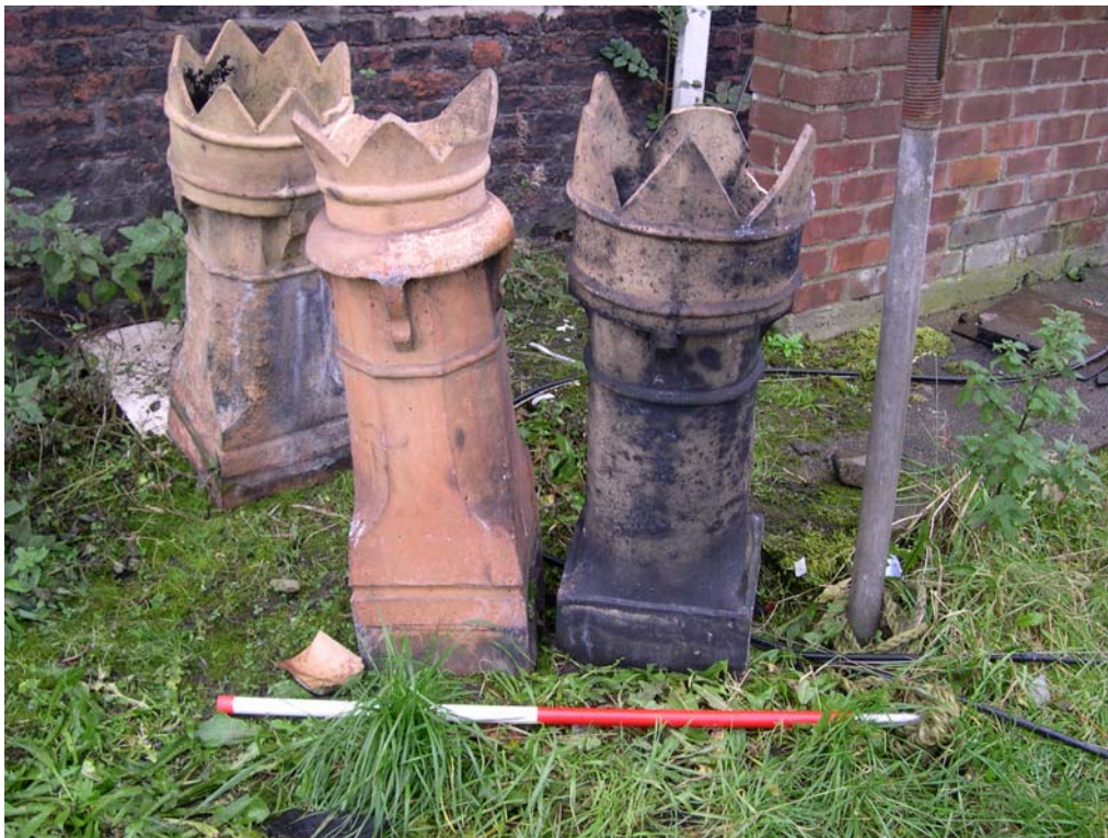
Plate 4: The bishop style pots used on all of the chimney stacks on the farmhouse.
