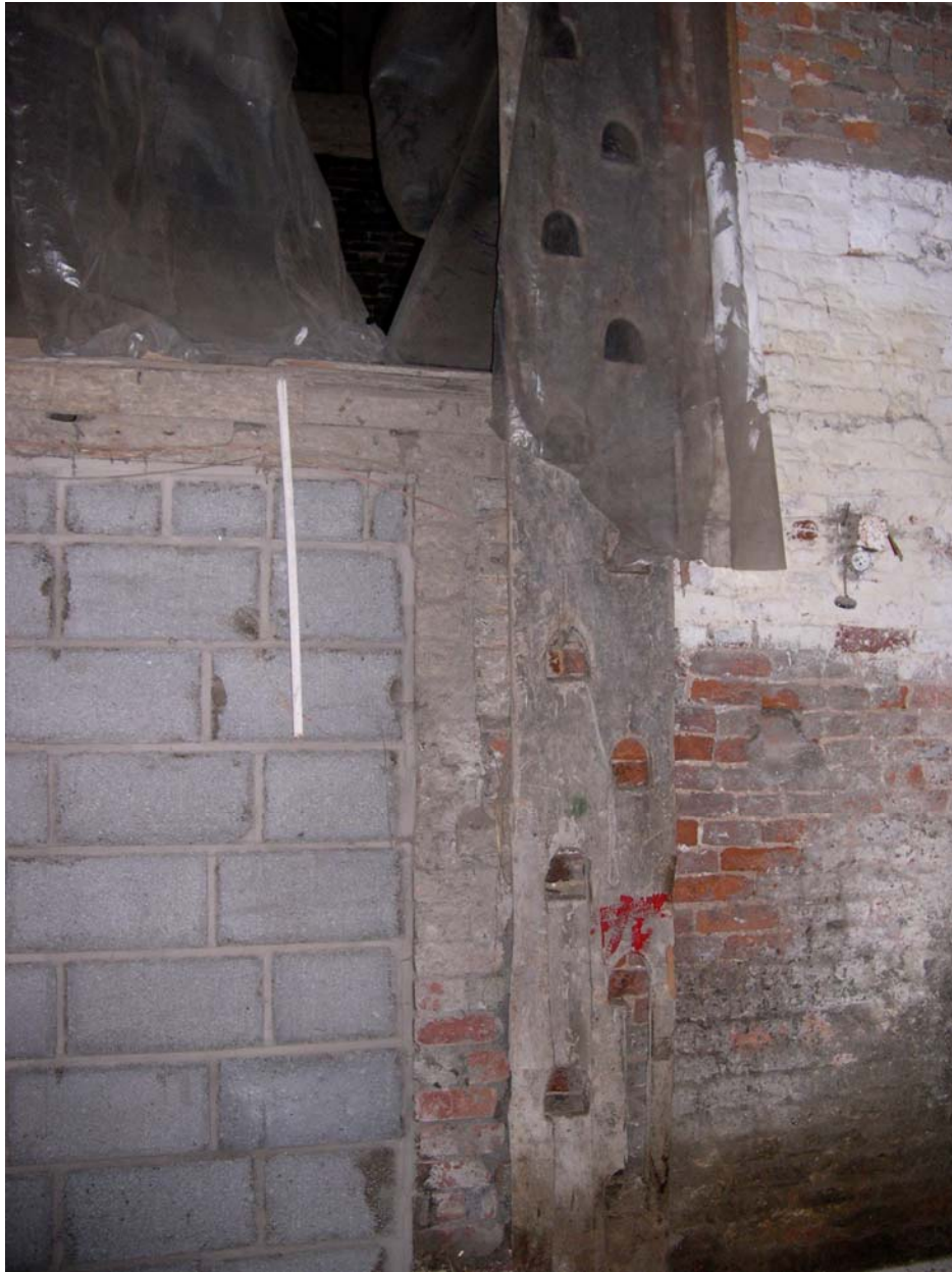
Plate 19: Detail of the loft-ladder and the blocked access doorway to the shippens
