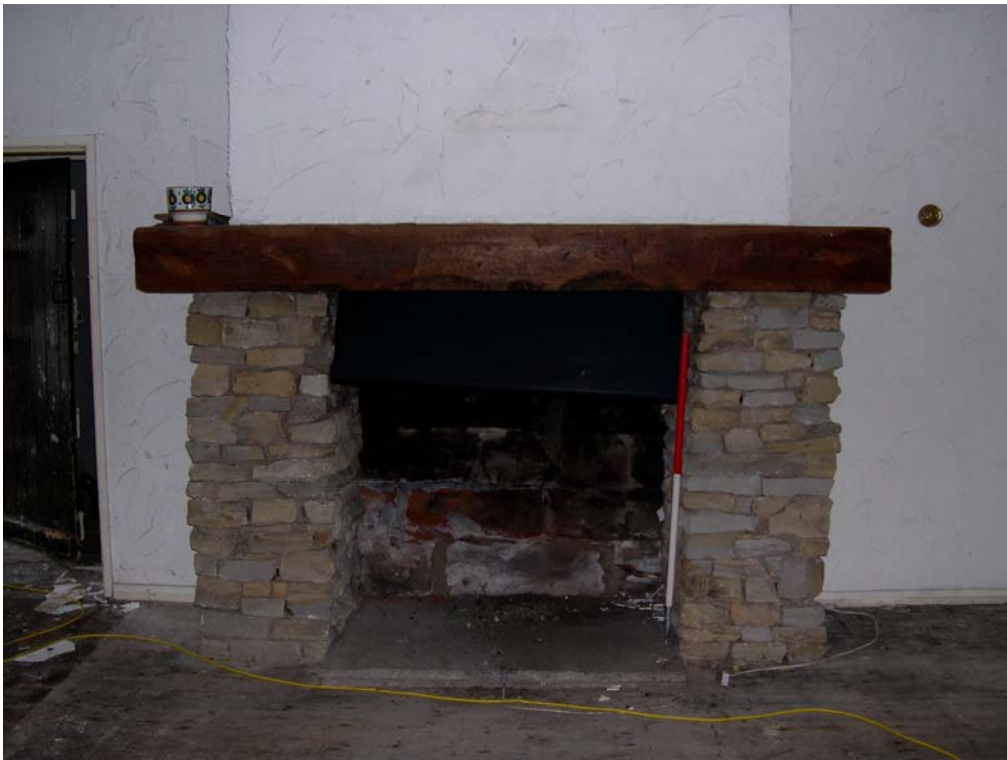
Plate 9: Detail of the modern stone fireplace in room 2
