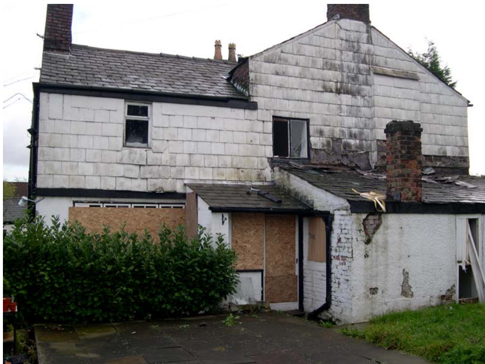
Plate 2: The west elevation of the farmhouse, including the slate-hung walls and the extension.
