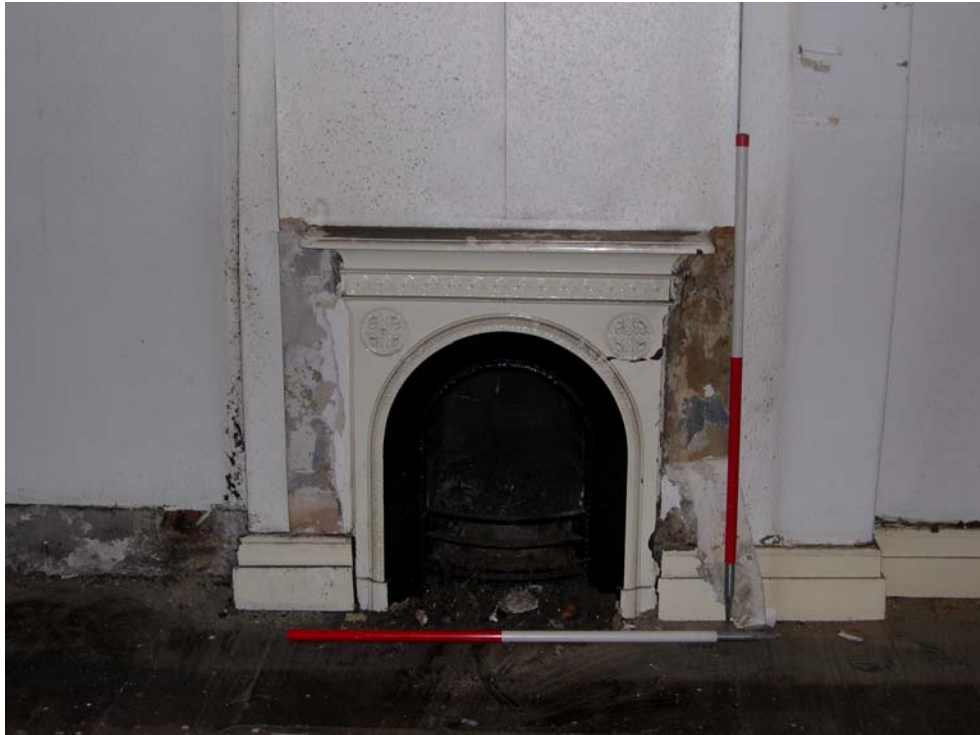
Plate 12: Detail of the fireplace in room 11
