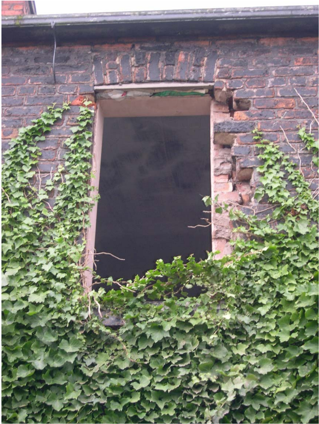
Plate 7: Detail of the segmental voussoir overlying one of the original window apertures
