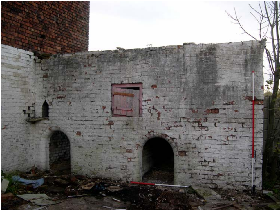
Plate 16: The hoghouse on the north-east of the barn
