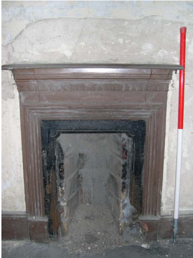
Plate 11: Detail of the fireplace in room 10
