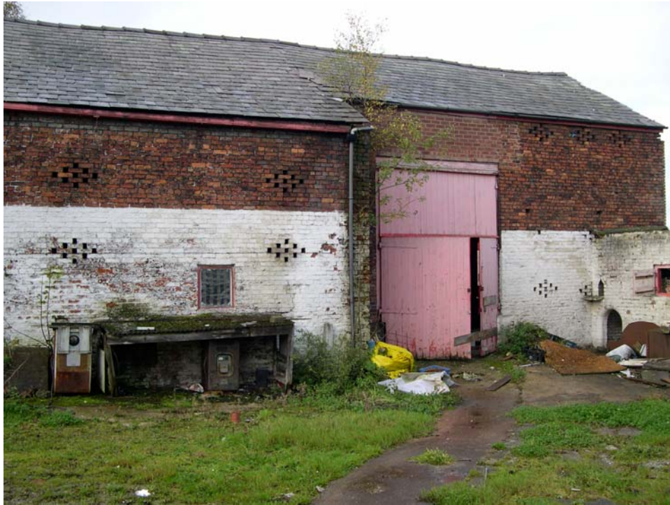
Plate 14: The east elevation of the barn ( Building Two )
