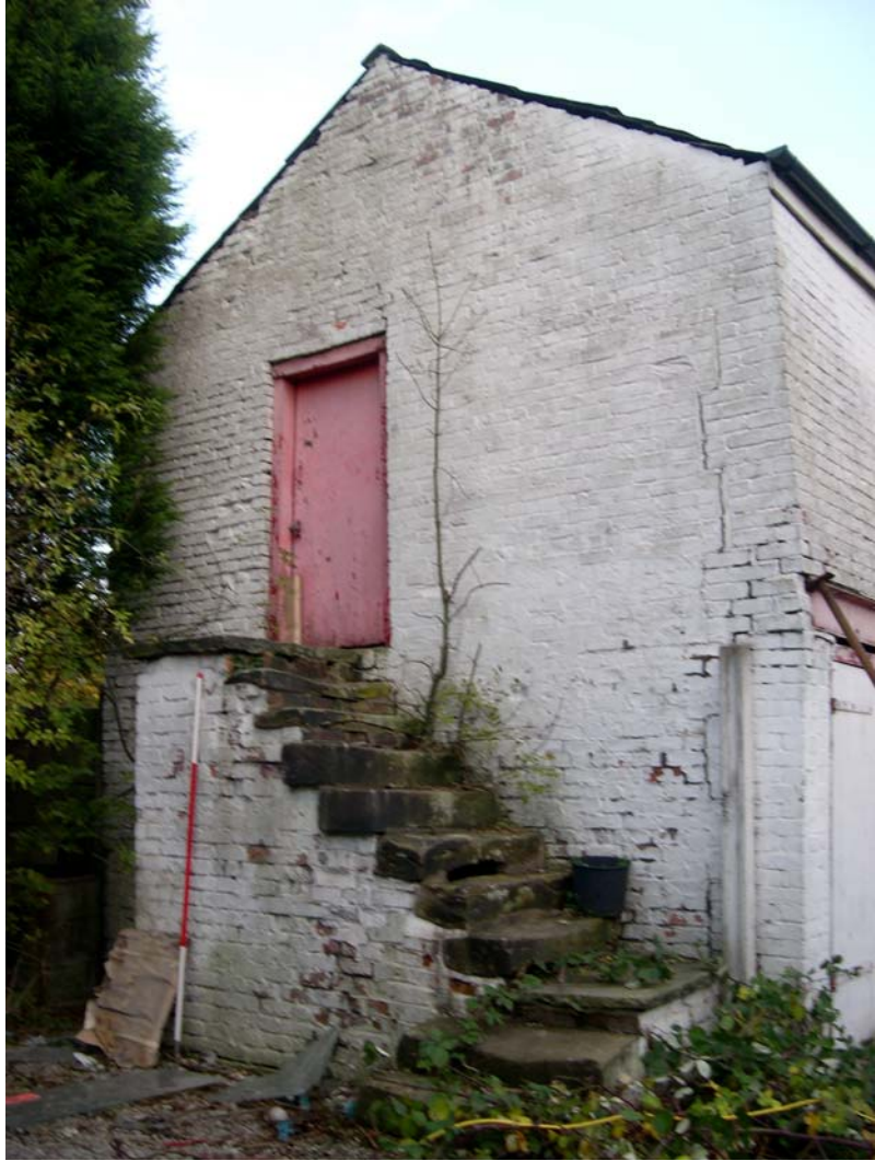
Plate 22: Detail of the staircase on the west elevation of Building Three
