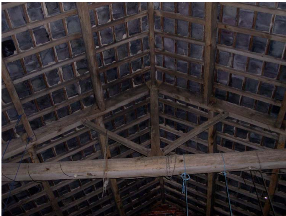
Plate 17: The king-post truss at the north extent of the barn
