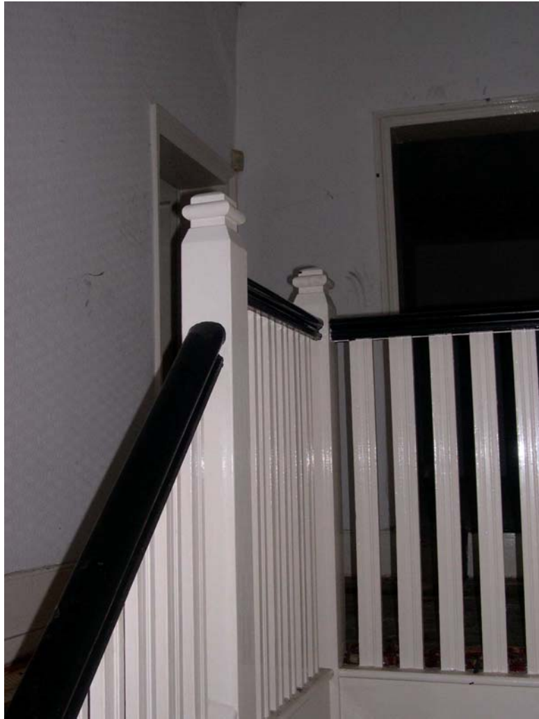
Plate 13: Detail of the balustrade on the staircase at the west end of the farmhouse
