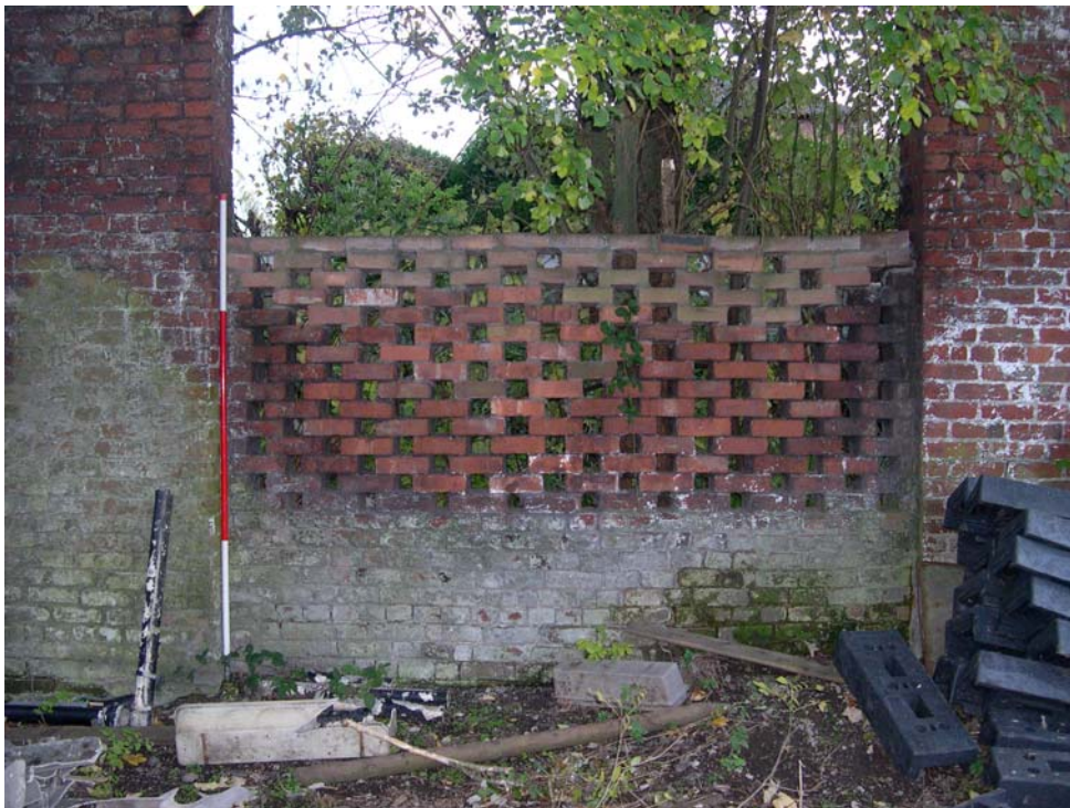
Plate 24: Detail of the ventilator pattern on the south elevation of the Dutch barn
