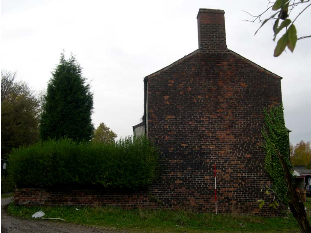
Plate 3: The east elevation of the house, illustrating the rebuild and oversailing of the gable chimney stack
