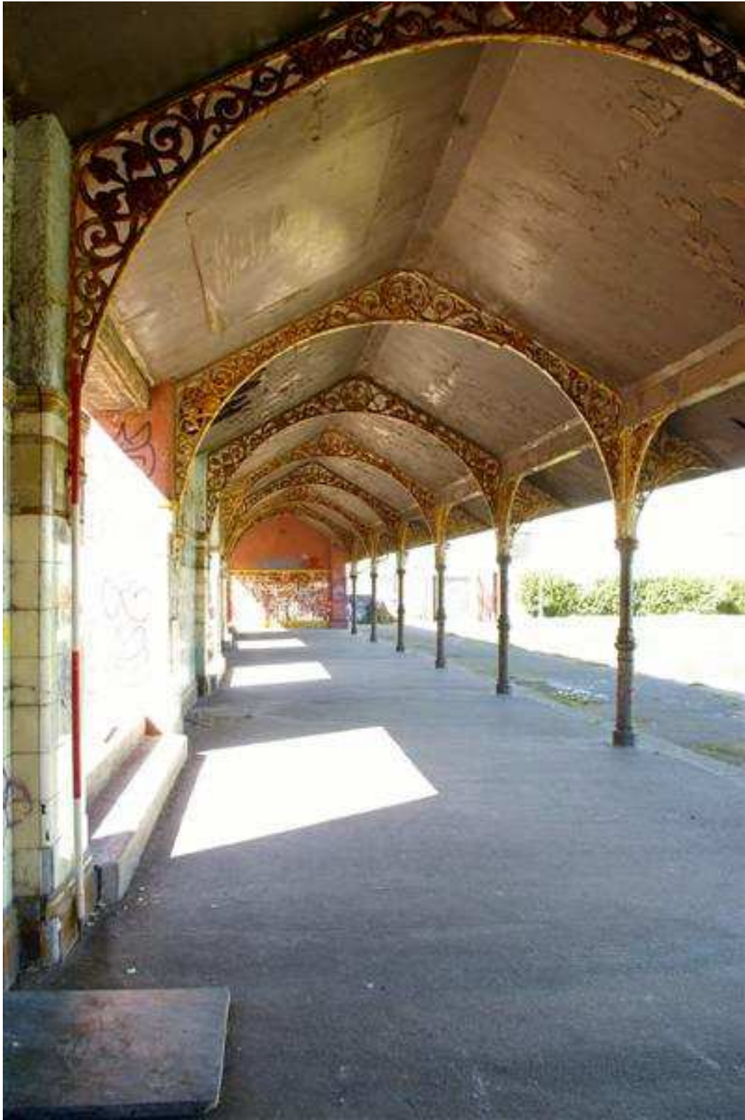
Plate 12: Interior of covered arcade
