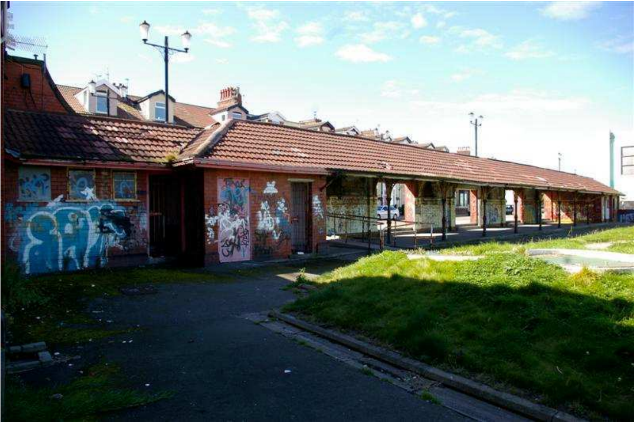
Plate 5: Covered arcade on the west of the building
