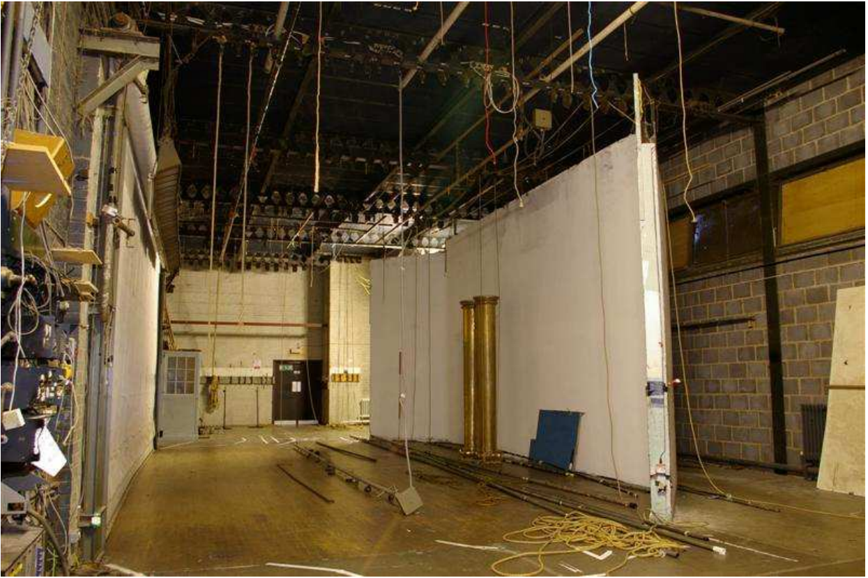
Plate 18: General view of the backstage area
