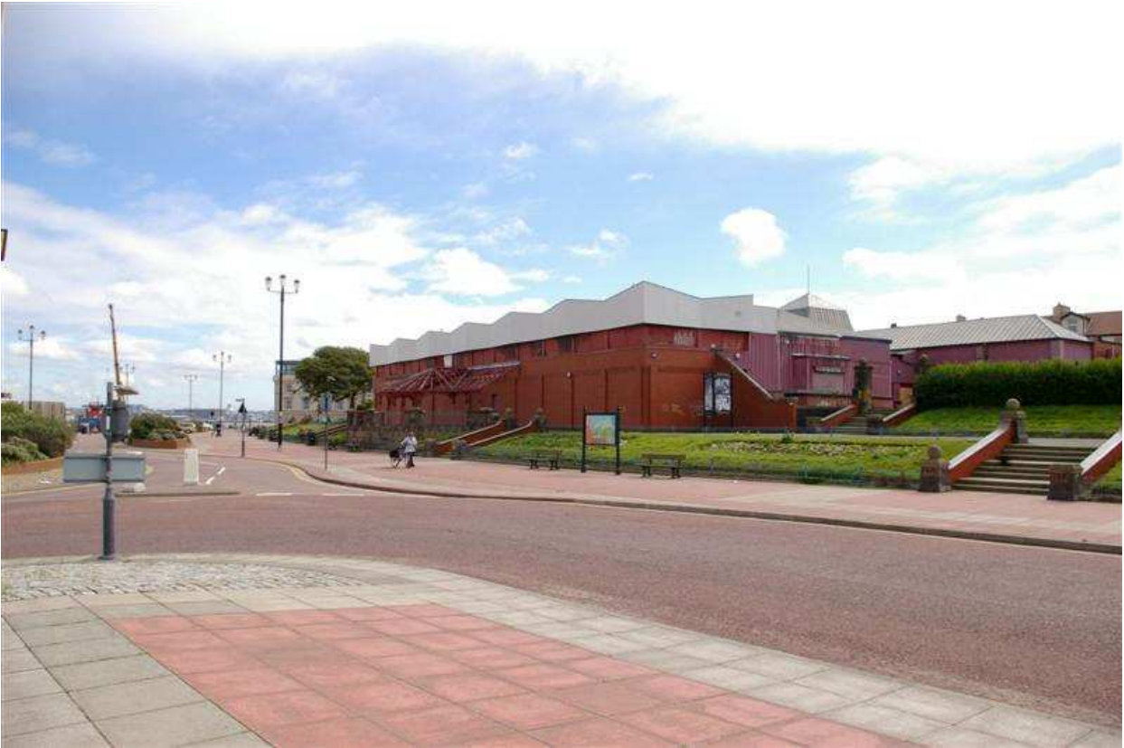
Plate 1: General view of the front of the Floral Pavilion
