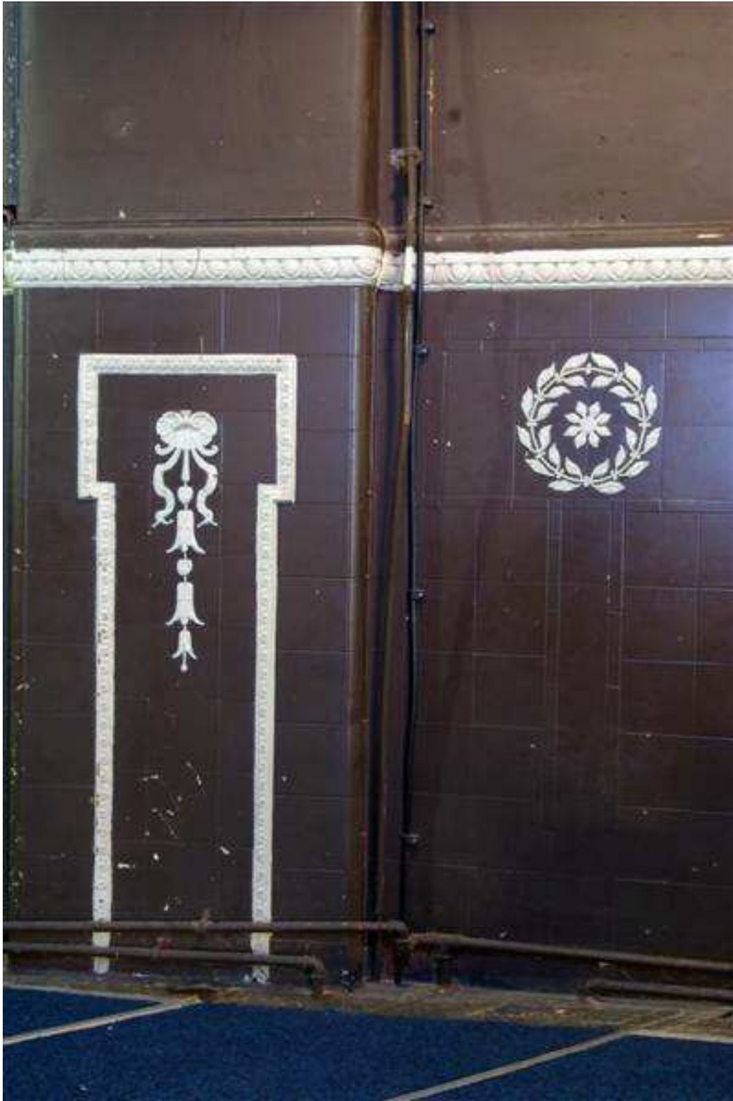
Plate 15: Decorative tiles at the rear of the auditorium
