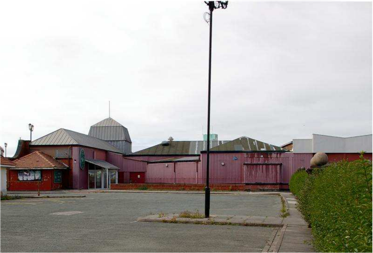
Plate 3: View of the east-facing elevation
