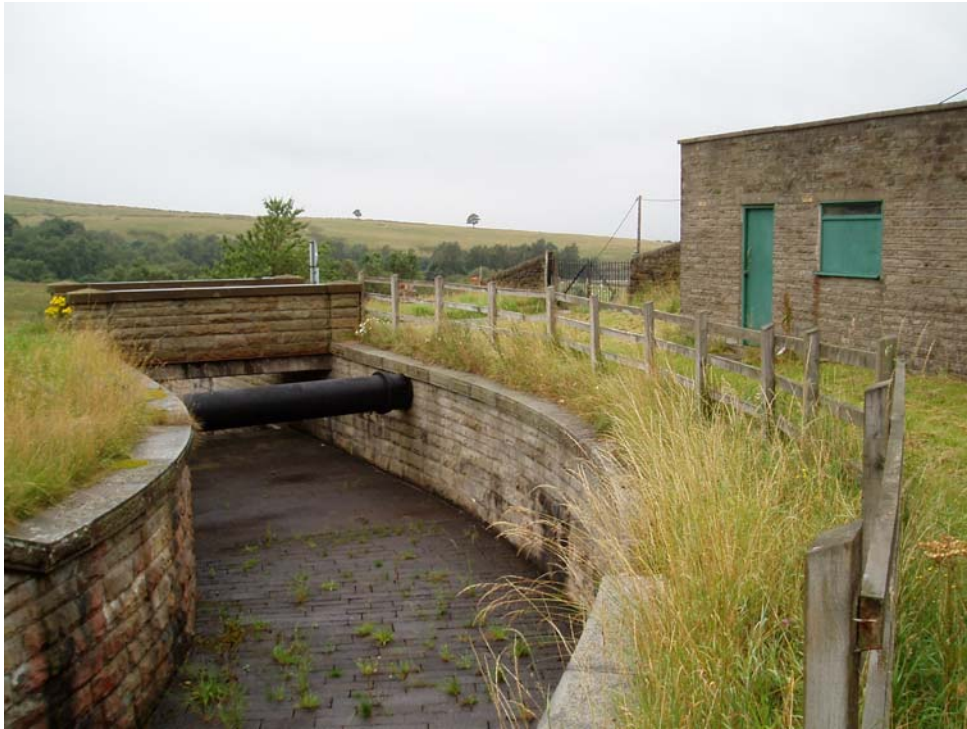
Plate 3: The fisherman's hut in relation to the overflow system of the dam for Bollinhurst reservoir
