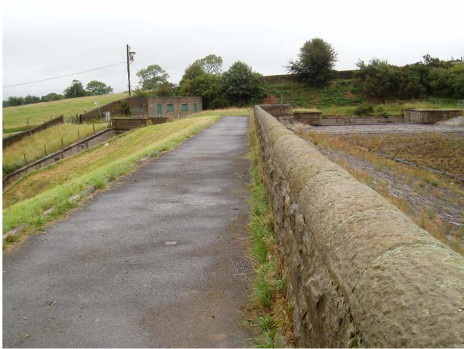
Plate 5: North-facing view of the fisherman's hut from behind the parapet wall of the dam
