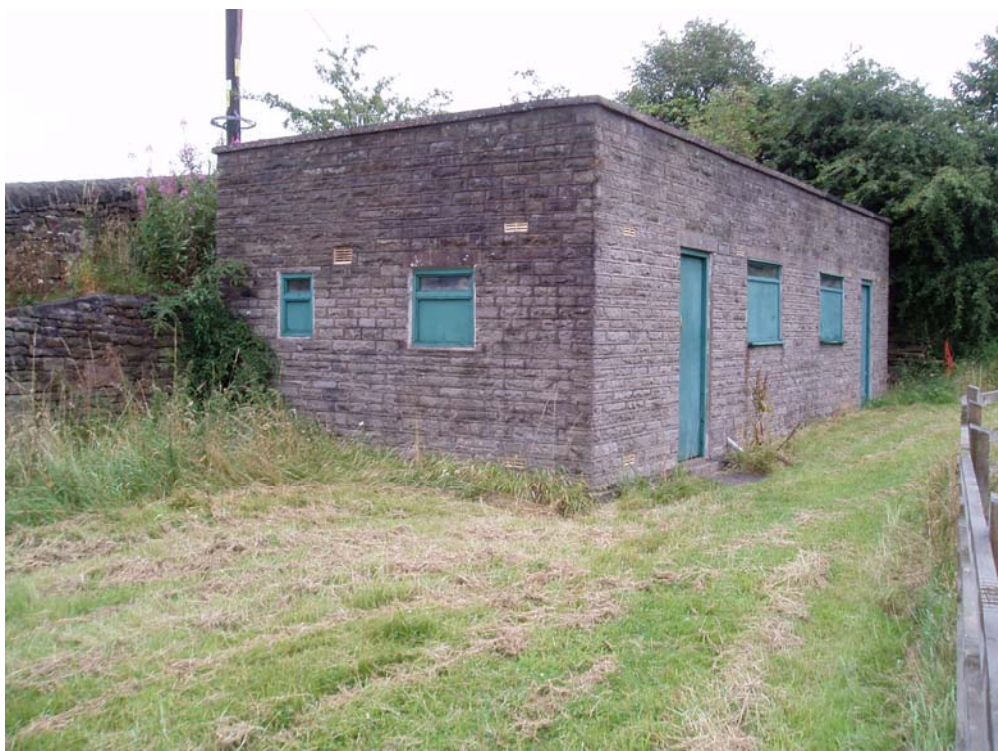
Plate 2: The west elevation of the fisherman's hut
