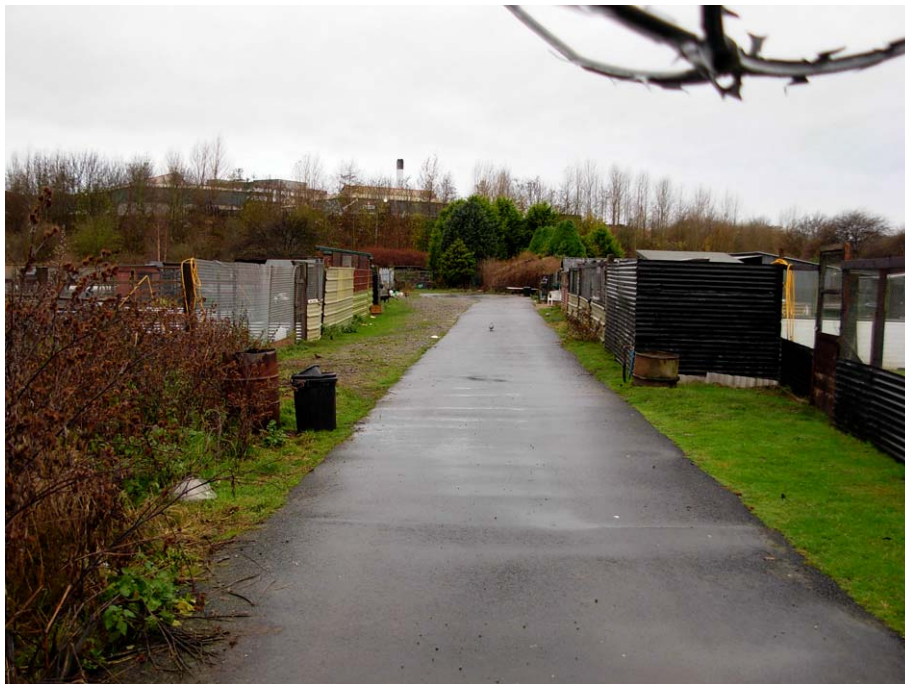
Plate 2: The route of the pipeline through the allotment gardens, viewed toward the west
