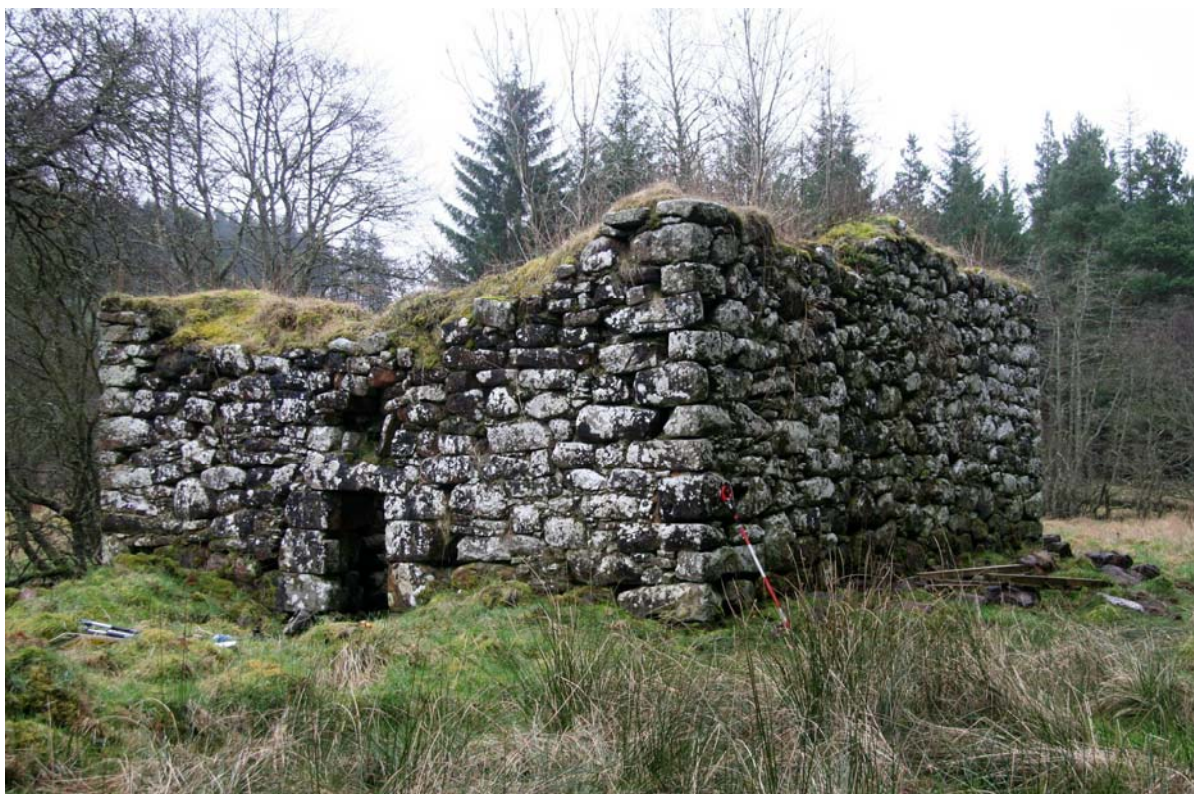
Plate 1: General view of Bog Head bastle looking south-east
