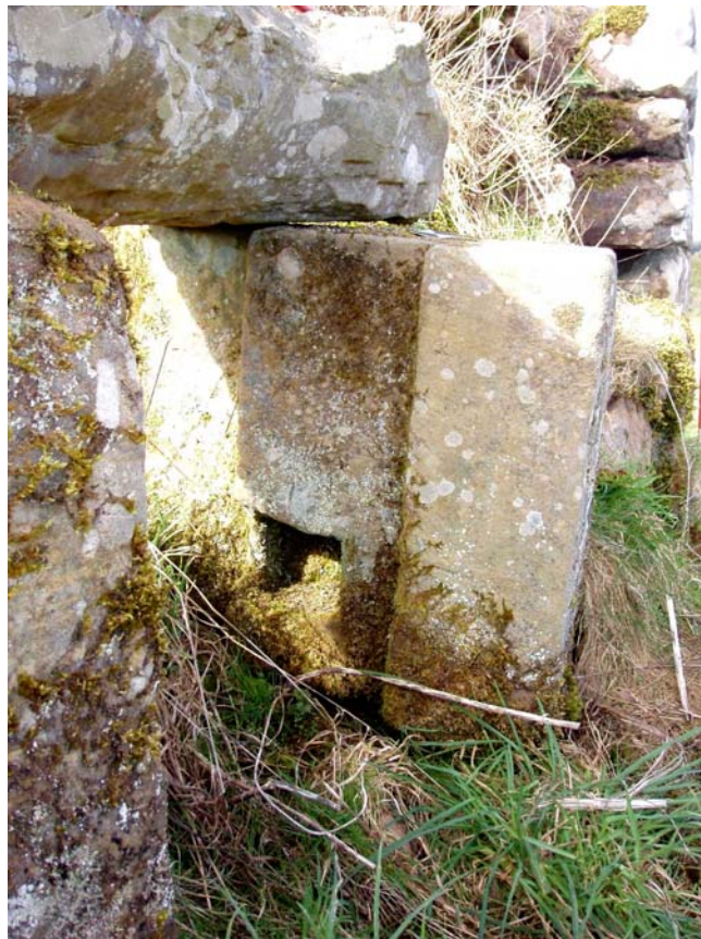
Plate 6: Entrance to Shilla bastle showing the tunnel for the drawbar
