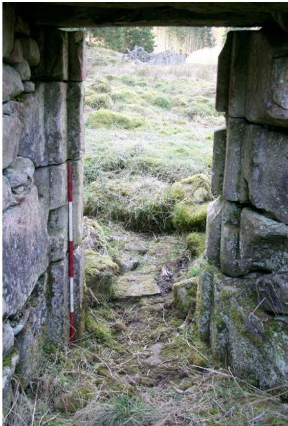
Plate 5: Principal entrance of Bog Head bastle showing the checks for two doors and the tunnels for drawbars
