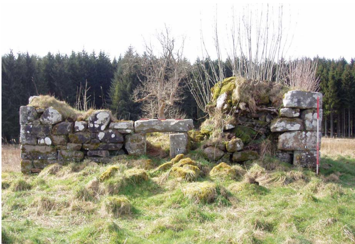
Plate 2: The principal façade of Shilla Bastle looking north-east
