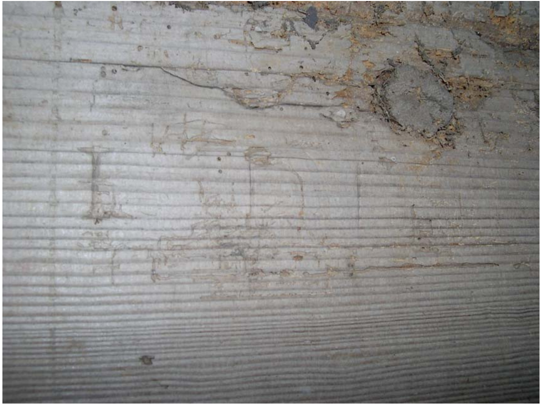
Plate 9: Carved 'I', possibly part of date, in the tie beam of the northern truss
