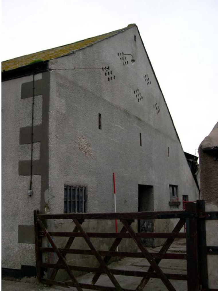
Plate 7: The north external elevation of the barn
