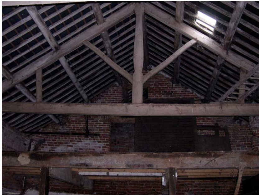
Plate 8: The southern truss within the barn
