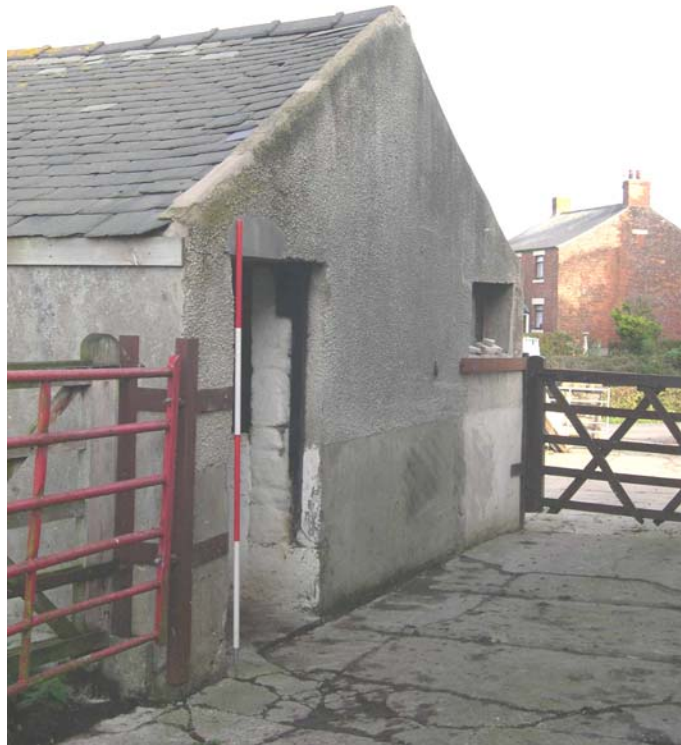
Plate 17: The south elevation of the north/south axis of the cow sheds
