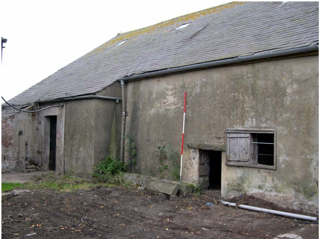
Plate 6: The north end of the west external elevation of the barn
