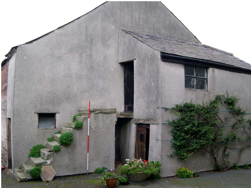
Plate 4: The south external elevation of the barn
