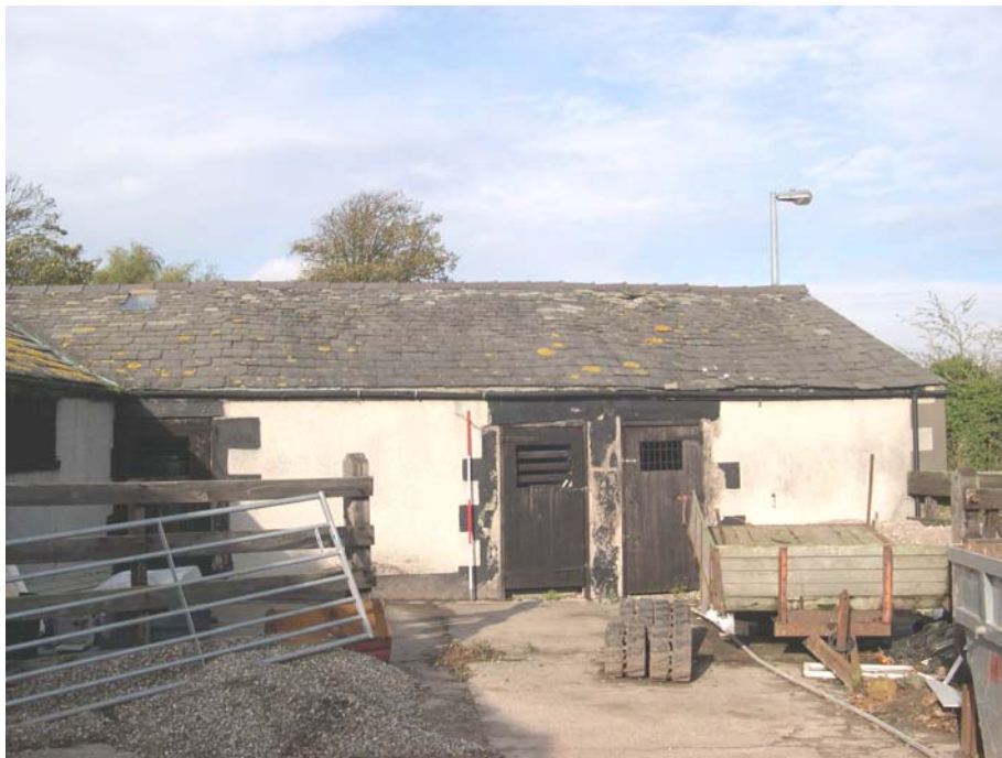
Plate 18: The south elevation of the east/west axis of the cow sheds
