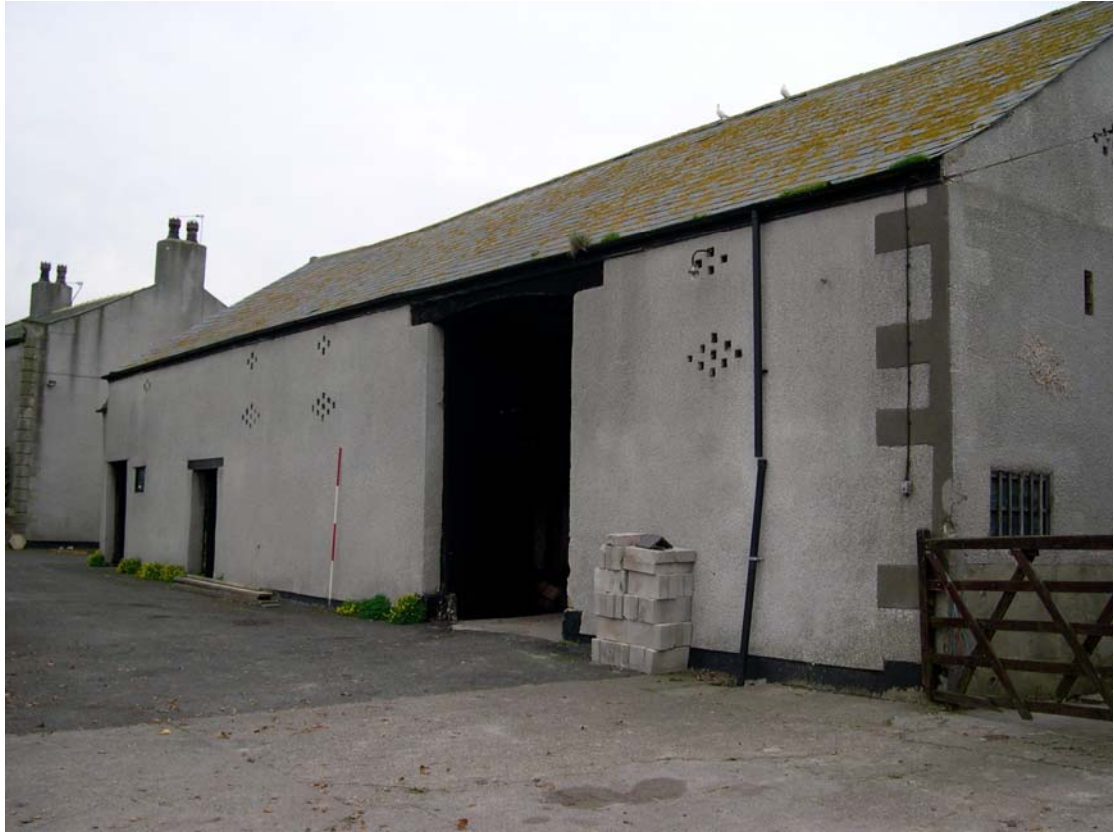
Plate 3: The east external elevation of the barn
