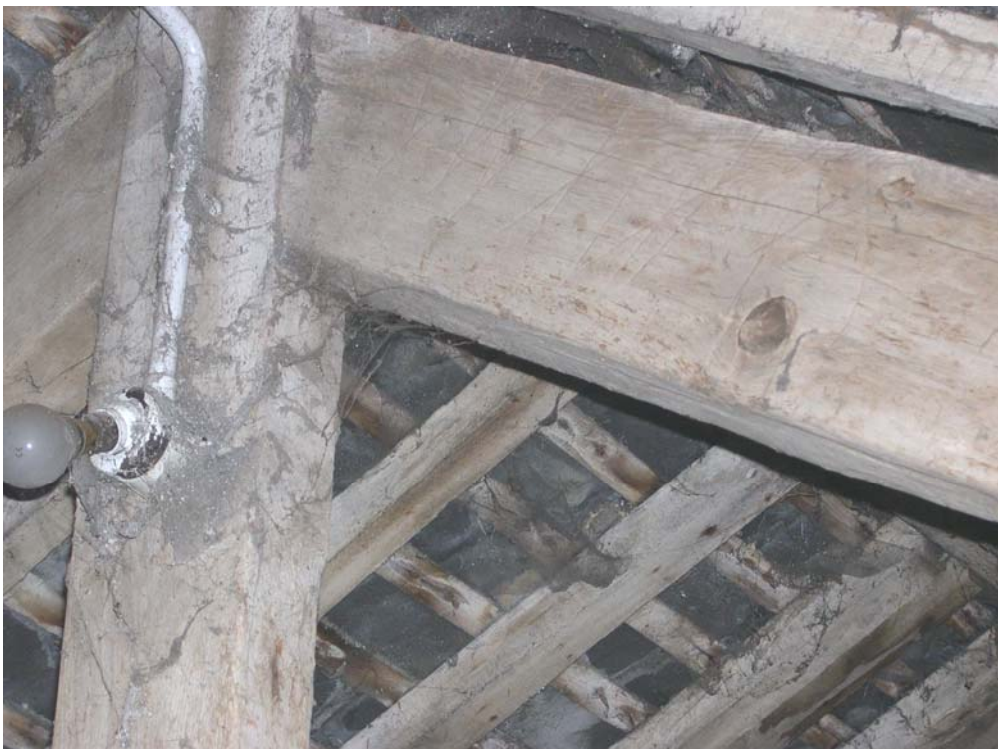
Plate 22: Detail of the Baltic timber marks on the central truss
