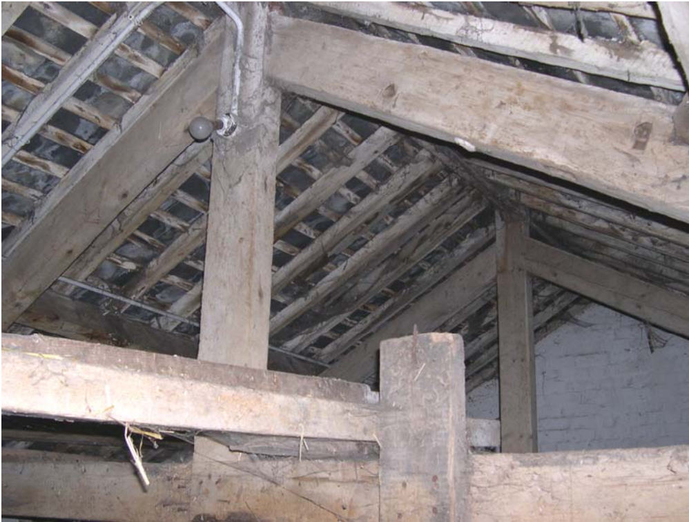
Plate 21: North-west-facing view of the central kingpost truss in Box One
