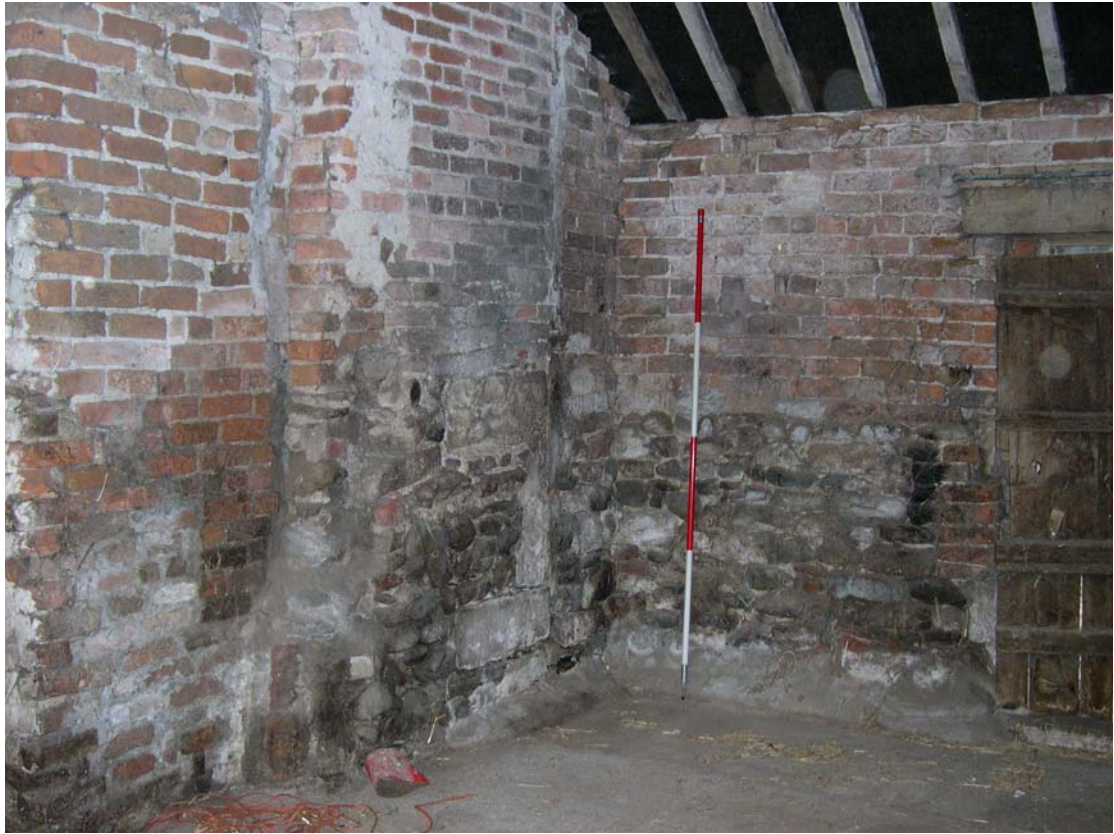
Plate 10: The north-west corner of the barn showing phases of stone and brick building
