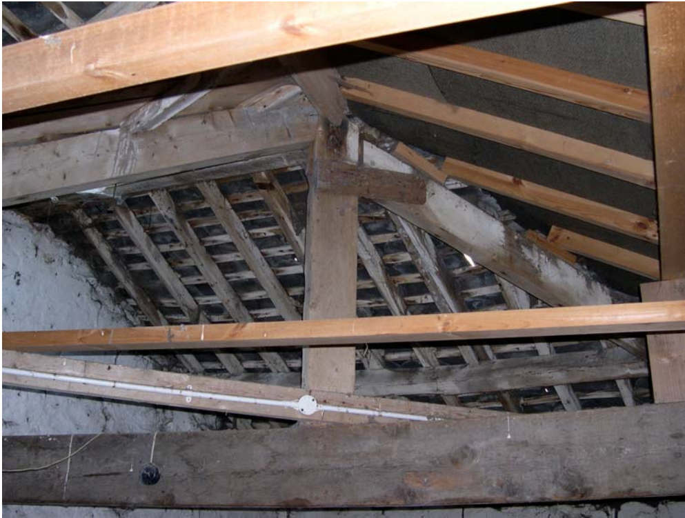
Plate 23 Detail of the recently replaced ceiling in Box Three
