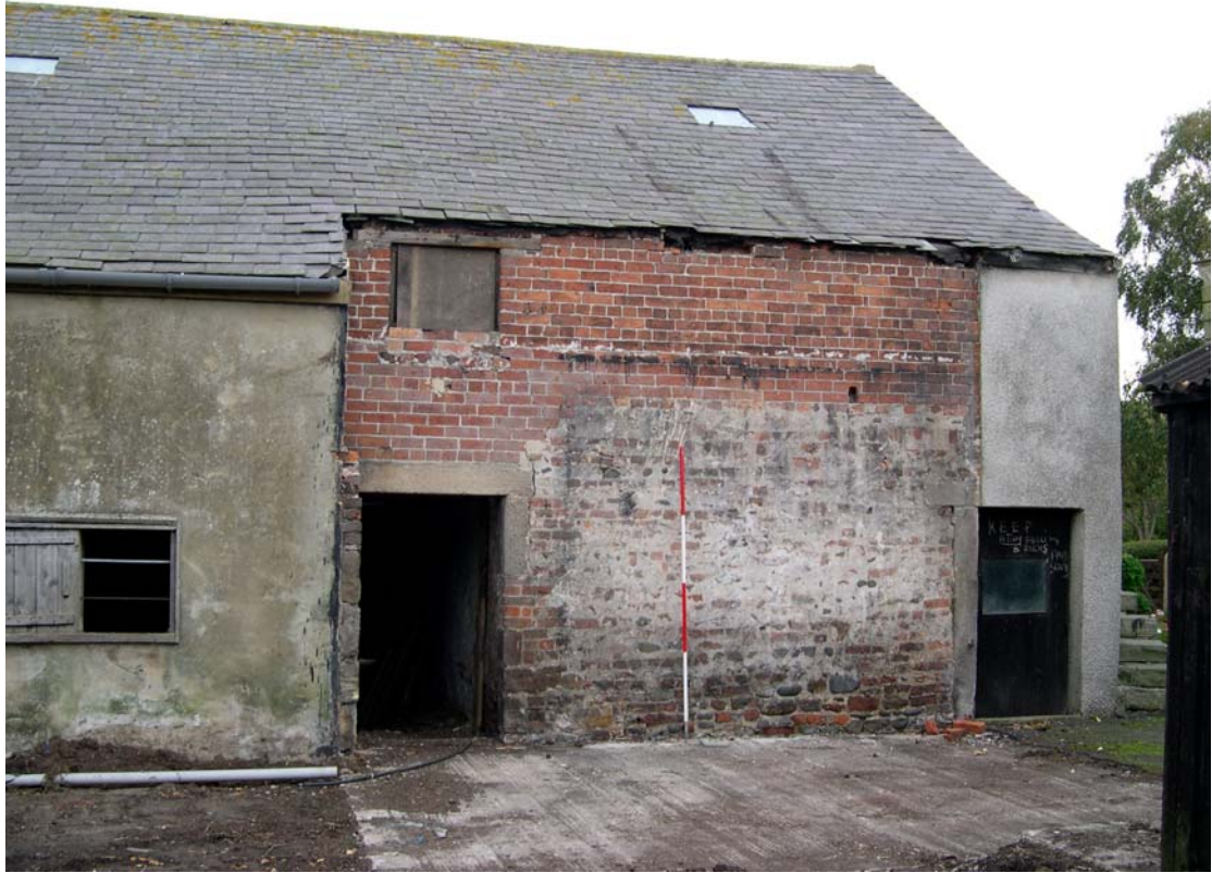
Plate 5: The south end of the west external elevation of the barn
