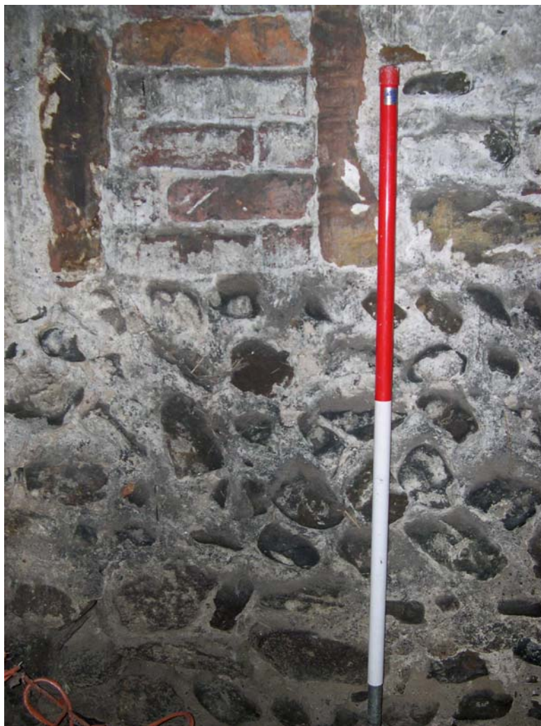
Plate 14: Blocked ventilation slot covered by the granary
