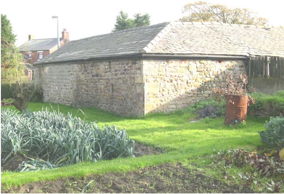
Plate 19: The north elevation of the east/west axis of the cow sheds
