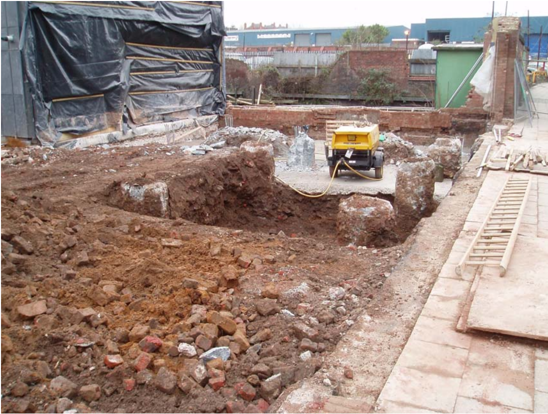
Plate 5: View looking west across the lift shaft pit, showing the concrete piles dating to the mid-20 th century
