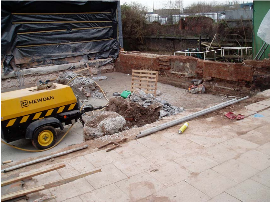
Plate 4: General view looking south-west across the site
