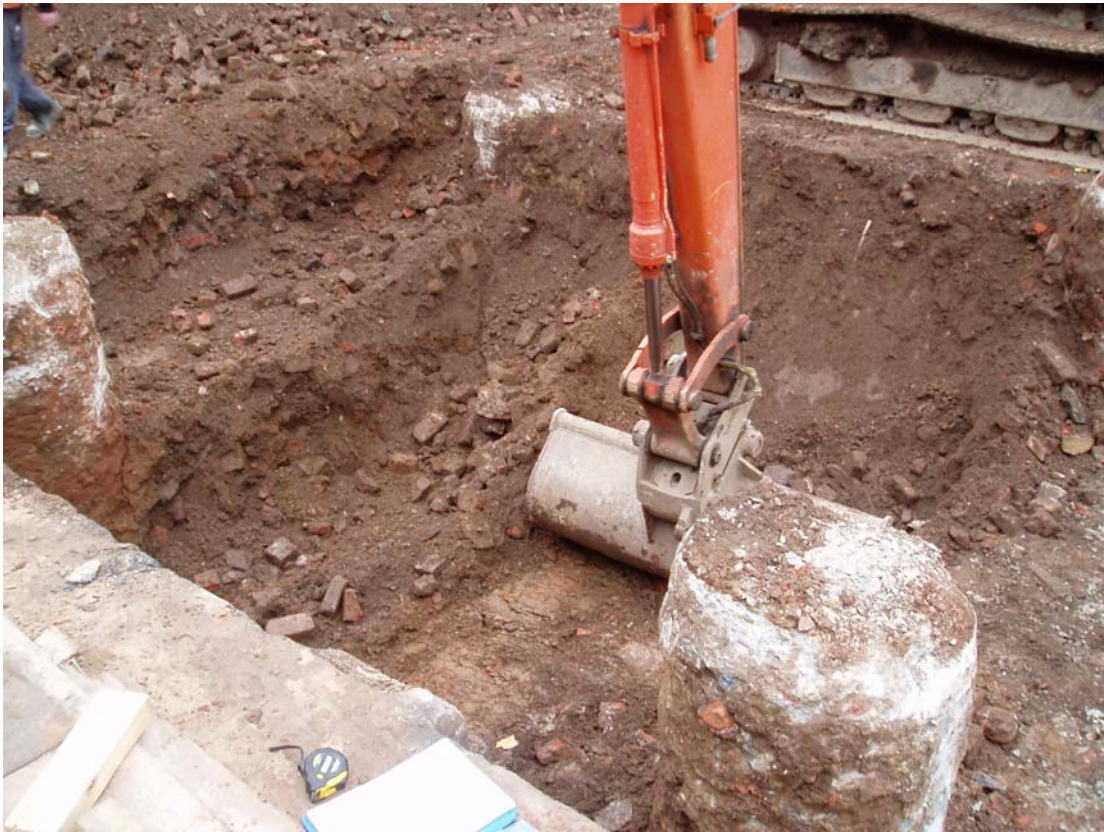
Plate 6: The lift shaft pit during excavation, showing 20 th -century demolition material
