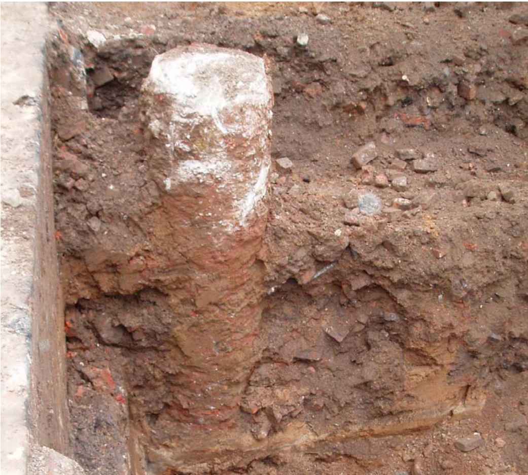
Plate 8: One of the 20 th -century concrete piles
