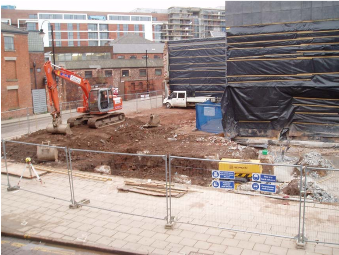
Plate 3: General view looking south-east across the site, showing the position of the lift shaft pit in the foreground
