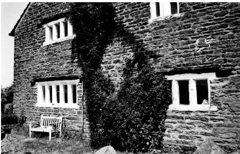
Plate 11: The label mouldings and stone mullioned windows on the south elevation of the cottage
