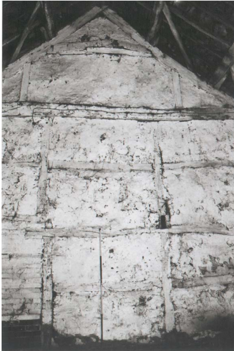
Plate 9: The wattle and daub wall, featuring the truss with queen struts in place
