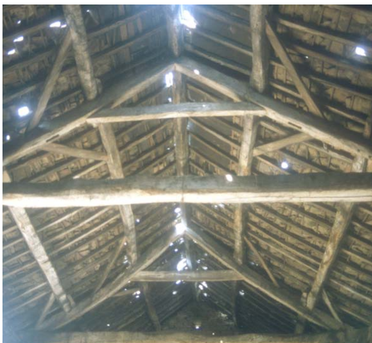
Plate 8: North-facing view of the queens-post trusses in the barn
