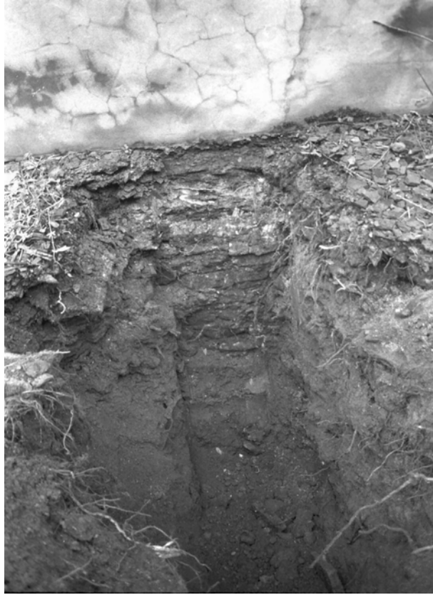
Plate 3: Trial Pit 2, showing the foundation of the adjacent property, looking north
