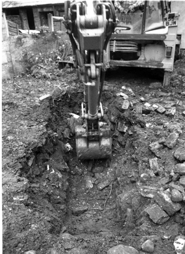
Plate 4: Trial Pit 5 during excavation, looking east.
