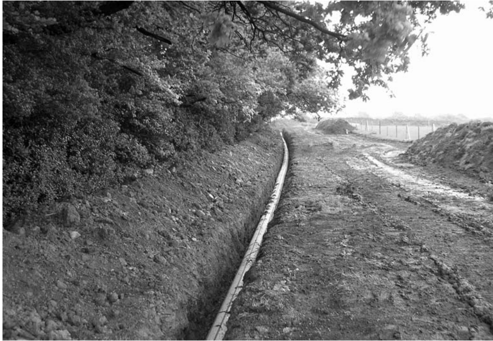
Plate 3: Laying of gas pipe, Field 4 looking east
