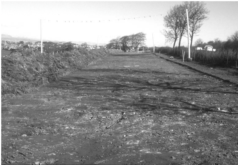
Plate 2: Excavated pipeline easement, Field 3 looking north
