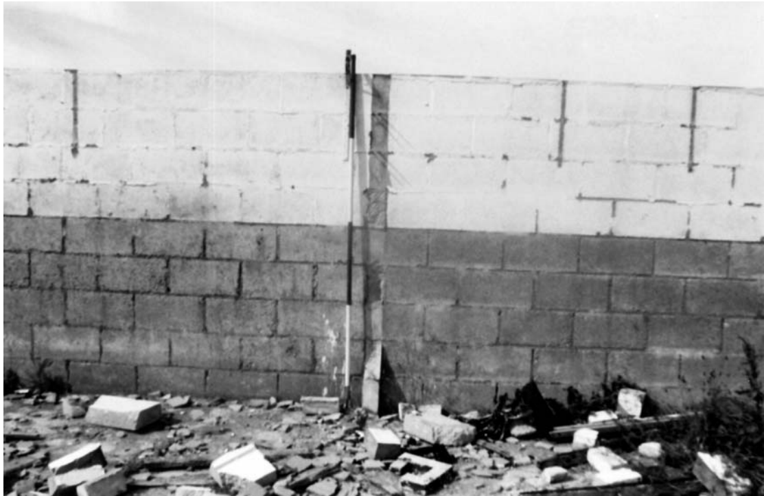
Plate 12: Scar of a partition wall within the east elevation, looking west
