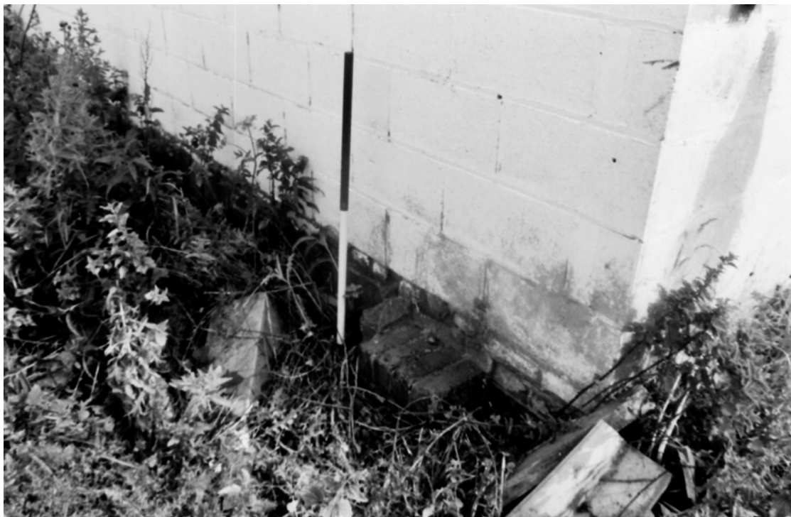
Plate 13: Brick buttress against the west elevation, looking north-east
