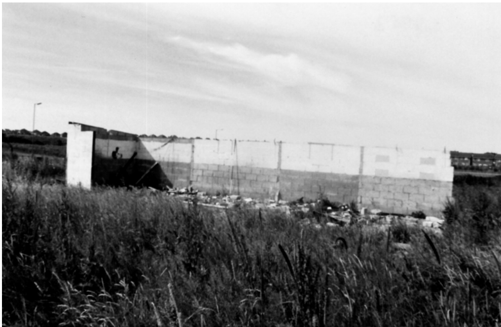
Plate 11: East Elevation of Building 1, looking south-west
