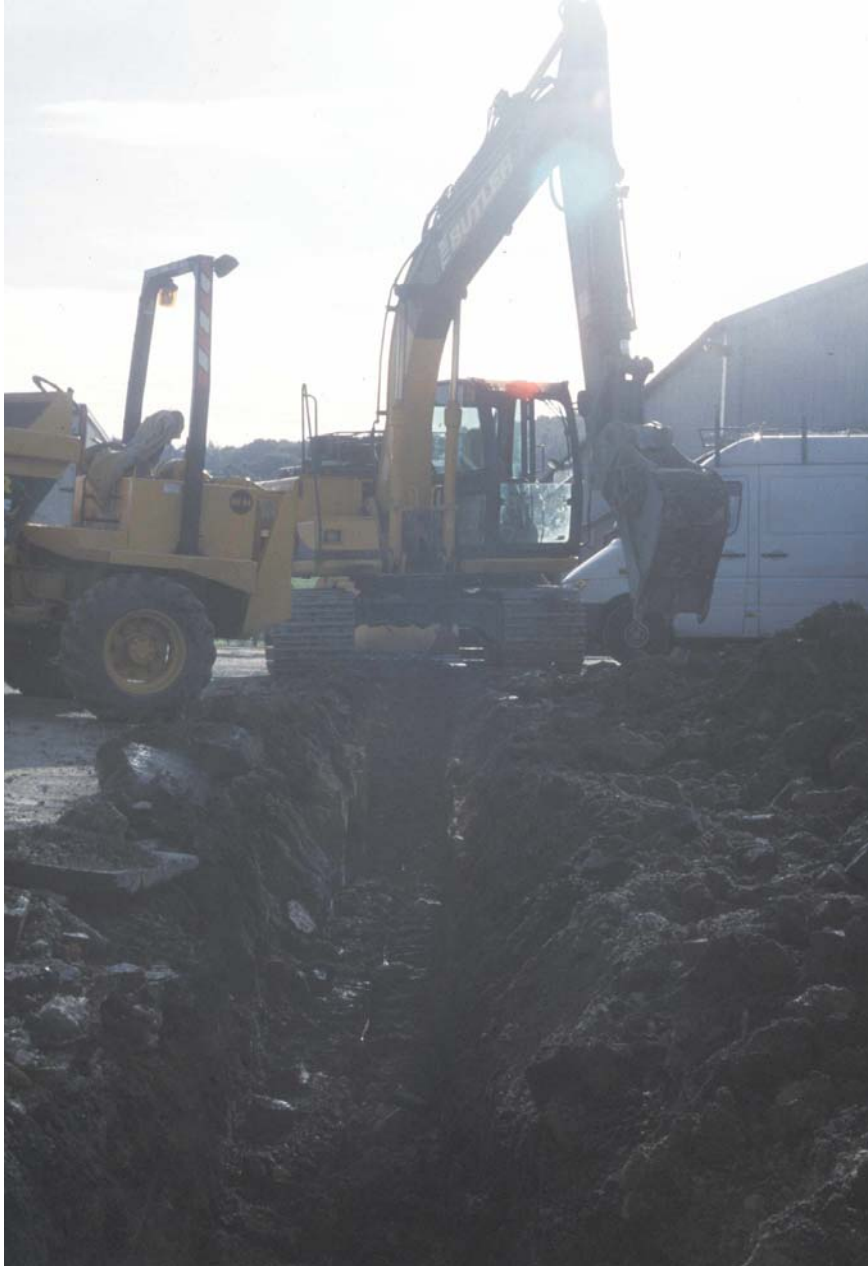
Plate 3: General working of trench under excavation
