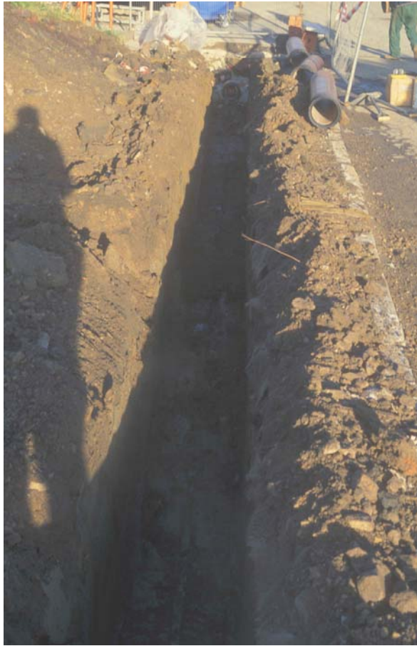
Plate 1: Excavated drainage trench
