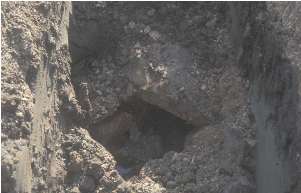
Plate 2: Stone drain within drainage trench
