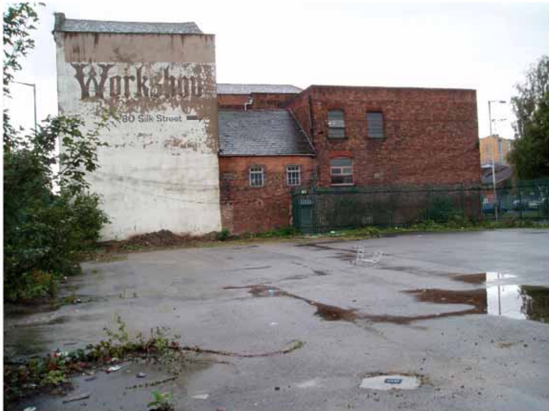
Plate 1: View looking west across the scheme area
