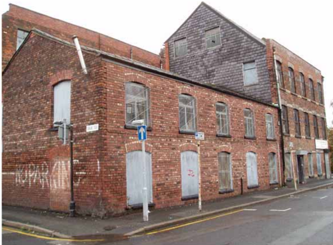
Plate 3: Buildings fronting Radium Street, forming western end of study area
