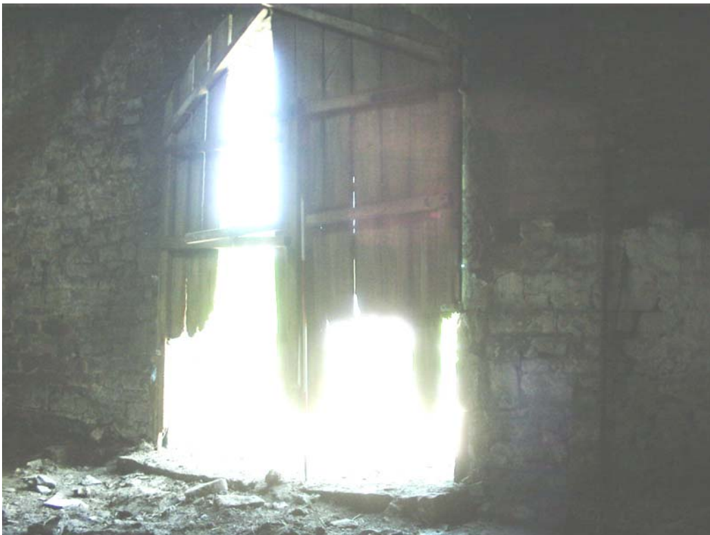
Plate 8: The east internal elevation of the barn featuring the wagon doors
