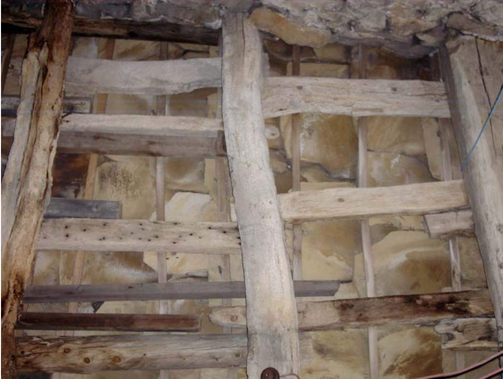
Plate 13: The roof of the outshut on the west of the barn
