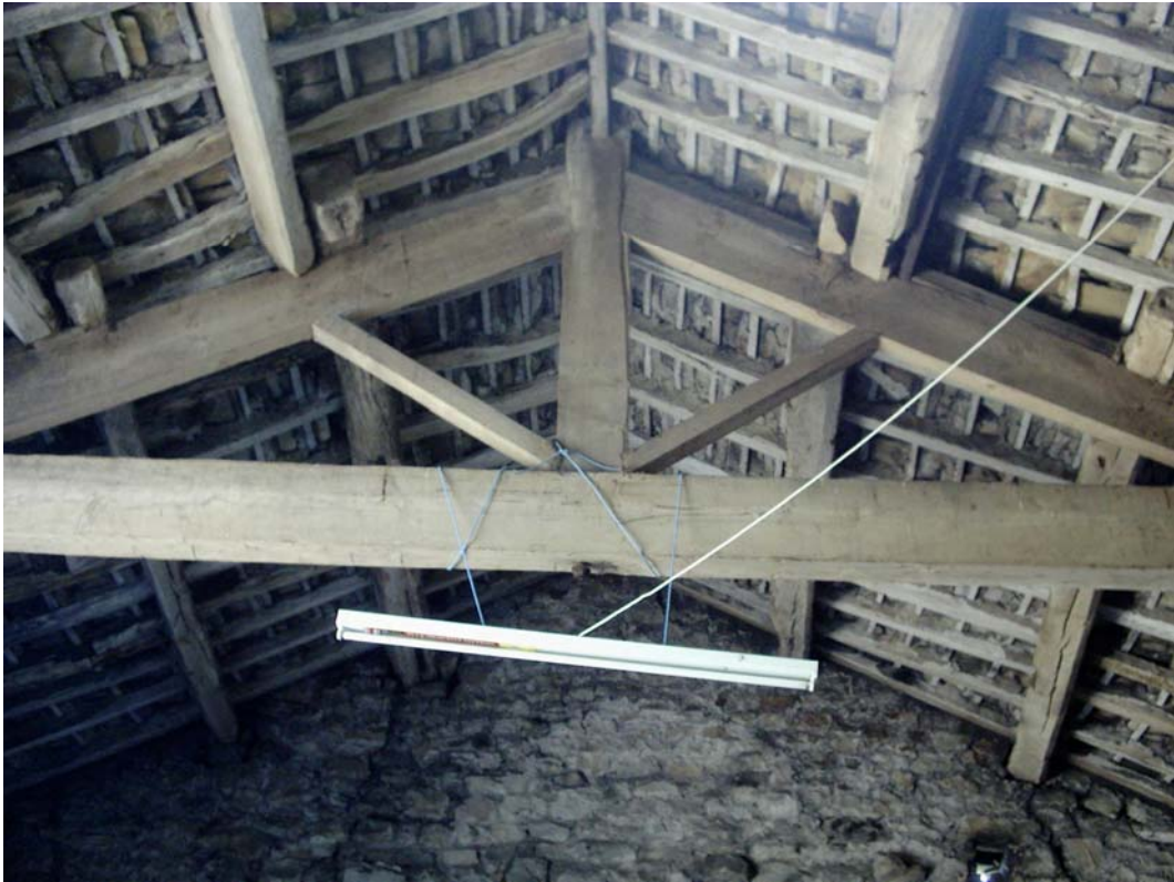
Plate 5: Detail of the roof truss
