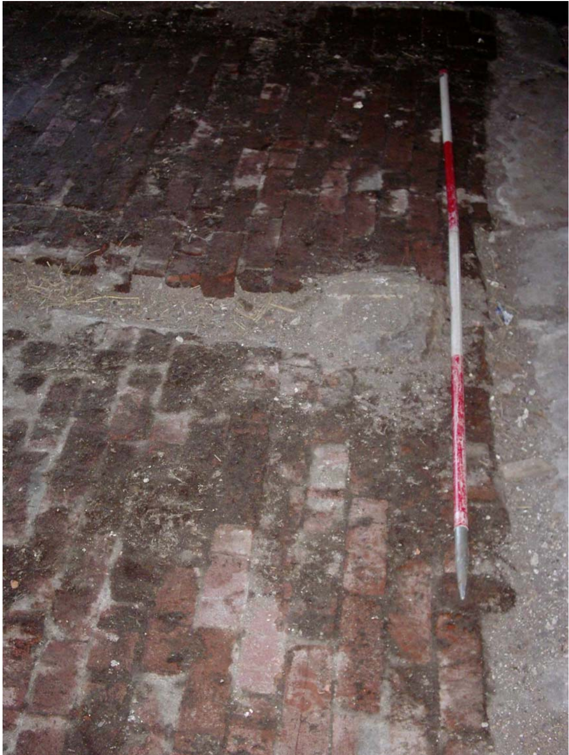
Plate 12: The brick floor at the south end of the building, featuring scars from the removed partitions
