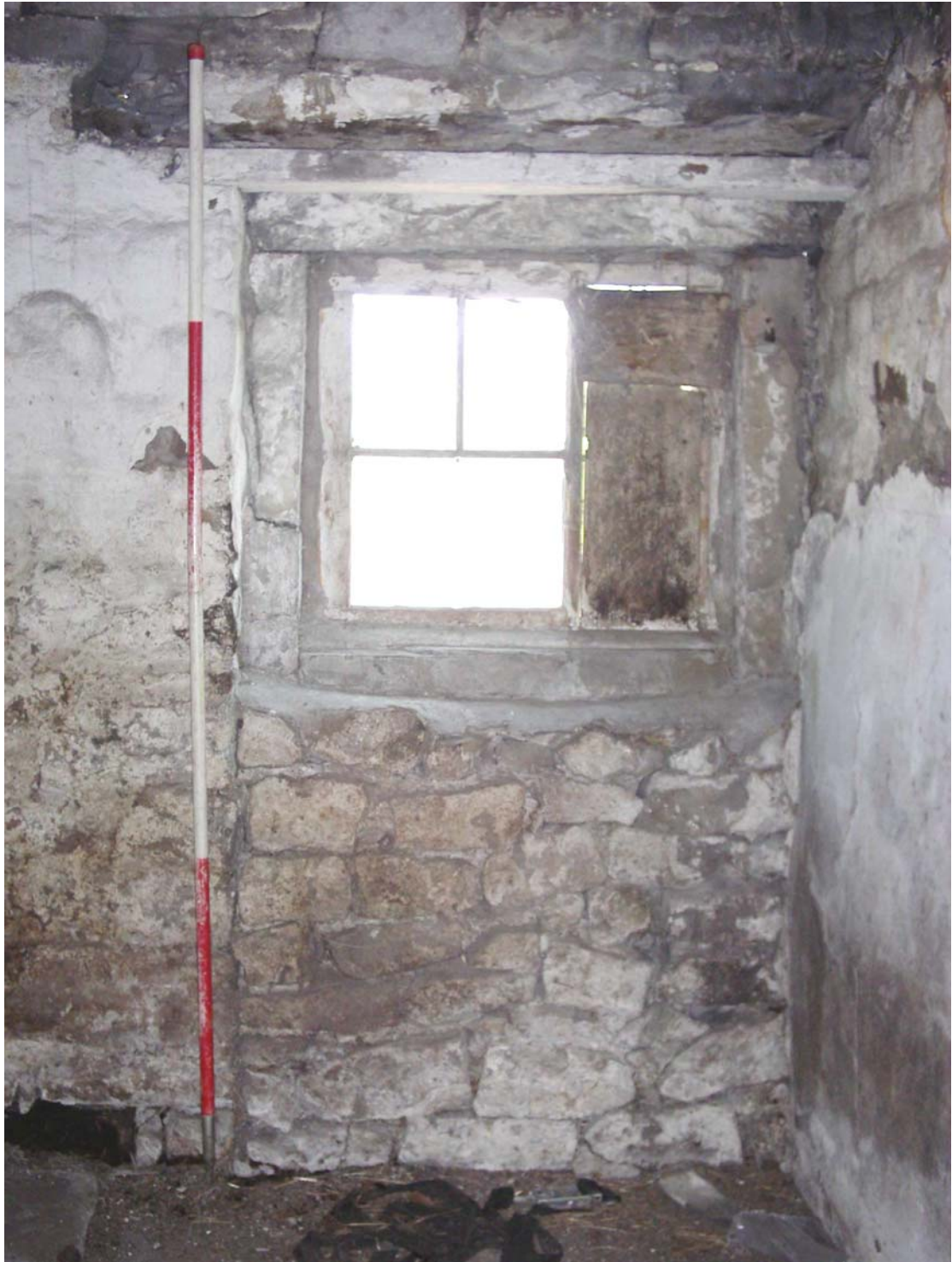
Plate 9: Partially blocked door on the east elevation
