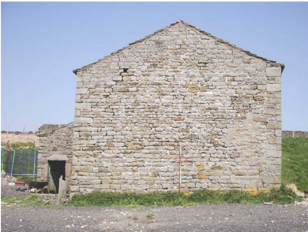
Plate 2: The south elevation of the barn
