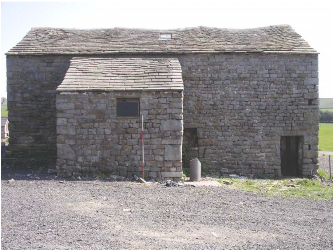
Plate 4: The west elevation of the barn
