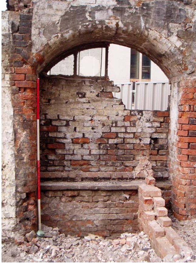
Plate 12: Blocking of window in north elevation, Bay 13
