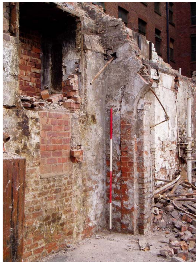
Plate 21: Internal partition wall within Bay 13
