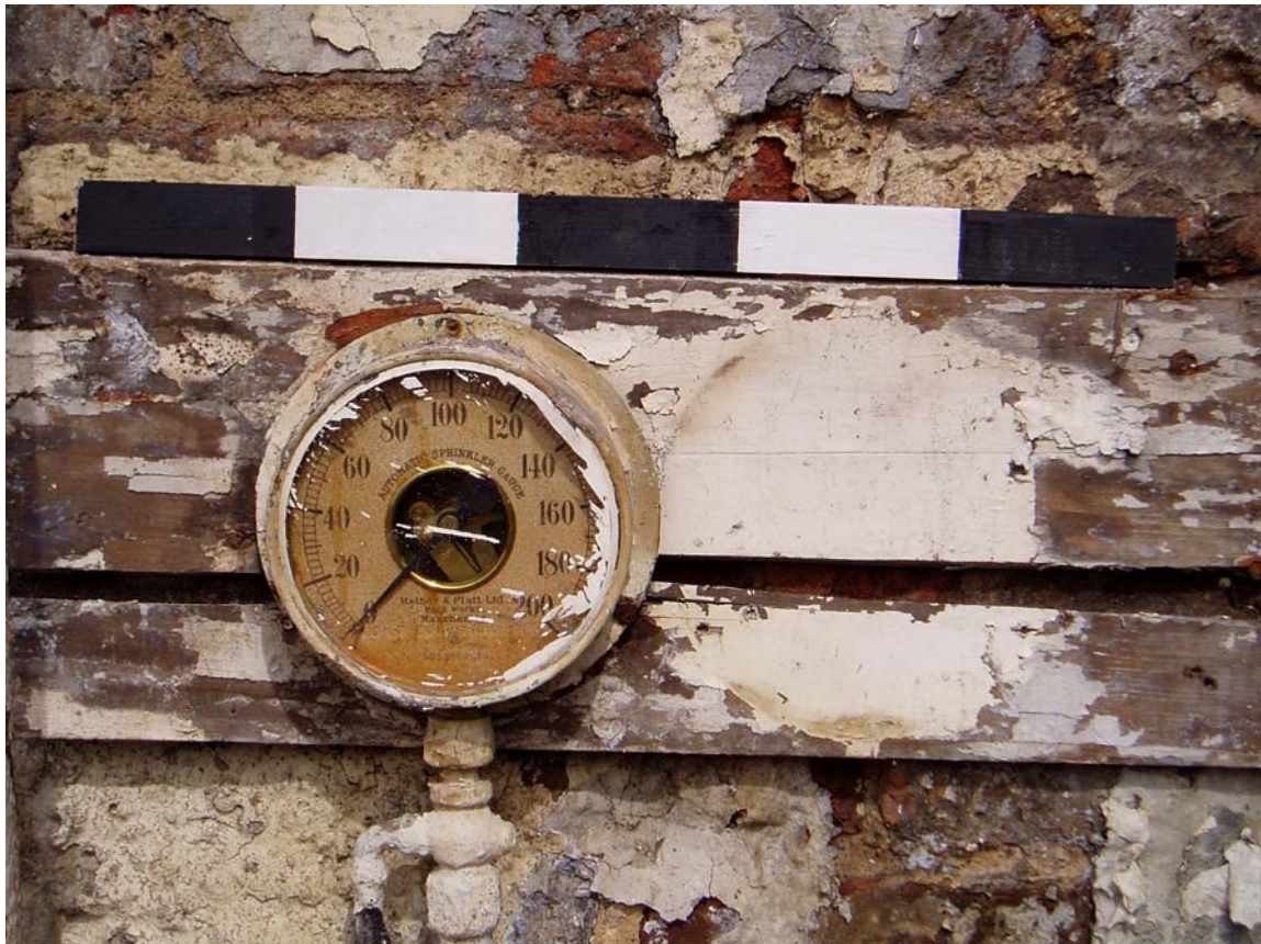
Plate 18: Pressure gauge from Automatic Sprinkler System
