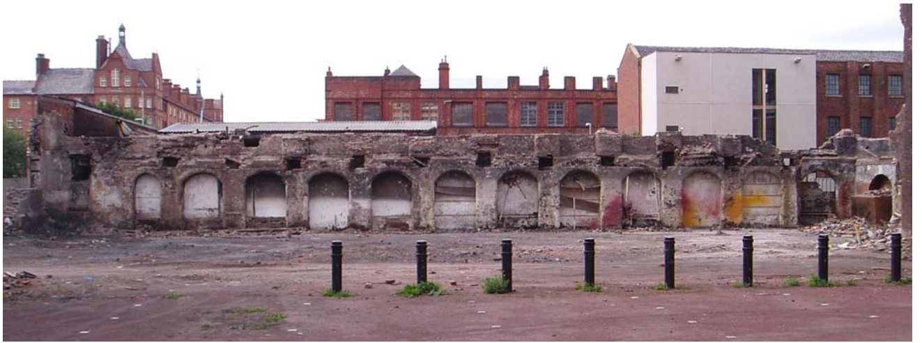
Plate 8: North internal elevation of the Bengal Street block, following emergency demolition
