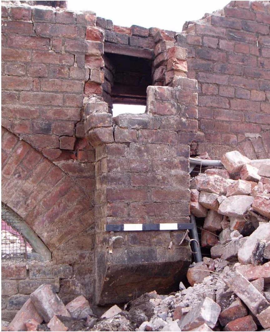
Plate 14: External detail of heating tower base, between Bays 11 and 12
