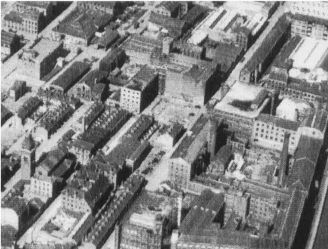
Plate 1: Aerial view of Ancoats taken in 1958, looking north-east, showing the study area
