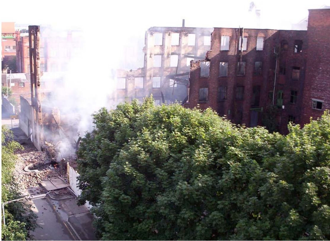
Plate 6: The smouldering remains of the Bengal Street block after the fire in July 2005
