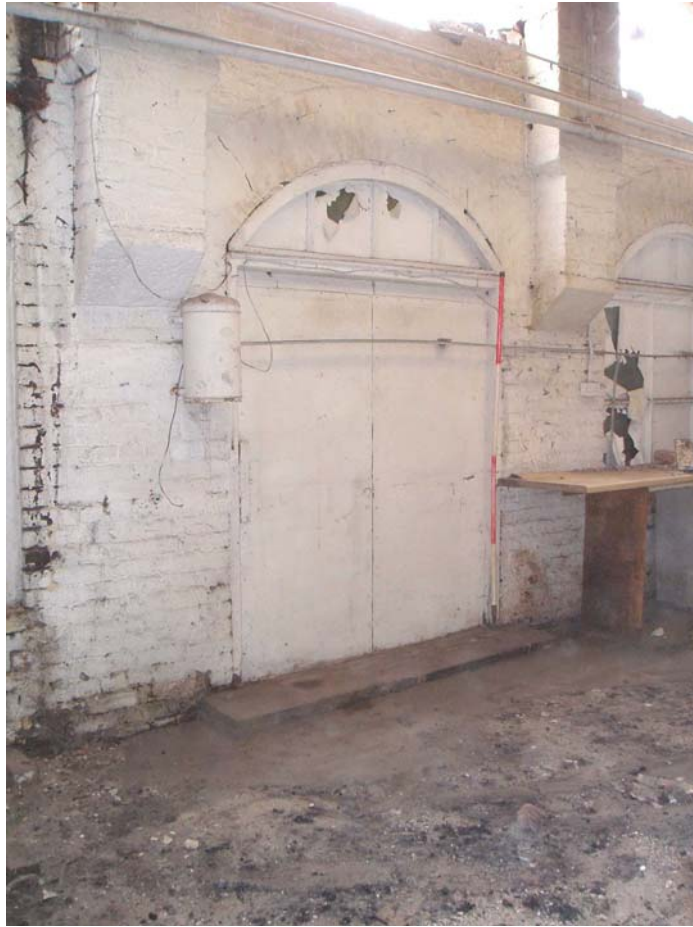
Plate 10: Full height opening in Bay 7, with external step
