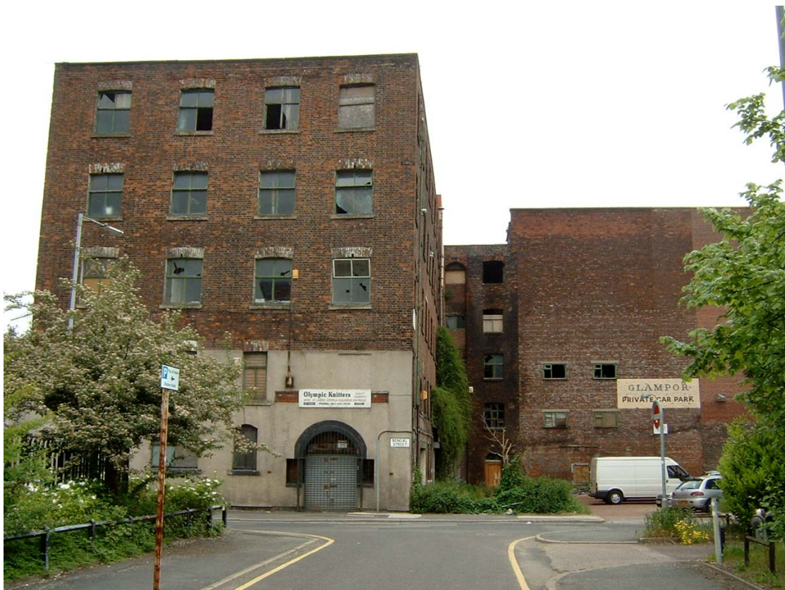
Plate 5: The south-west-facing elevation of the Bengal Street block in June 2005
