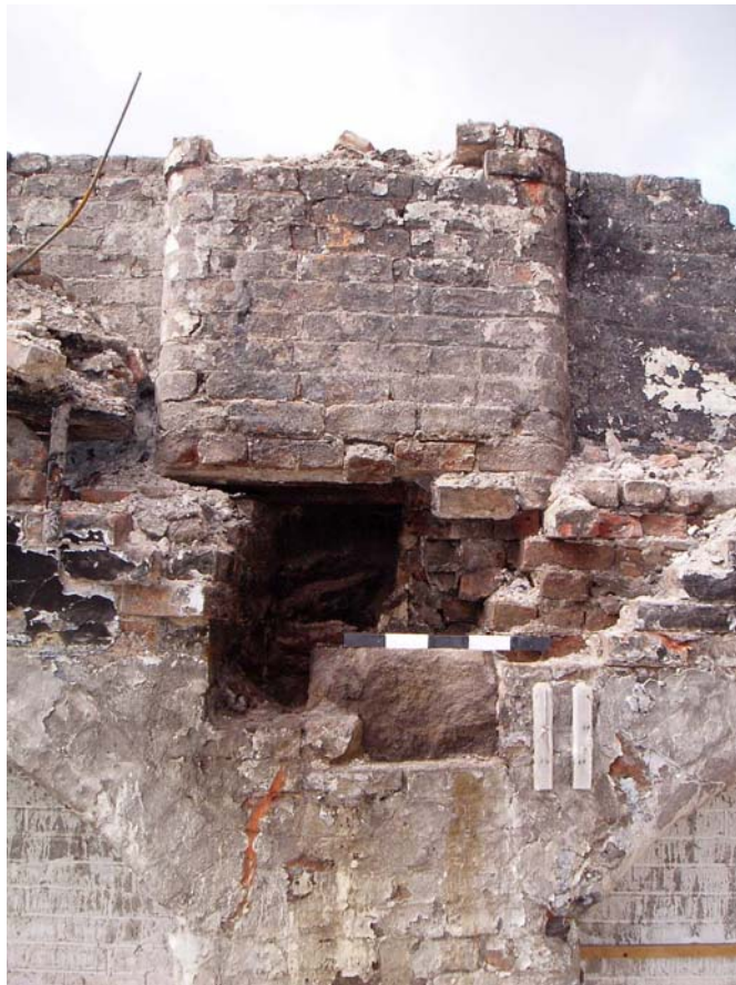
Plate 13: Detail of base of heating tower flue, between Bays 11 and 12
