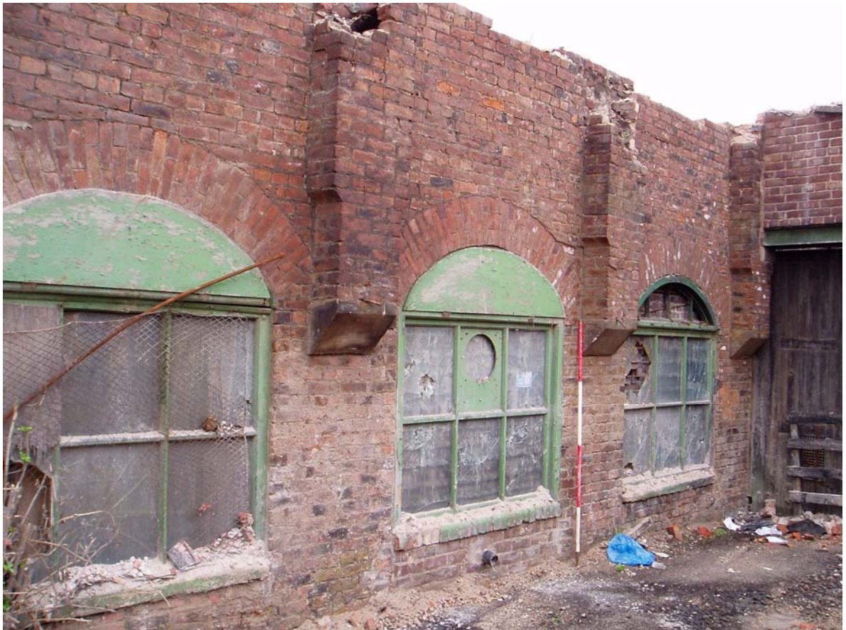
Plate 9: Original windows in north face of Bengal Street block
