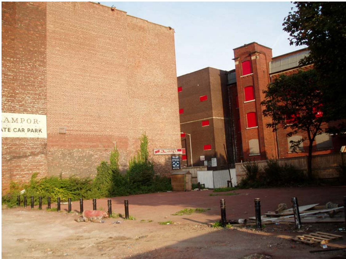
Plate 22: View looking south-east across the study area towards Jersey Street
