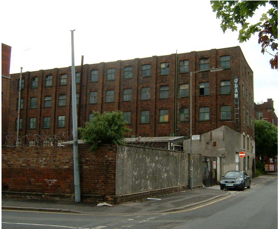
Plate 4: The north-west-facing elevation of the Bengal Street block in June 2005
