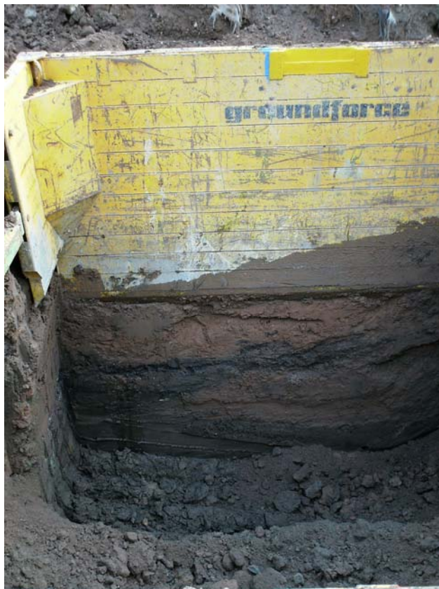
Plate 6: Trench 3 base prior to seating of box
