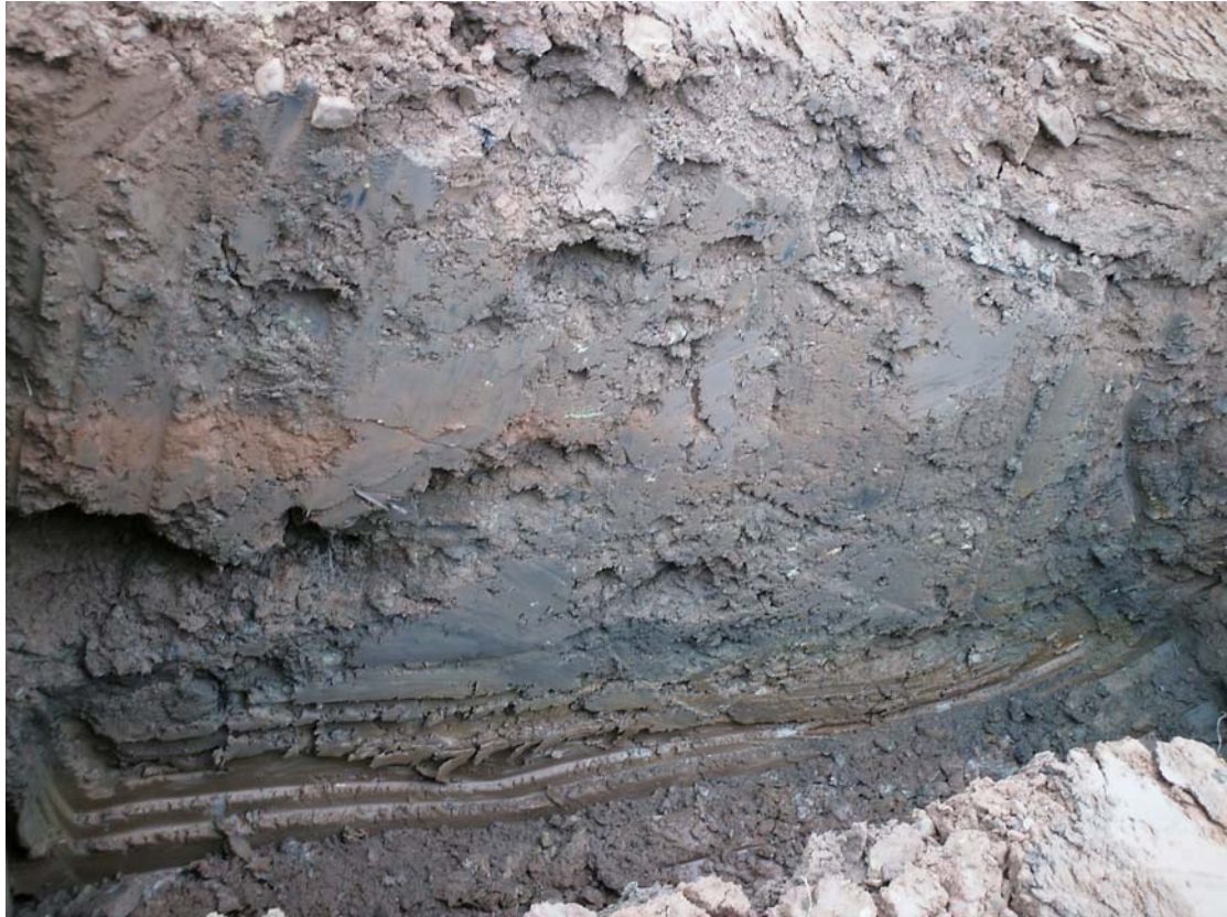
Plate 5: Trench 3 section showing bands of made up ground with rubble deposits
