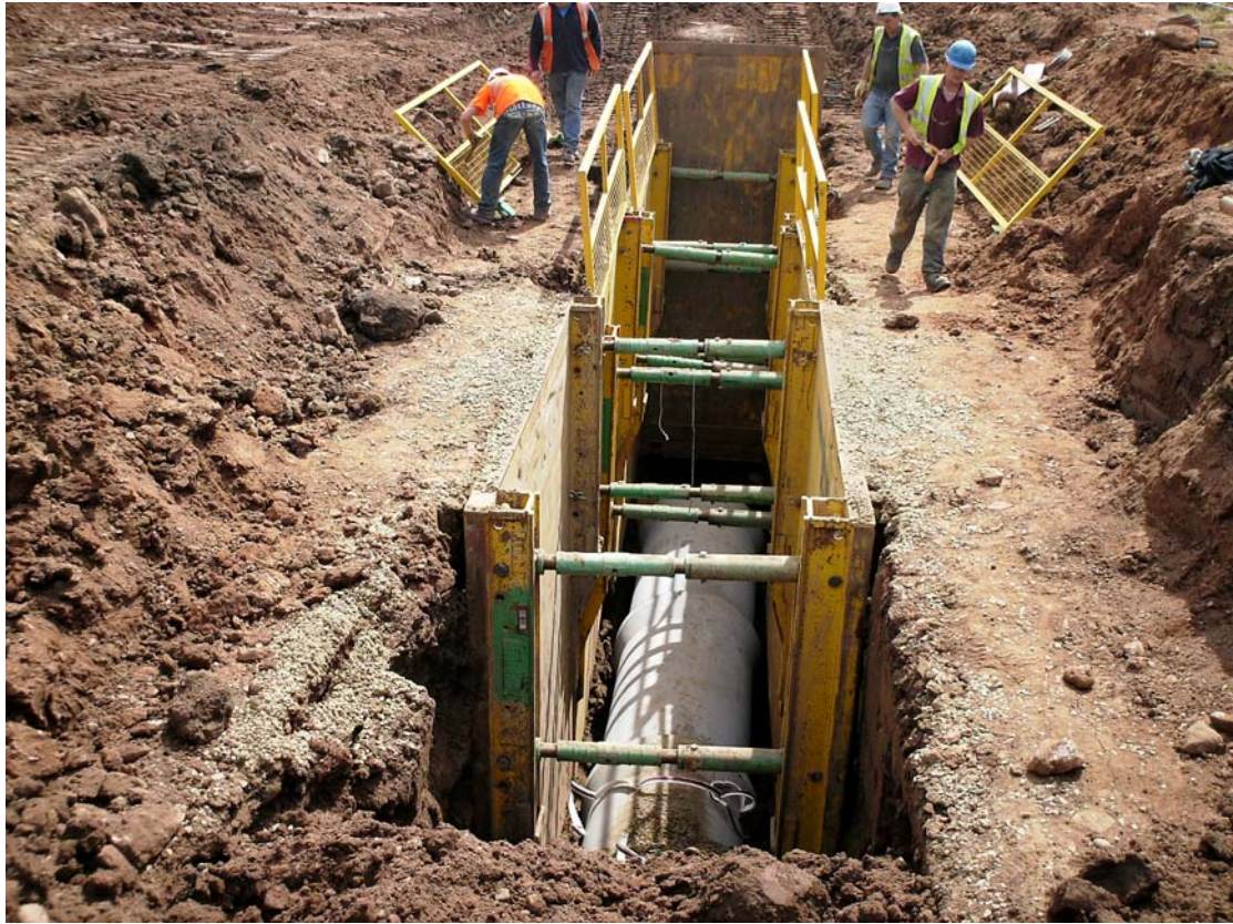
Plate 1: Working shot of Trench 1 looking south
