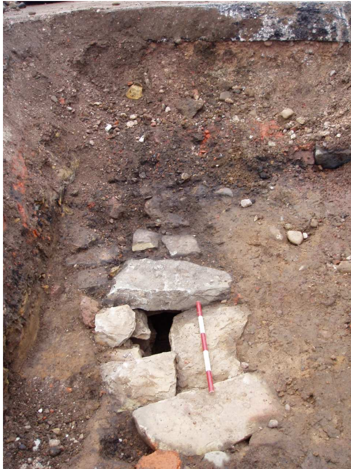
Plate 7: Detail of culvert 137 , Trench 2, looking north
