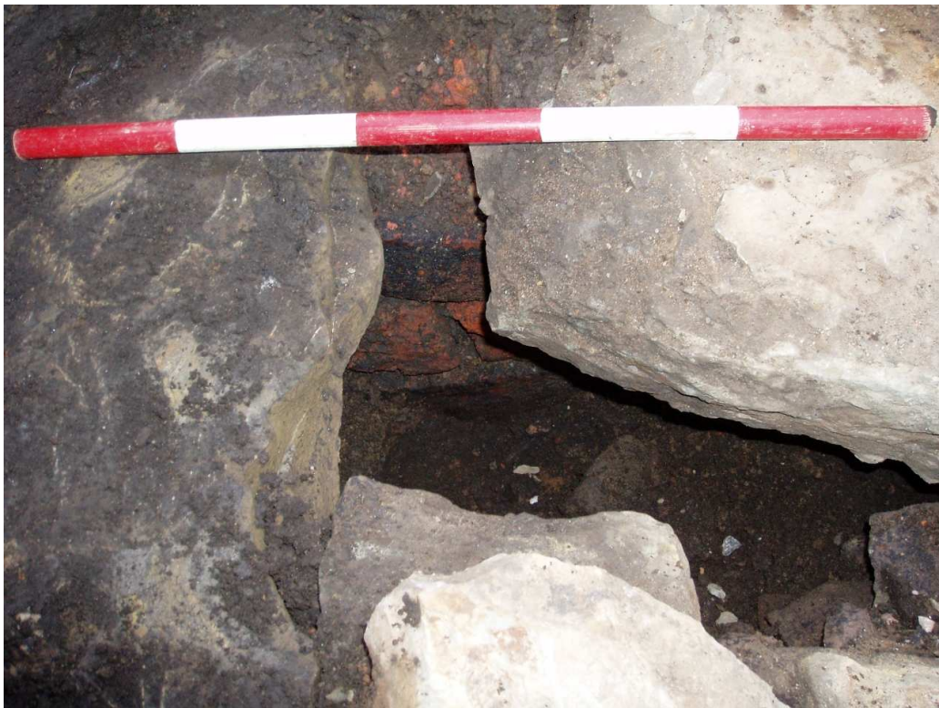
Plate 8: Detail of culvert 137 , Trench 2
