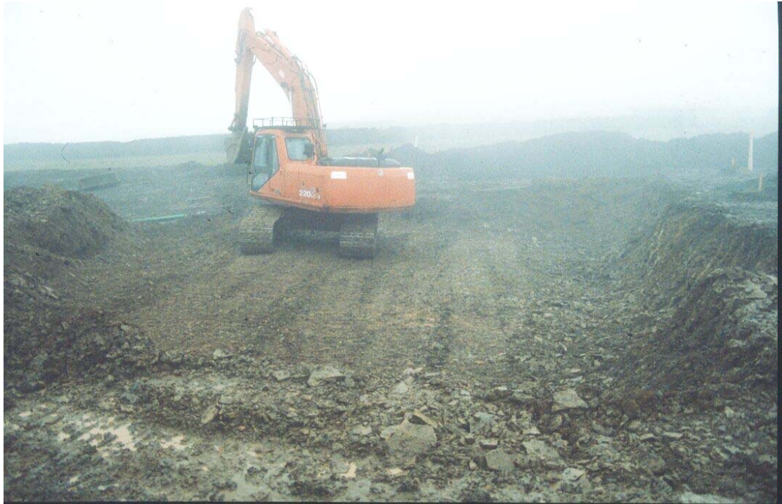
Plate 3: Working Shot showing Shale Geology beneath compound
