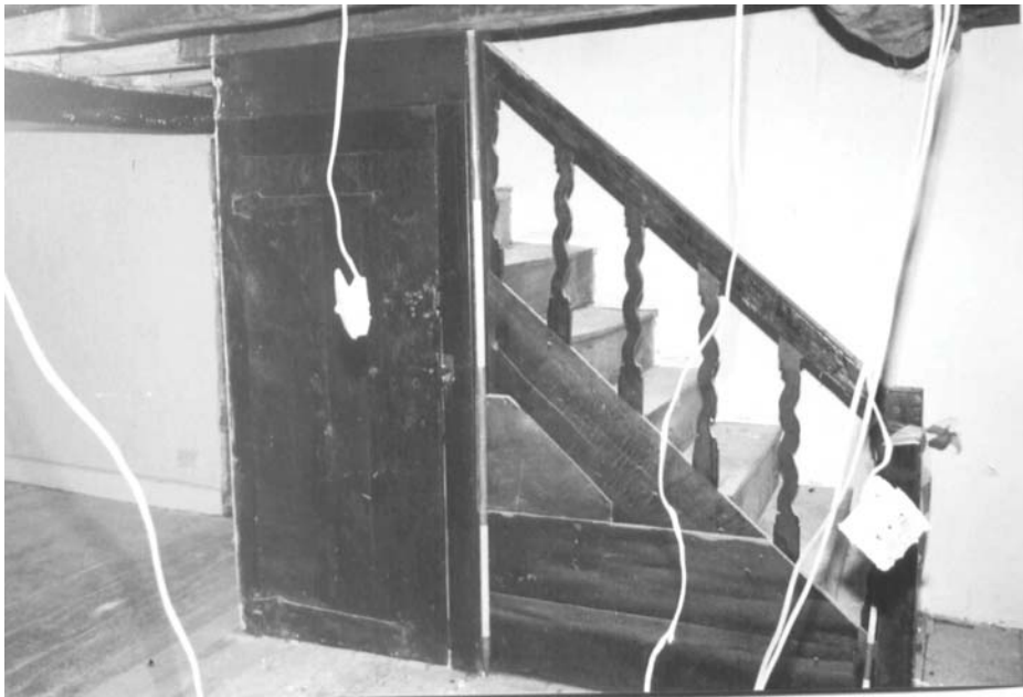
9: Original oak door and nineteenth century staircase in Room 16
