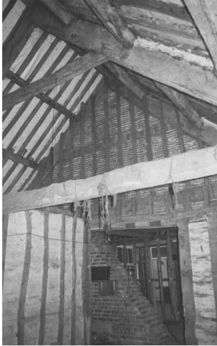
Plate 7: South-east-facing view of the roof truss and modern chimney-breast in Room 12
