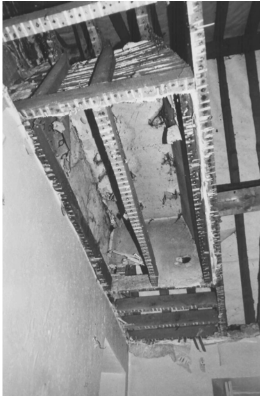
Plate 10: The lath and plaster 'smoke hood' above the fireplace,, Room 7
