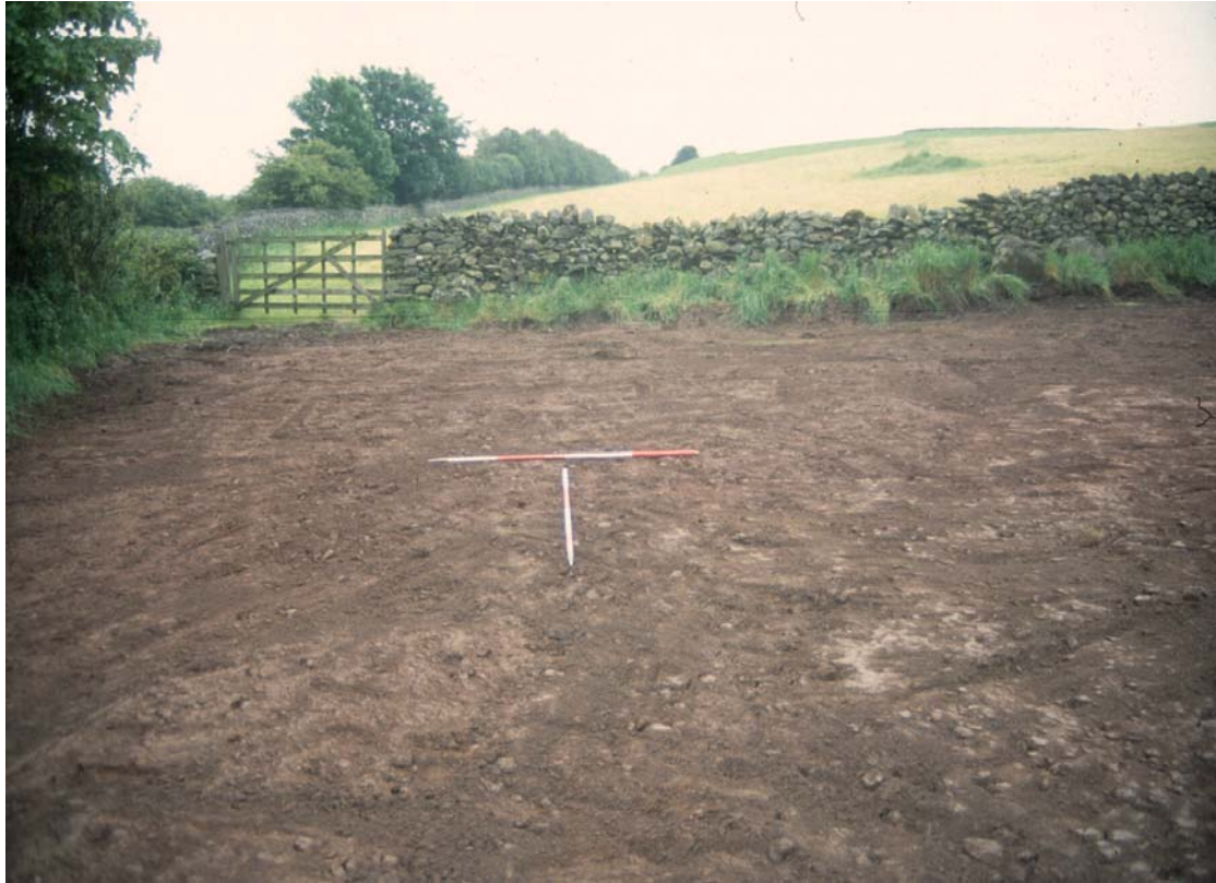
Plate 1: Topsoil strip facing south
