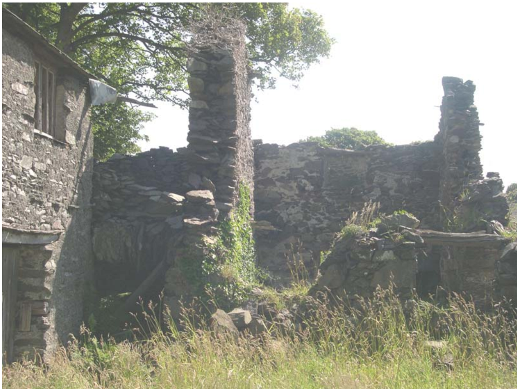
Plate 9: East-facing view of Elevation 7
