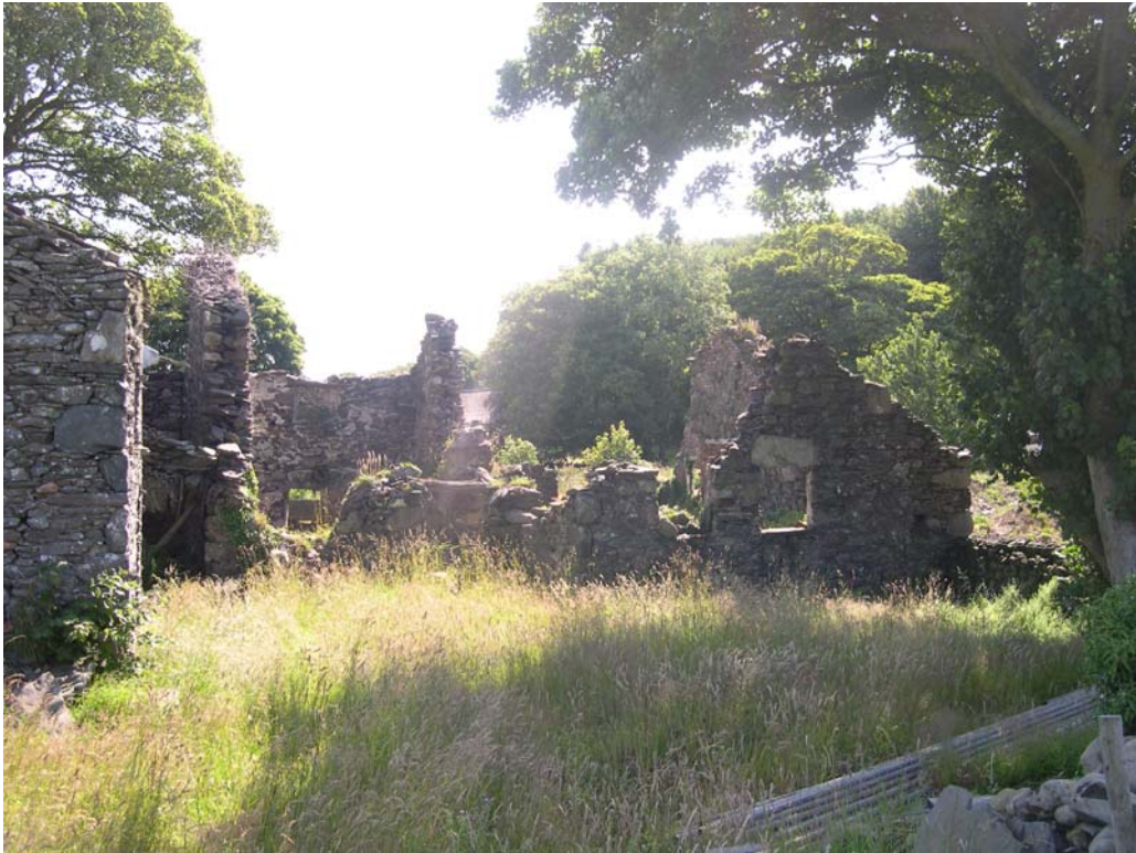
Plate 8: East-facing view of Elevation 5
