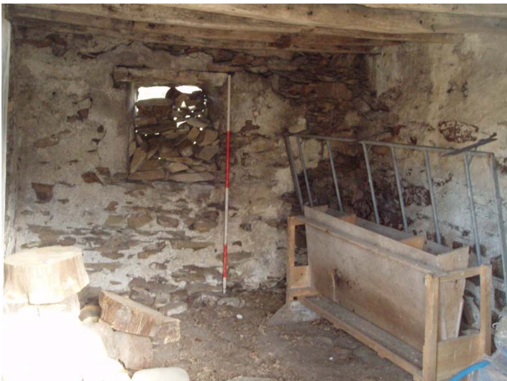
Plate 13: North-facing view of Room 2
