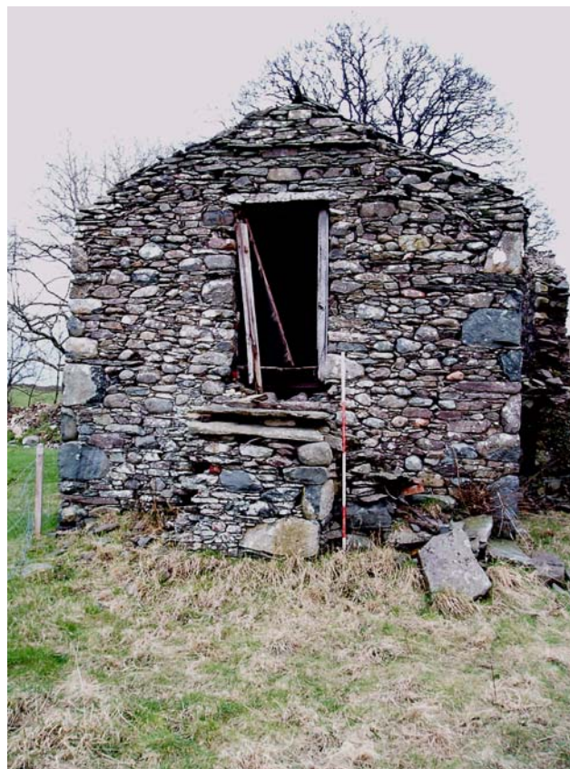
Plate 11: East-facing view of Elevation 9
