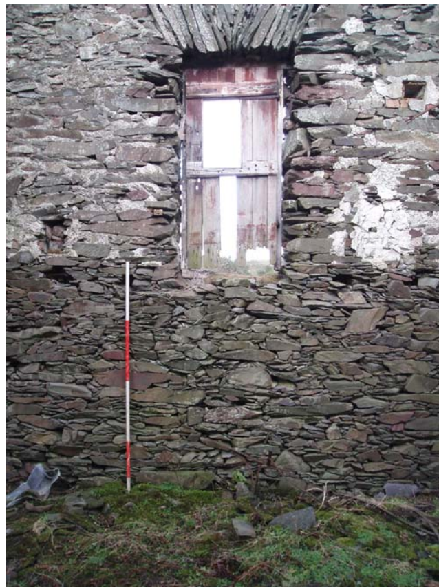
Plate 15: North-facing view of Room 4
