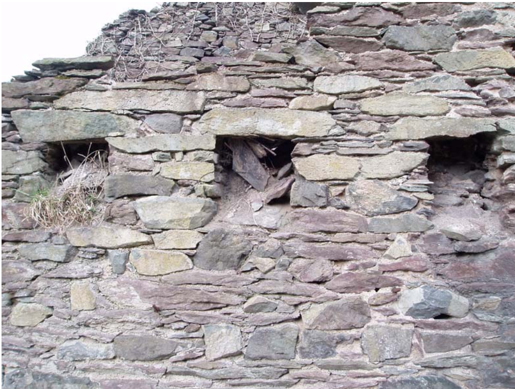
Plate 19: Detail of the flues within Elevation 16
