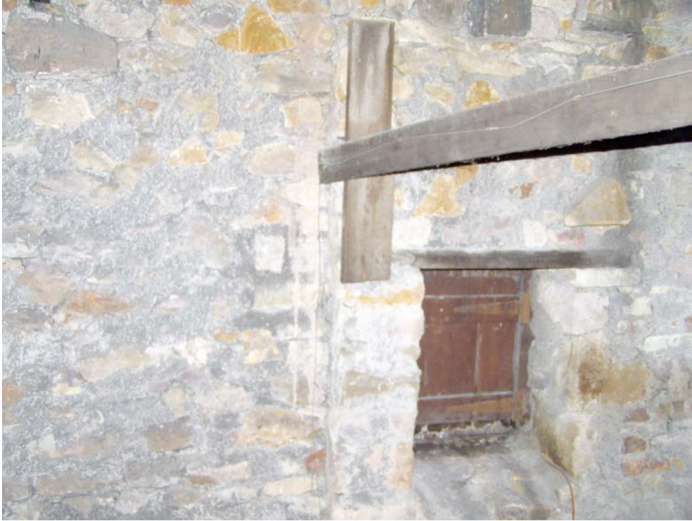
Plate 31: Hatch in east elevation of roof space
