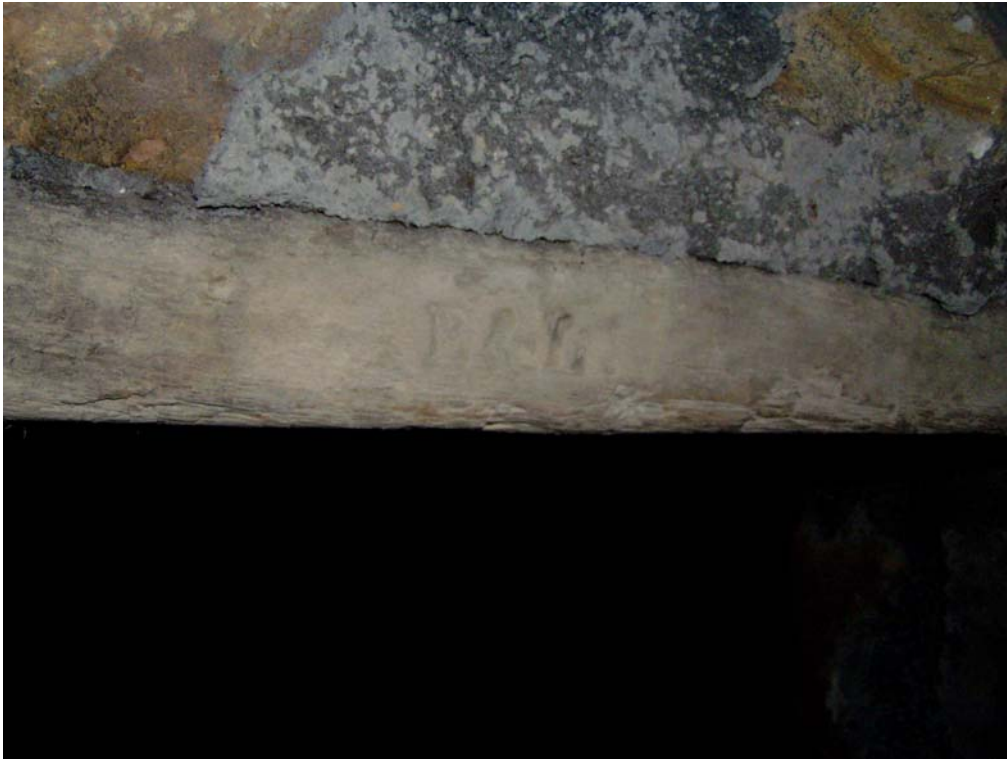
Plate 27: Initials 'B & L' in lintel
