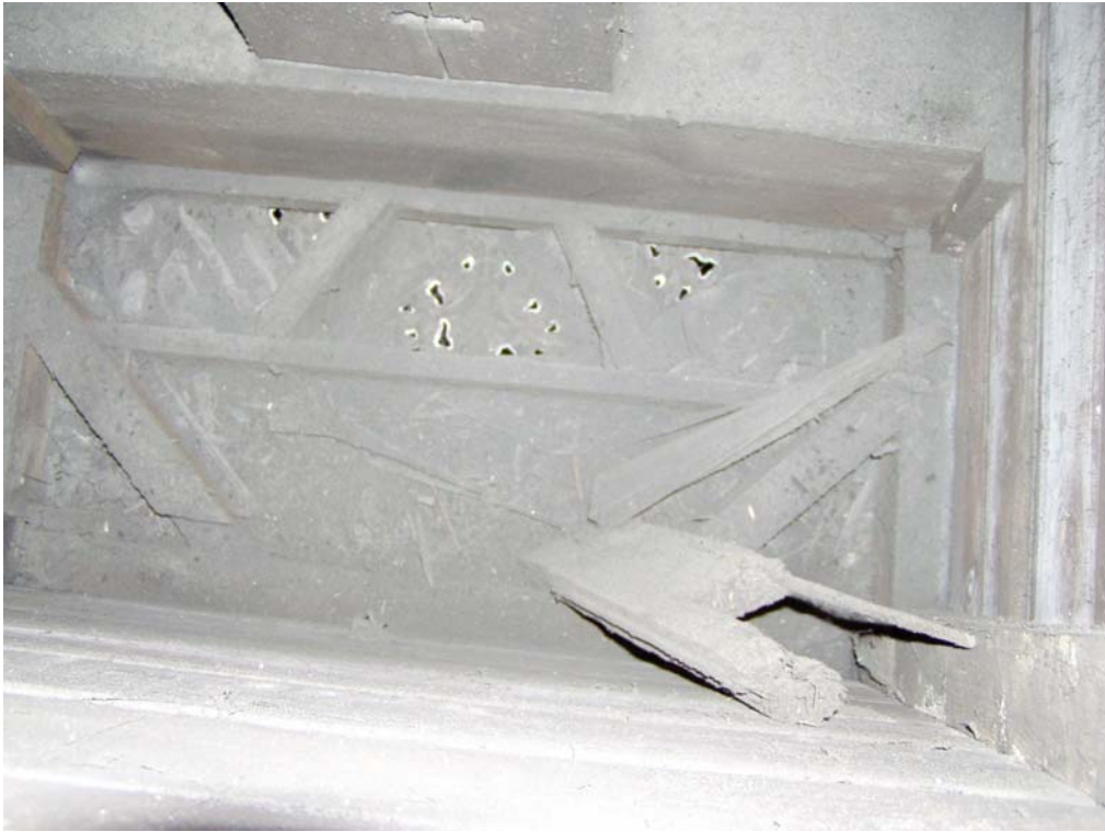
Plate 33: Perforations above ceiling rose
