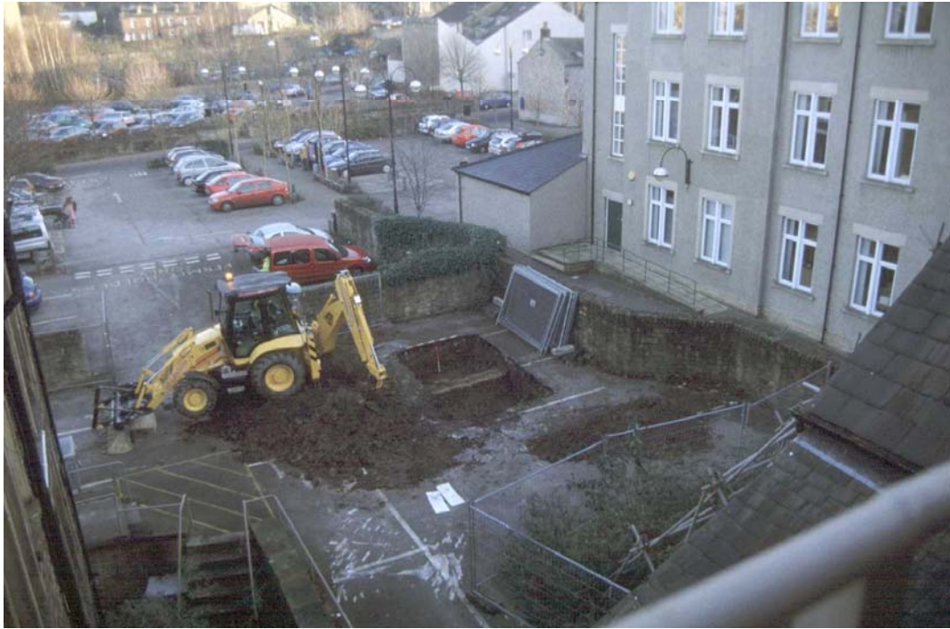
Plate 1: General shot of trench, facing east
