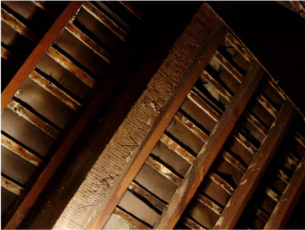
Plate 29: Baltic timber marks on soffit of west principal rafter
