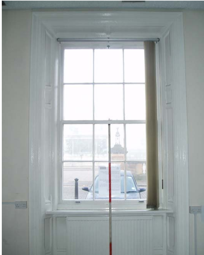
Plate 11: Sash window in Room 2
