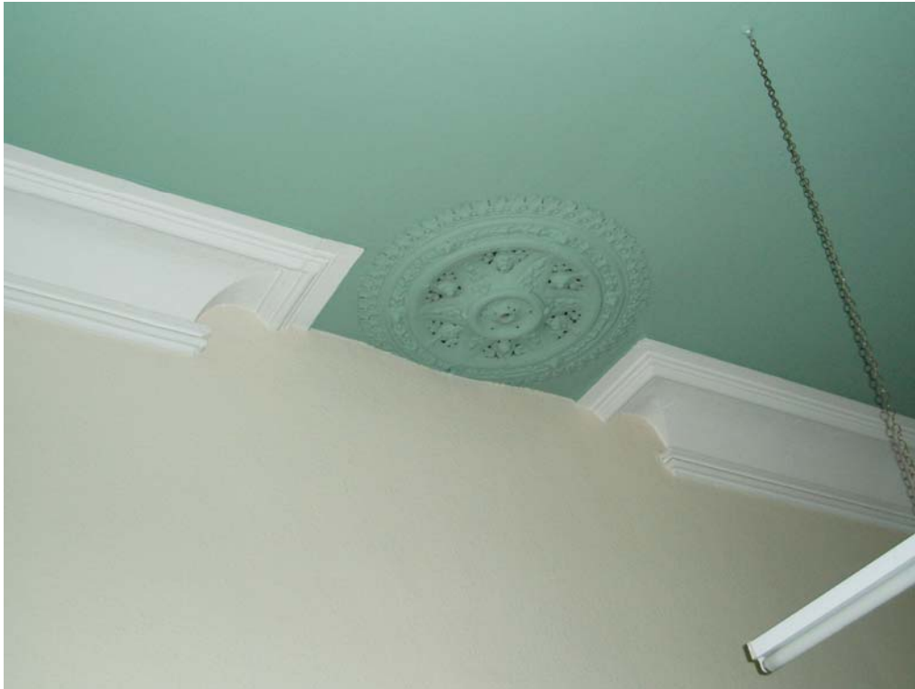
Plate 21: The cornice and ceiling rose in Room 8
