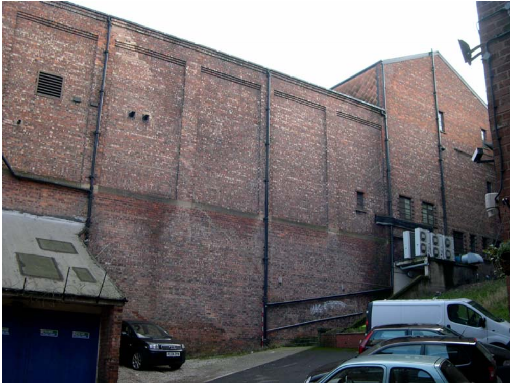
Plate 5: Western elevation of Gala bingo hall
