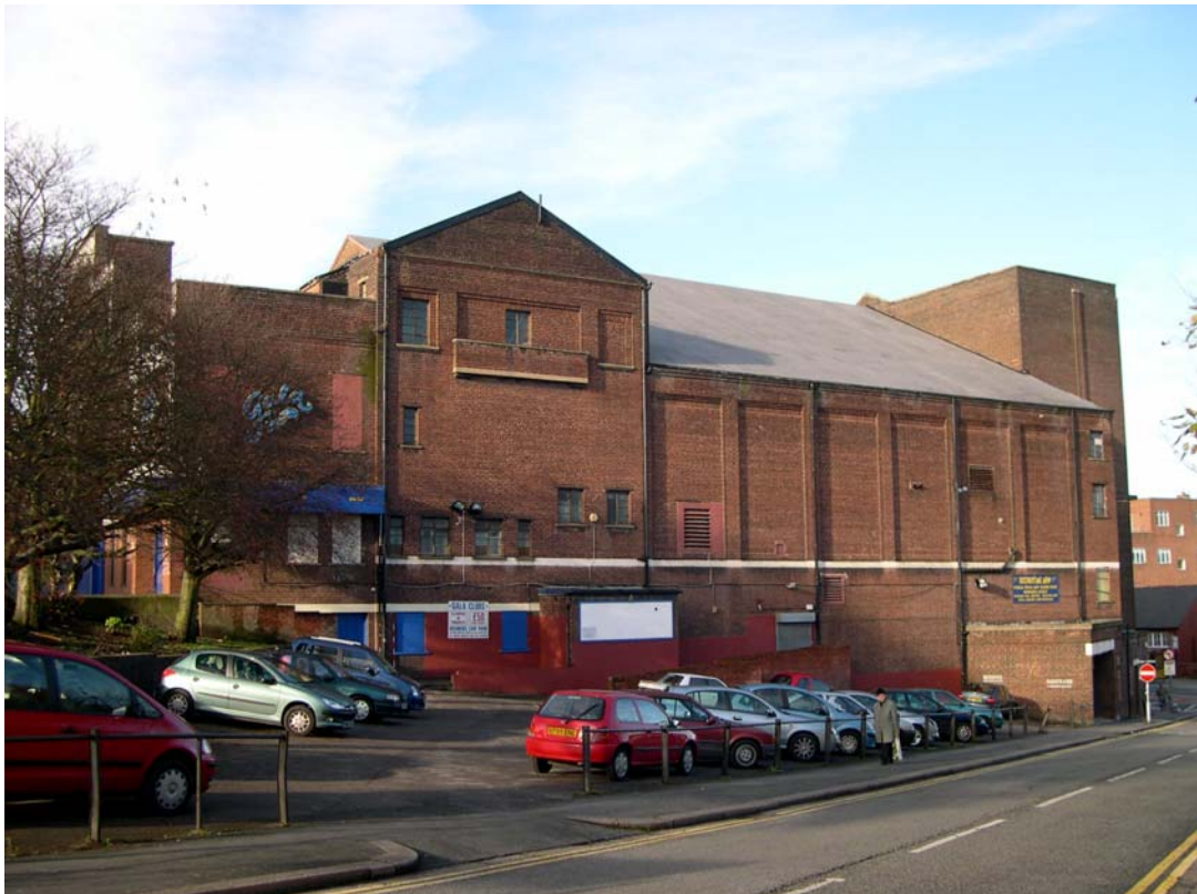
Plate 2: Eastern elevation of Gala bingo hall
