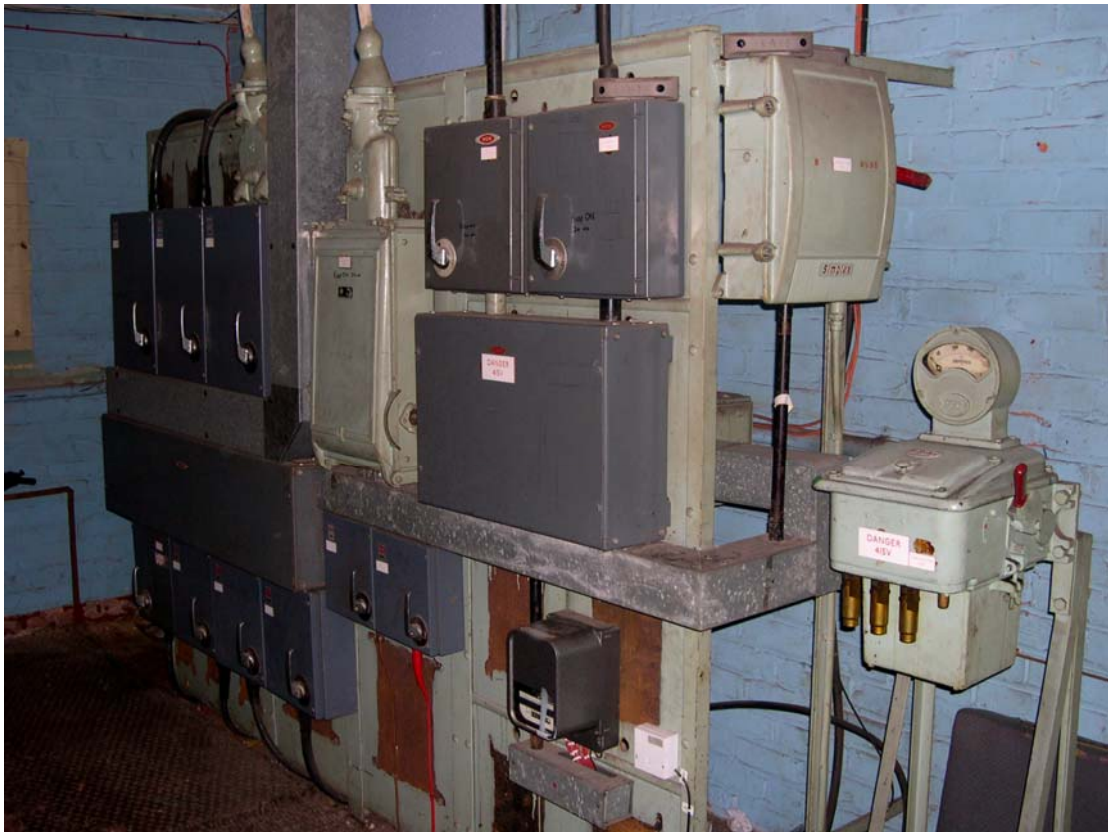
Plate 4: Fuse-boxes in outshut
