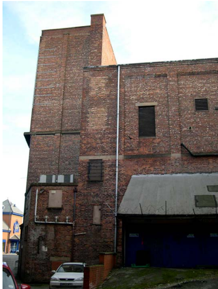
Plate 6: Boiler house and loading bay, Gala bingo hall
