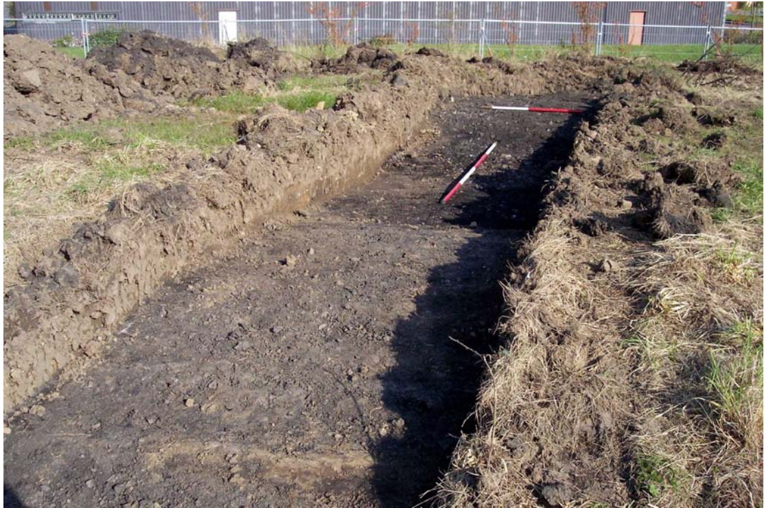
Plate 9: General view of Trench 1, looking east
