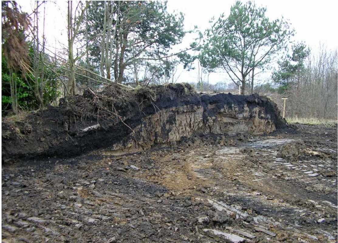
Plate 1: View of north-facing section of the embankment looking south-west, showing recent truncation
