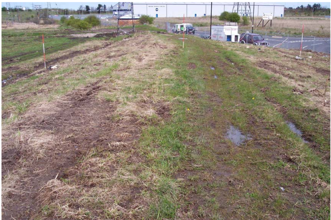
Plate 4: The north-east end of the embankment, looking north-east
