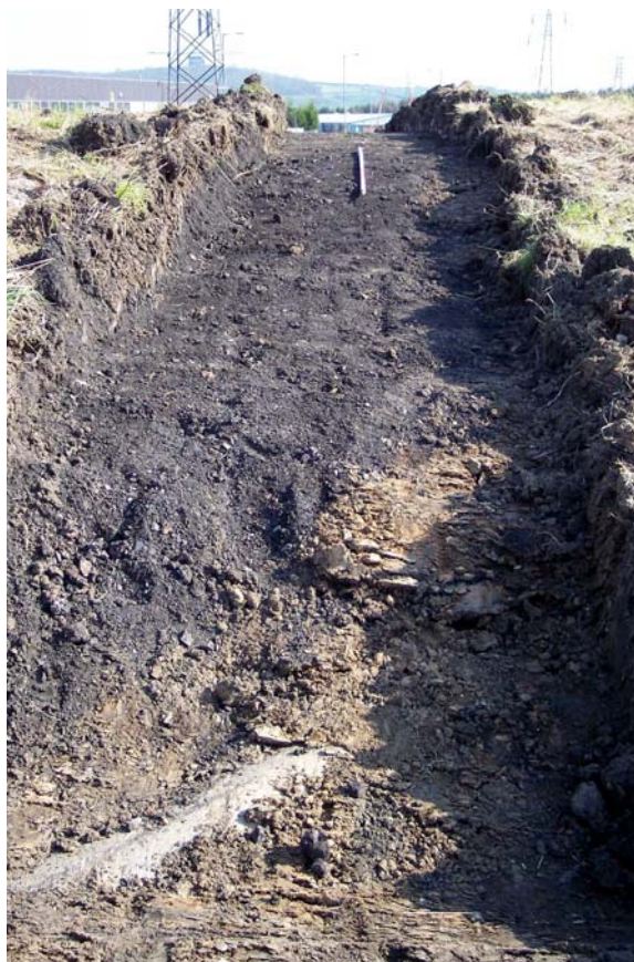
Plate 10: Trench 2, looking south, with service pipe in the foreground
