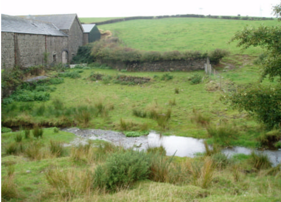
Plate 11: Scale Bank Farm retaining wall rear of farm (Site 46)
