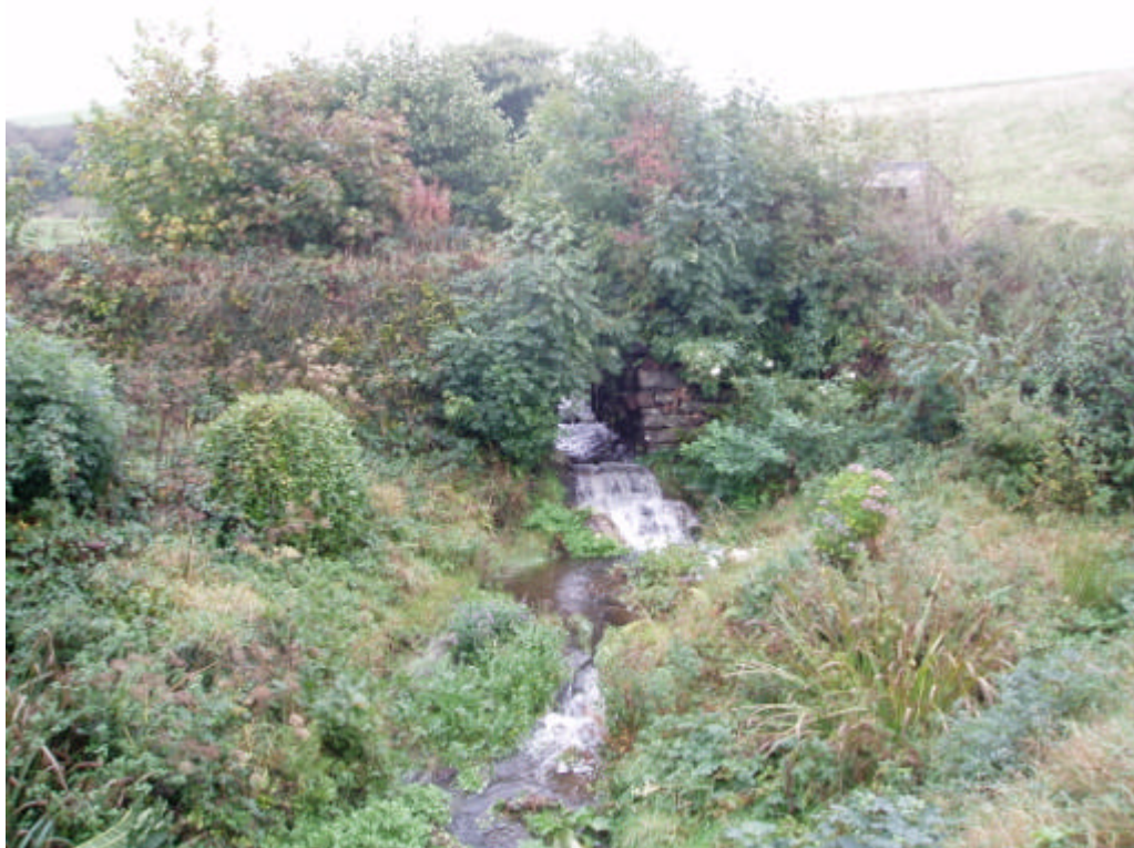
Plate: 9 Wheel Pit and sluice, Scale Bank Farm (Site 46)
