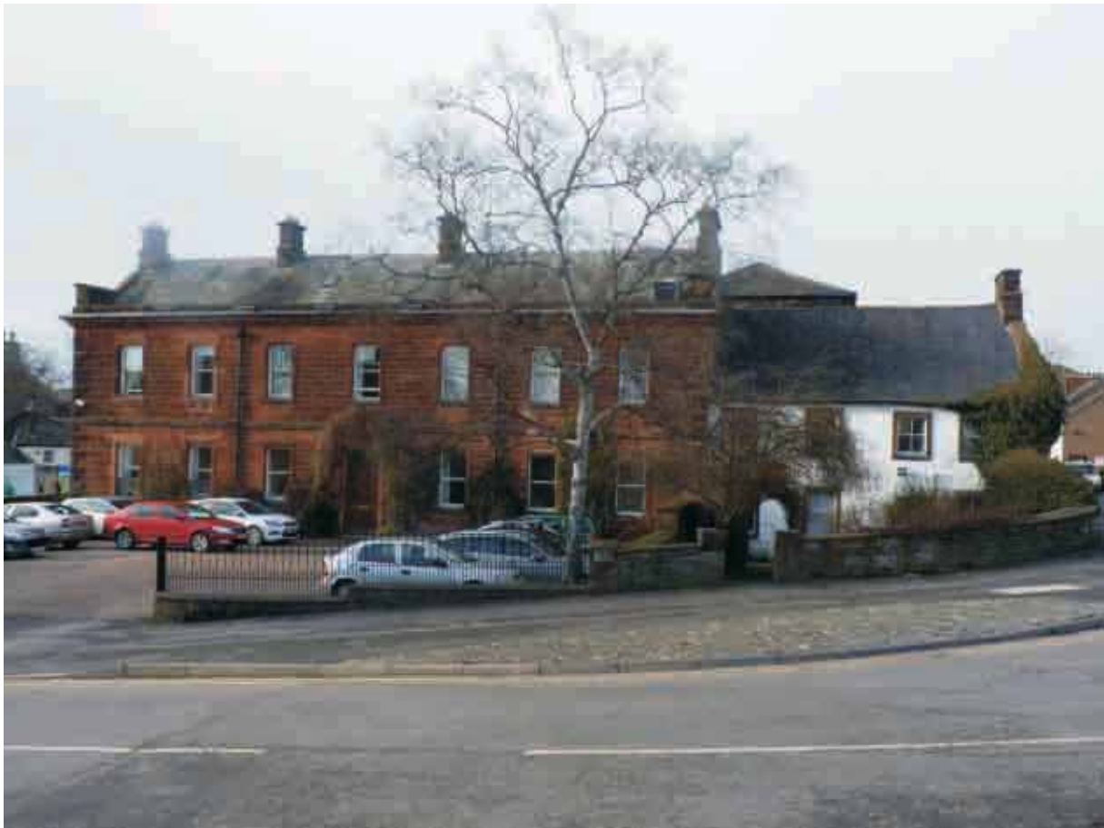
Plate 1: View looking north-west from Friargate to Hutton Hall and Masonic Hall
