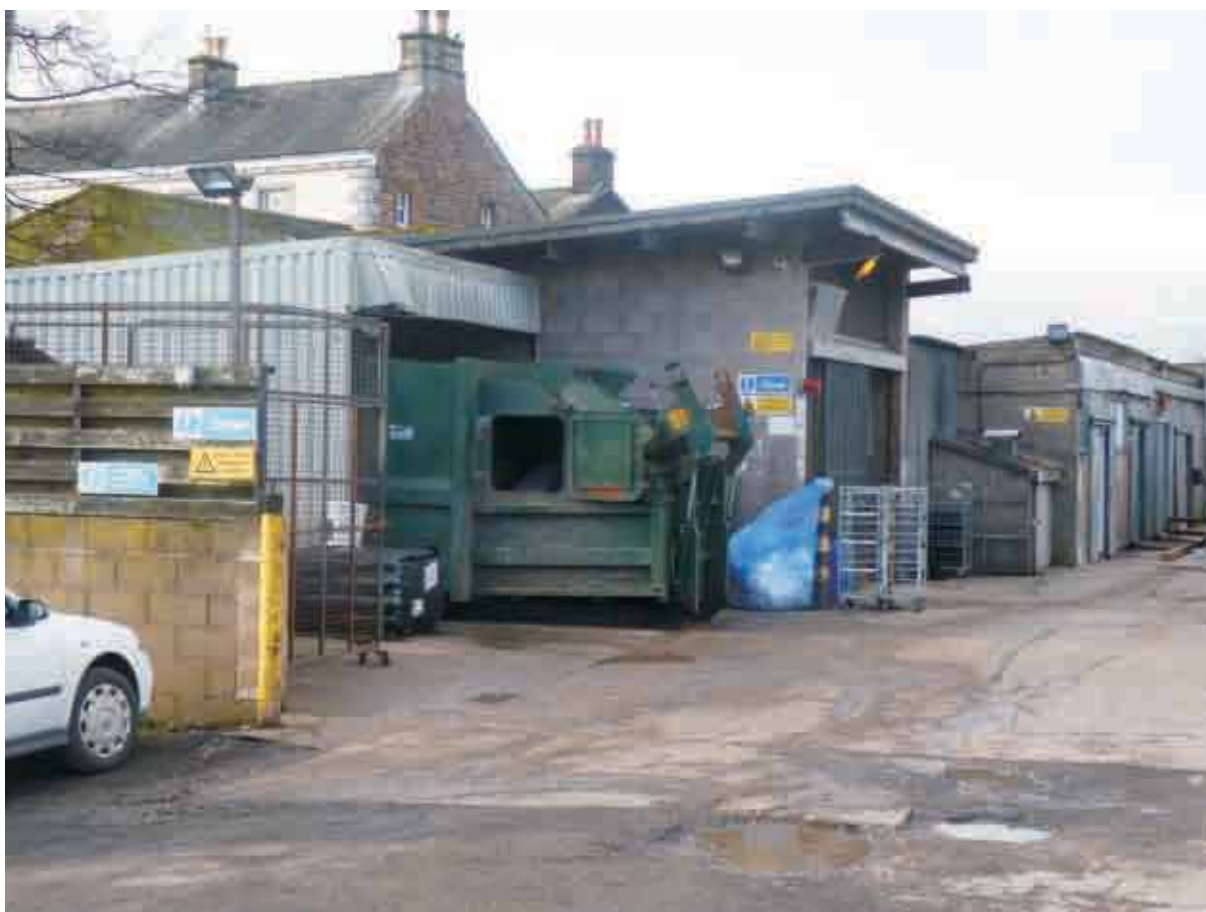
Plate 8: View looking west towards the bakery outbuildings
