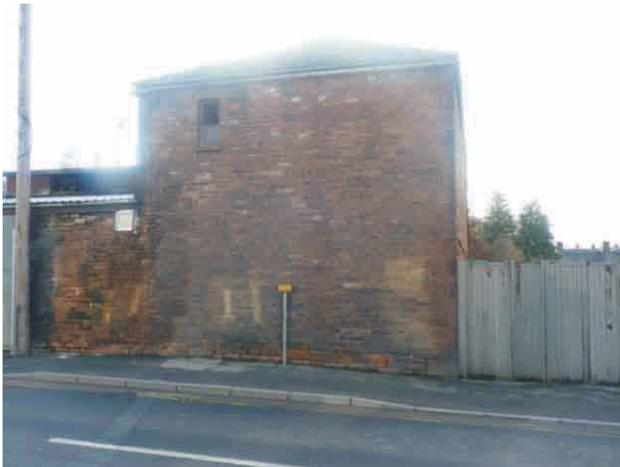
Plate 5: View looking south-west across Benson Row towards the outbuilding in the northernmost part of the development site
