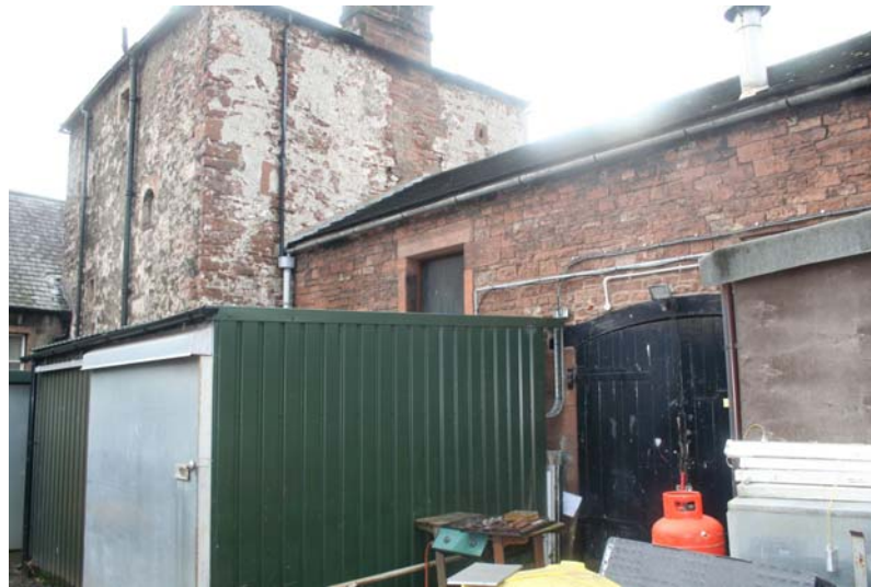
Plate 5: The former coaching house obscured by modern obstructions and clutter
