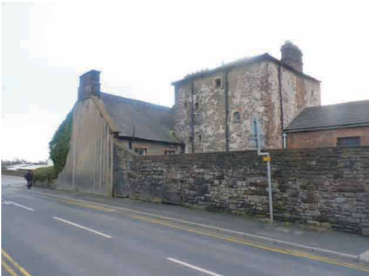
Plate 2: View looking south from Benson Row to the back of Pele Tower and Masonic Hall
