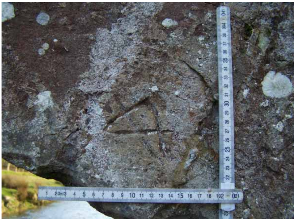
Plate 16: Low Bridge: mason's mark on possible seventeenth-century masonry on the north side of the arch
