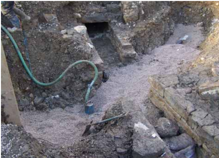
Plate 11: Construction of pipeline across the tail-race channel (SG 168)
