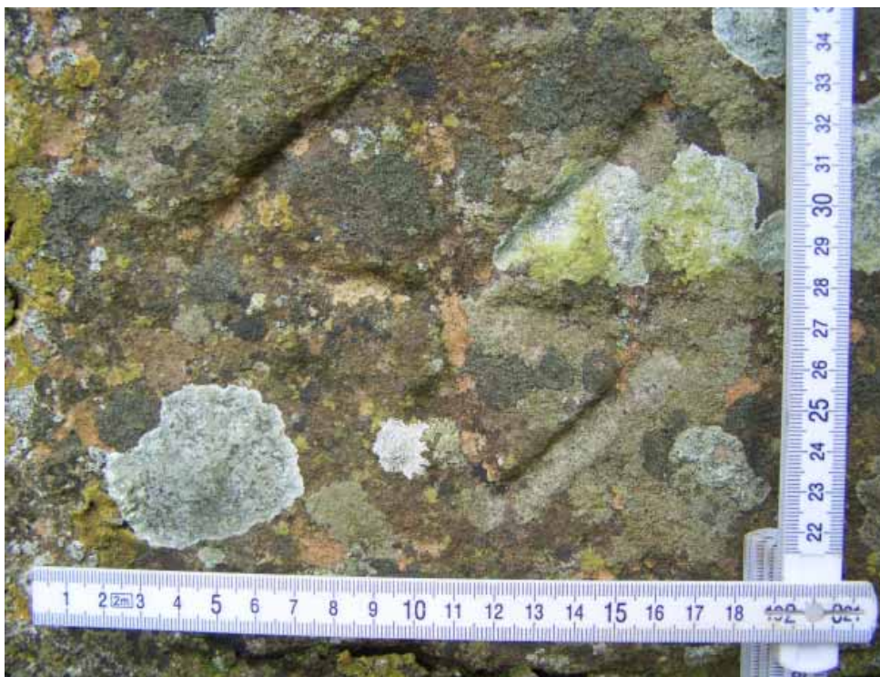
Plate 18: Low Bridge: mason's mark on mid-nineteenth-century masonry on the south side of the bridge
