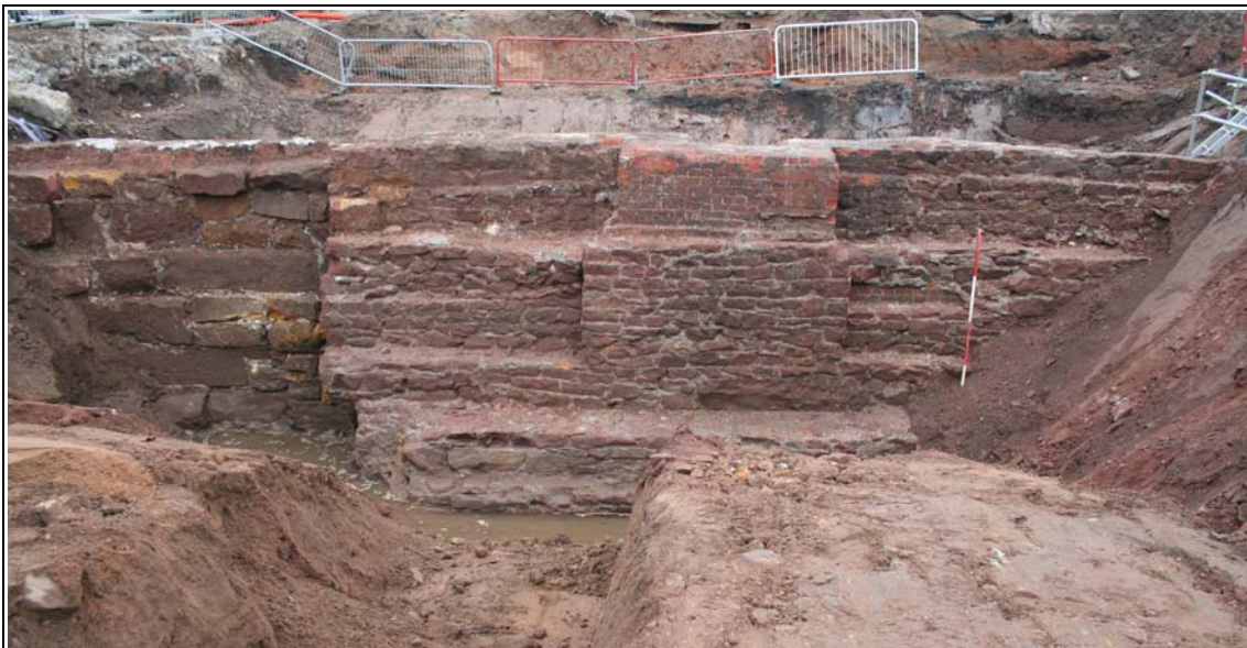
Plate 2: George's Dock Basin: the rear face of the north wall
