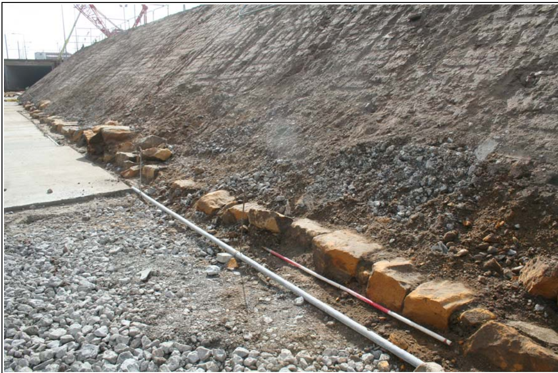
Plate 3: Remains of the sea wall between George's Dock Basin and Princes Dock
