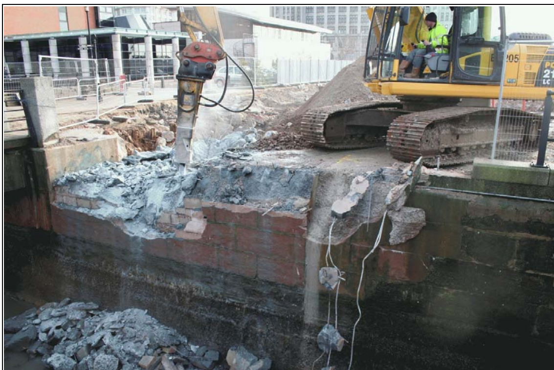
Plate 8: Princes Dock: the south wall during demolition, showing the materials used when the wall was reinstated in the 1980s
