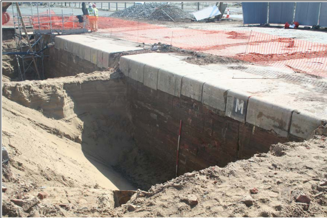
Plate 5: Trafalgar Dock: south wall
