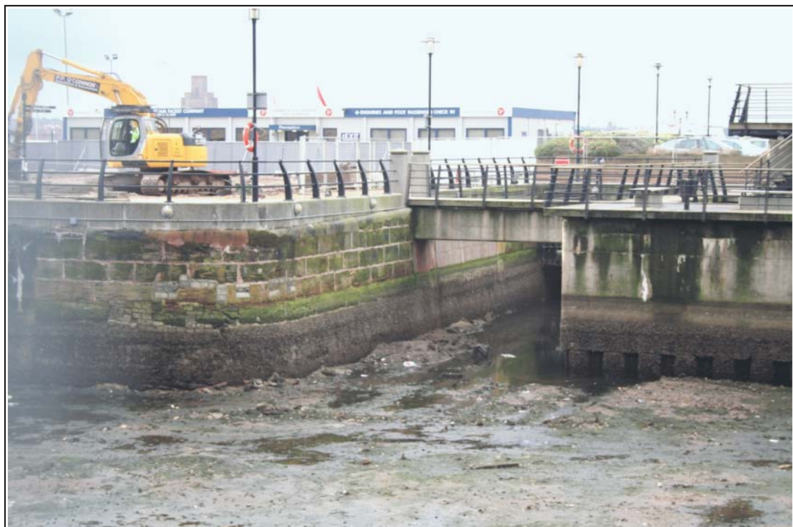
Plate 4: Princes Dock: south wall
