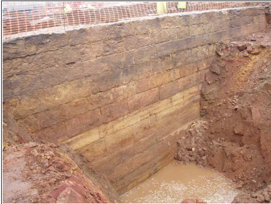
Plate 3: Sea wall 7304, from the west
