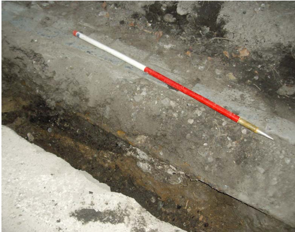
Plate 5: Existing service pipe visible in excavated trench at a depth of 0.3m
