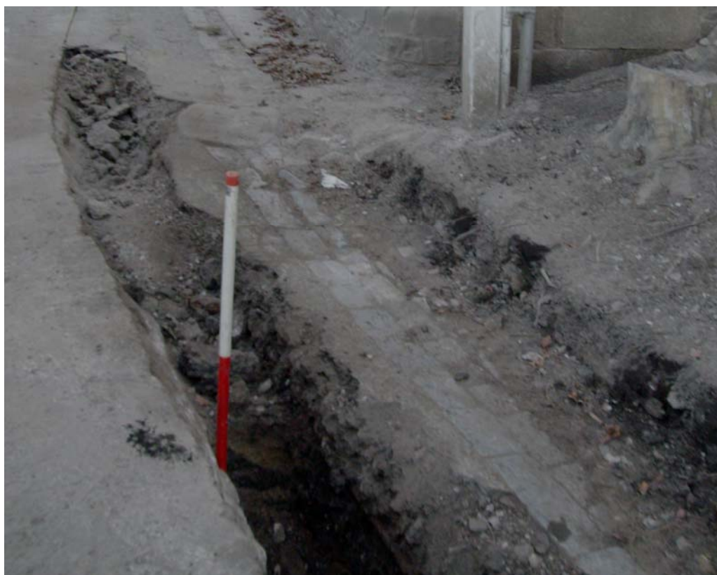
Plate 4: Excavation of the lower section of the drive approaching the gateposts
