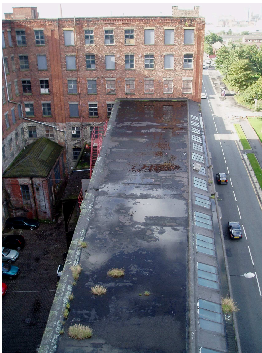
Plate 23: View along the roof of the Bradford Road block in 2005, showing inclined sky-lights
