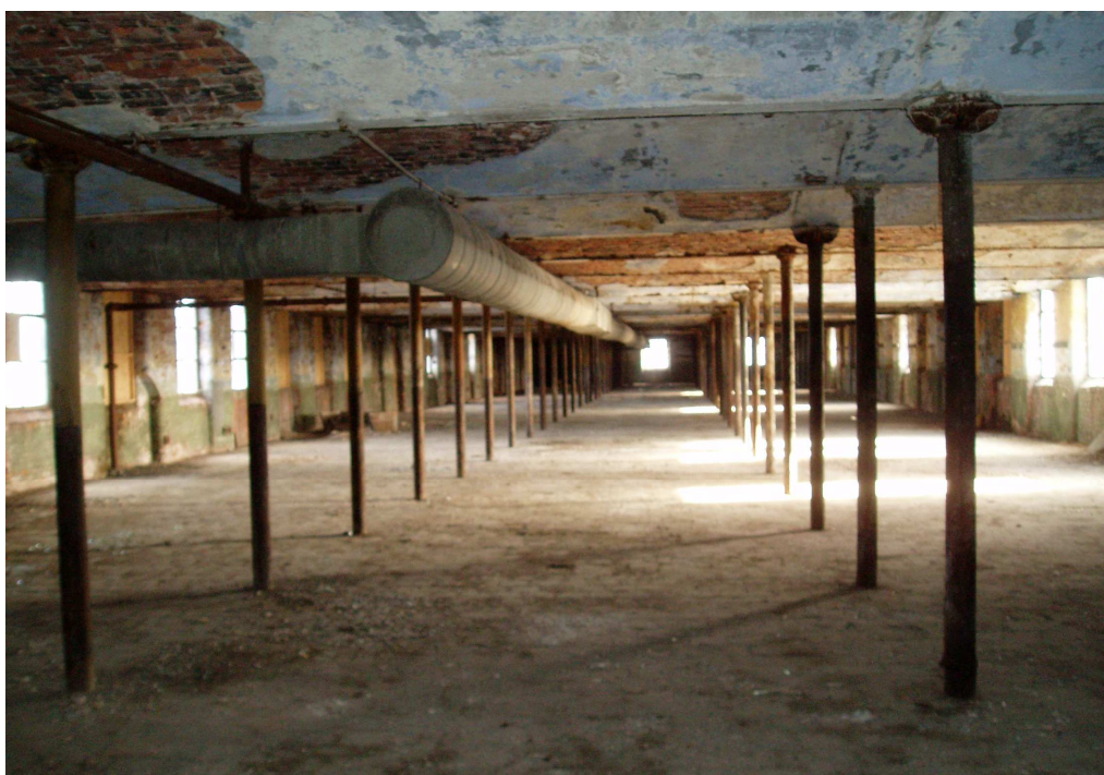
Plate 10: The top floor of the main spinning block, showing the fireproof construction
