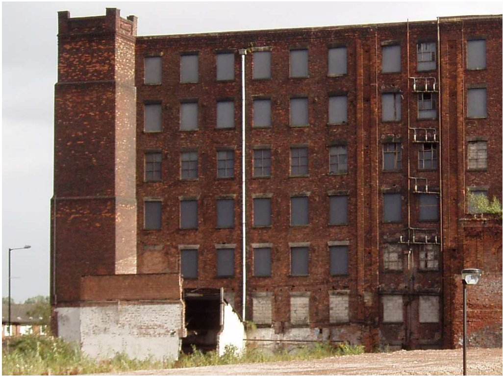
Plate 21: The west-facing elevation of the mill in 2005, showing the late nineteenth-century dust flue
