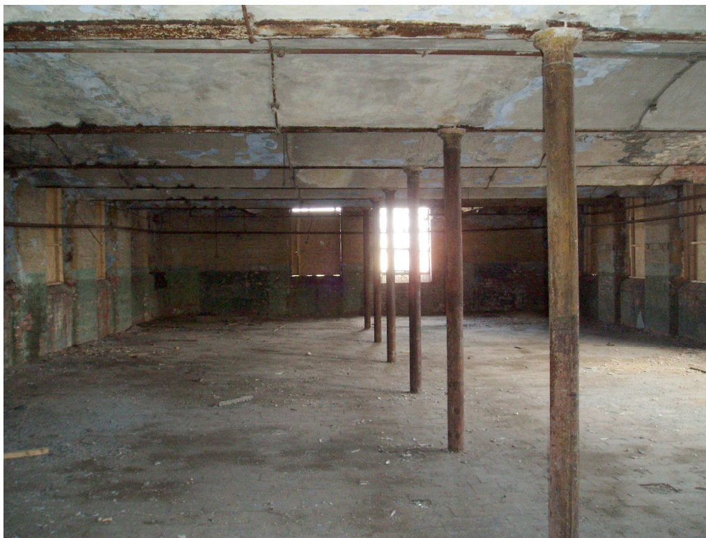
Plate 12: View across the top floor of the West Wing Mill, showing brick-vaulted ceiling and single row of cast-iron columns
