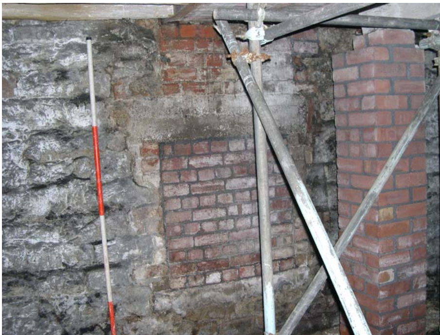
Plate 12: Blocked apertures and inserted brick pillar in Room 2, east Bridge House
