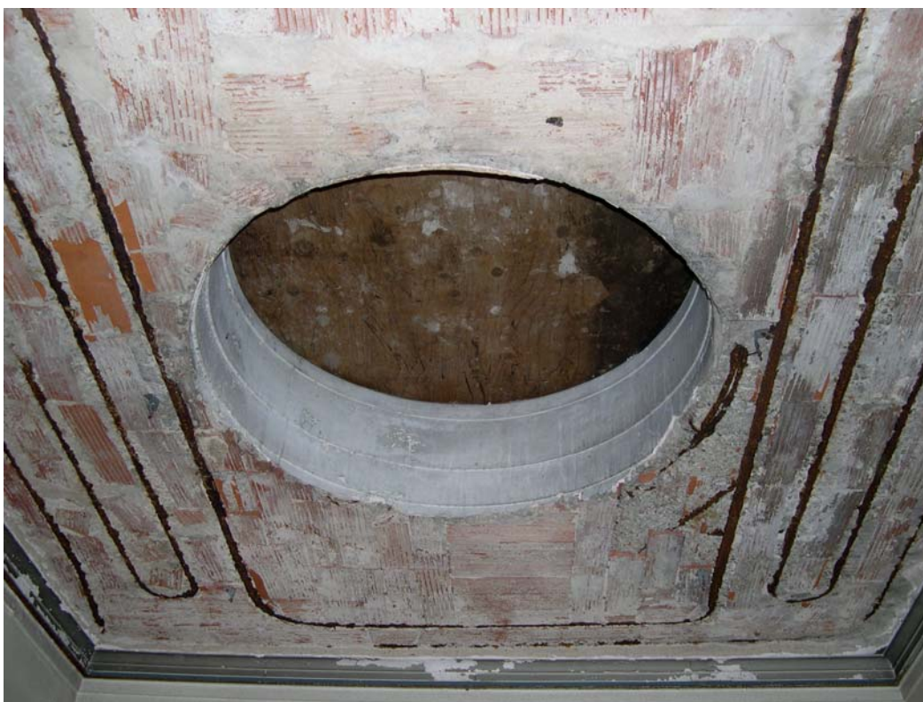
Plate 36: Example of the reinforced ceiling structure and skylight, Room 5, baths
