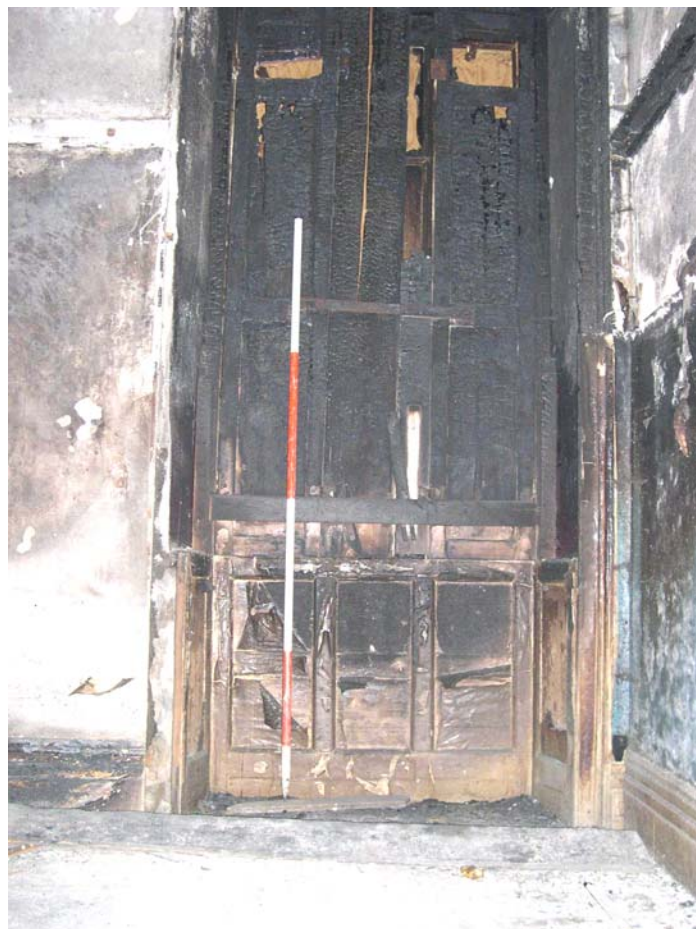
Plate 14: Window in Room 7 of east Bridge House, showing remains of badly damaged shutters and surrounds
