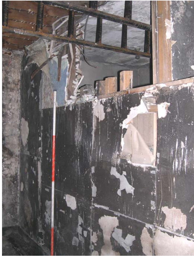
Plate 24: Junction of modern and early partitions between Rooms 14 and 18 , west Bridge House
