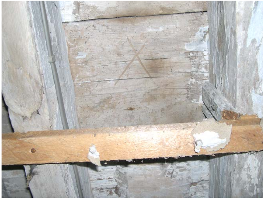
Plate 21: Timber mark in floorboards, Room 2, west Bridge House
