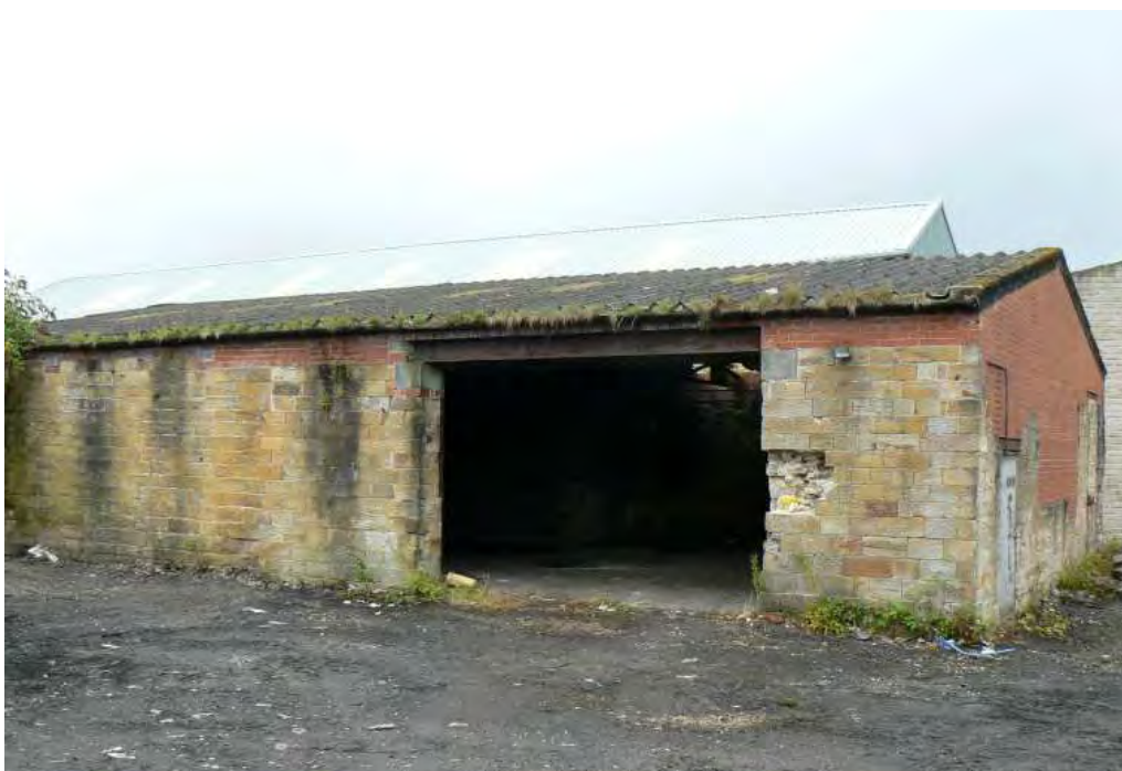
Plate 30: Surviving building in the Wiseman Street complex
