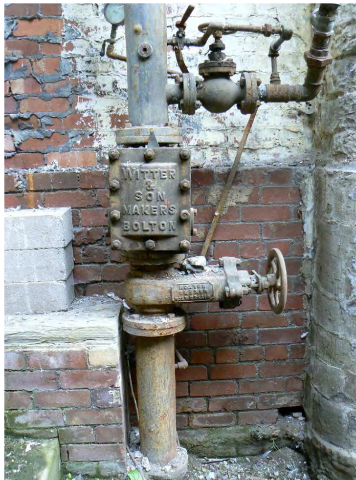
Plate 24: The main valve for the sprinkler system
