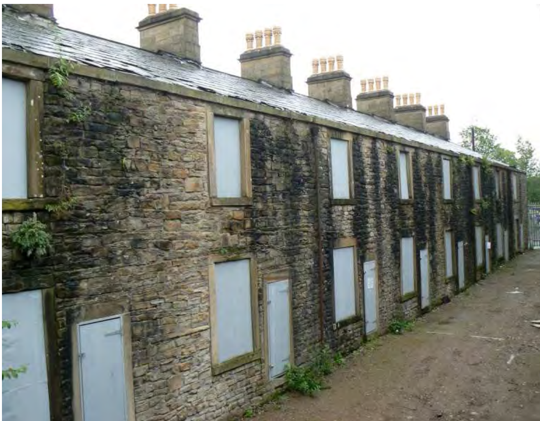
Plate 10: View along the rear of Slater's Terrace, looking towards Sandygate
