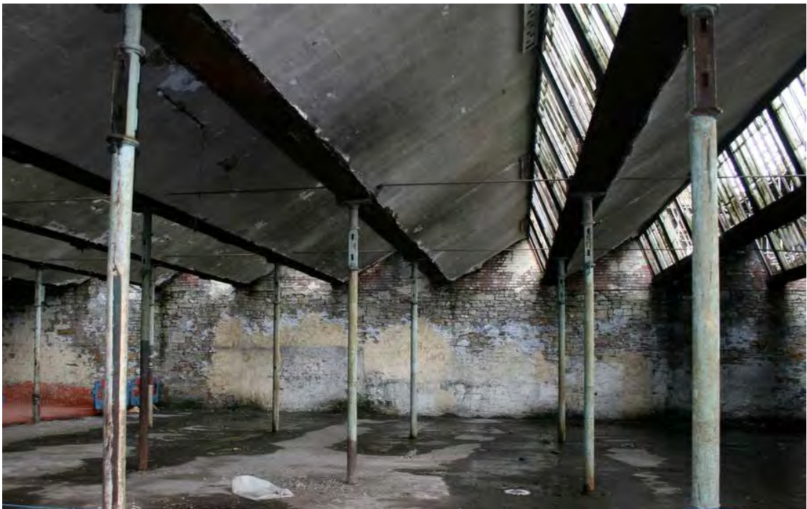
Plate 26: The interior of the weaving shed in Victoria Mill, showing the lineshaft mounting surfaces on the cast-iron columns
