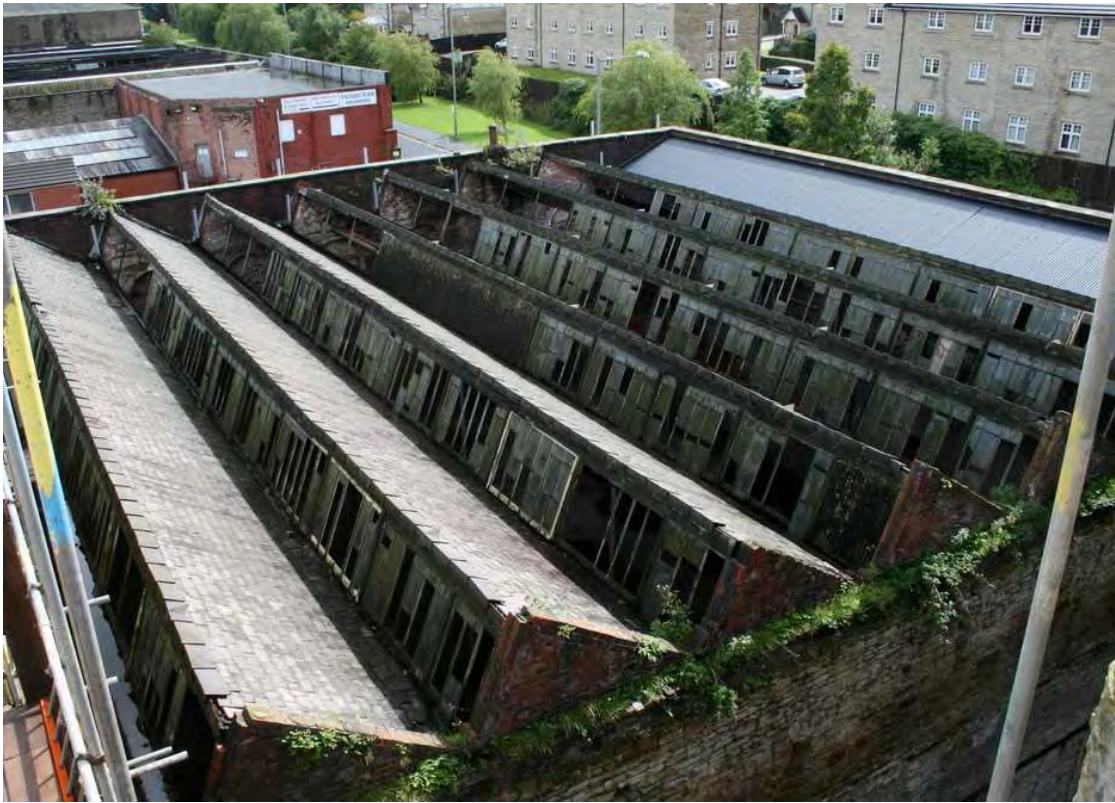
Plate 25: The first-floor weaving shed
