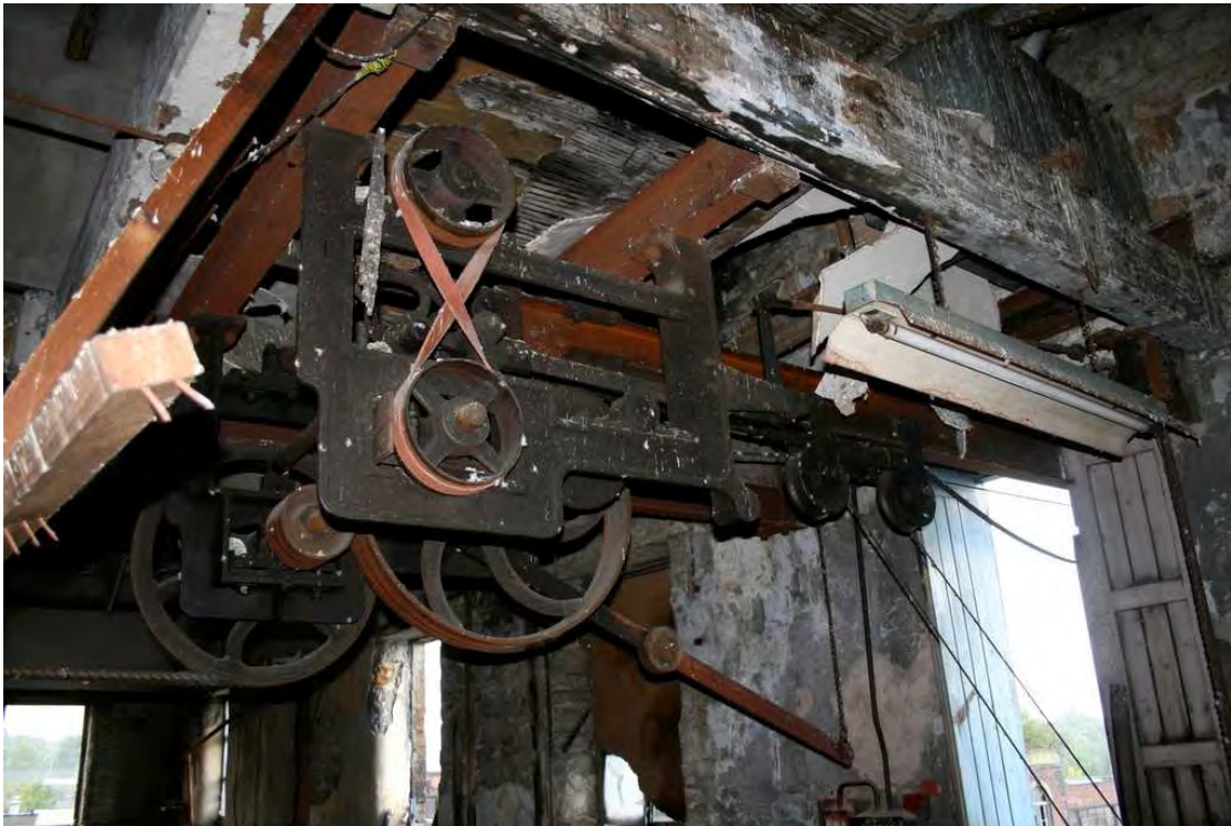
Plate 23: The original hoist, situated on the top floor of the spinning block
