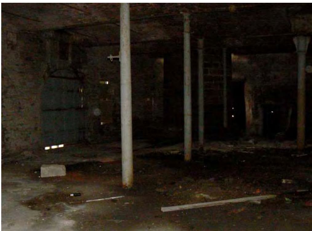
Plate 13: The ground floor of the warehouse adjacent to Slater's terrace
