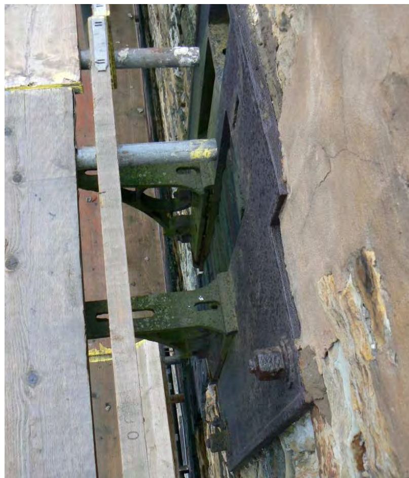
Plate 17: Cast-iron housing, probably for a vertical shaft, affixed to the north-west-facing wall of the spinning block at third-floor level
