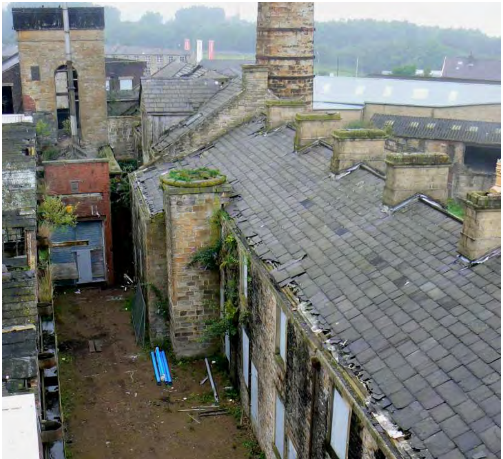
Plate 12: The rear of Slater's Terrace, abutted by the original chimney. The original boiler house was situated behind the chimney, whilst the associated engine house may have occupied the yard area in front of the late, brick-built boiler house.
