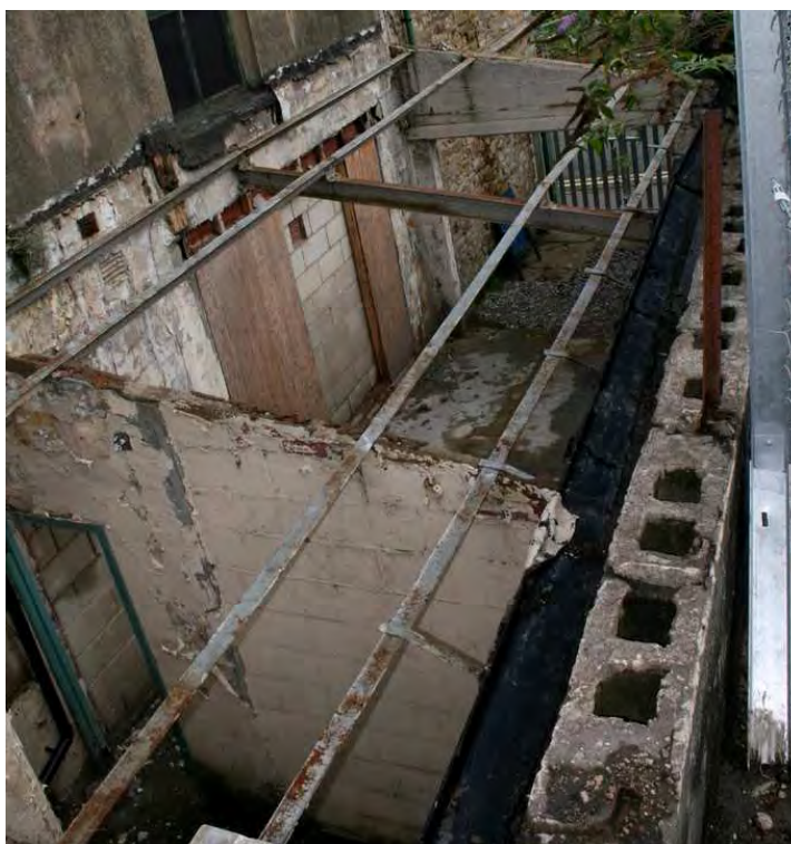
Plate 8: Clinker-block outshut to Neptune House
