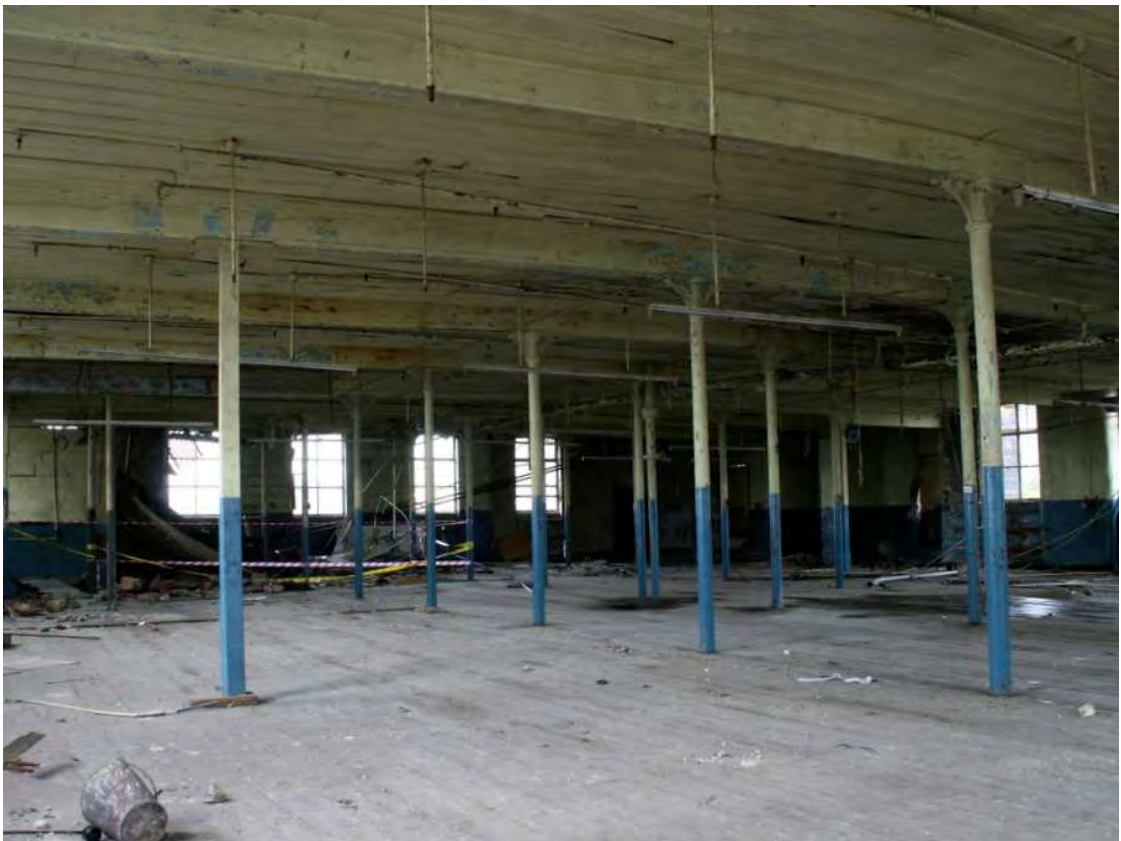
Plate 22: Second floor in the spinning block, showing density of columns and timber props
