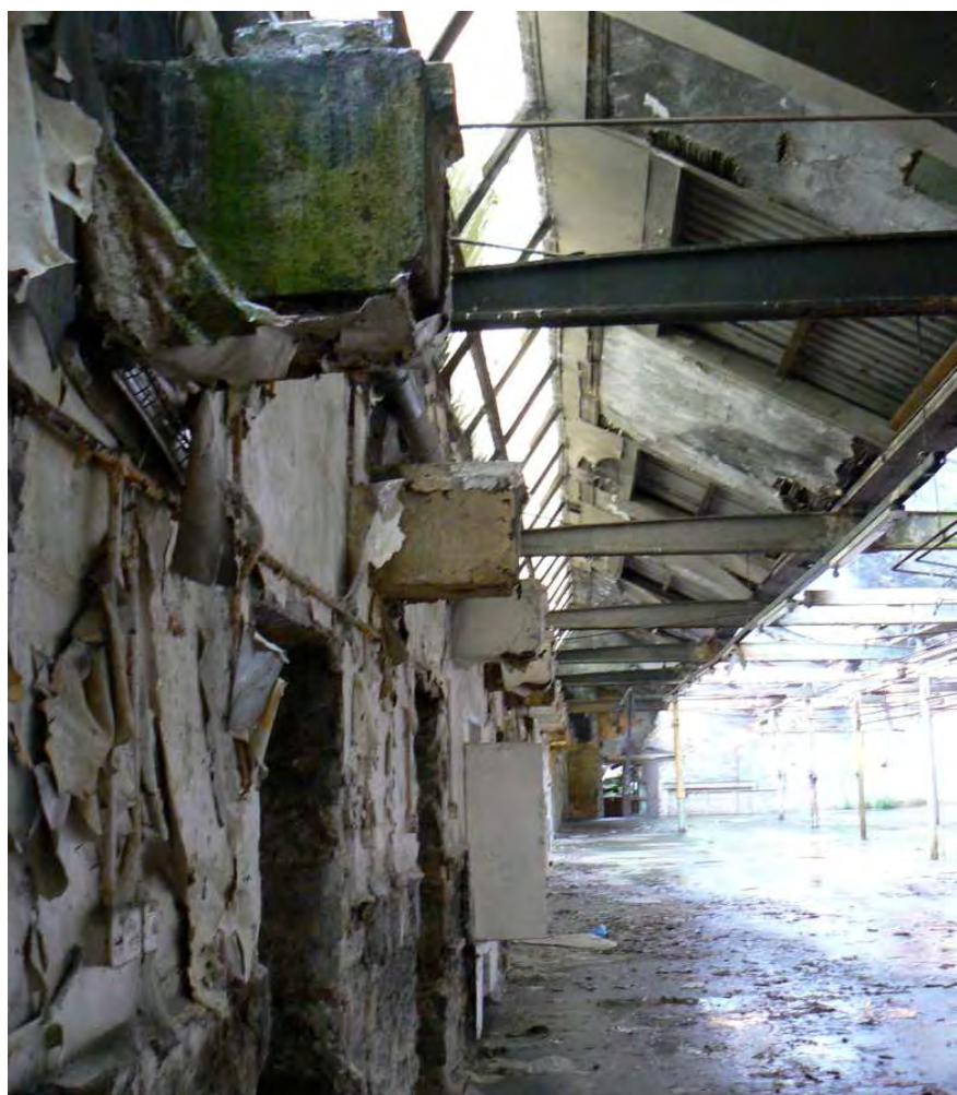
Plate 19: View across the weaving shed, showing the lineshaft bevel-gear housings
