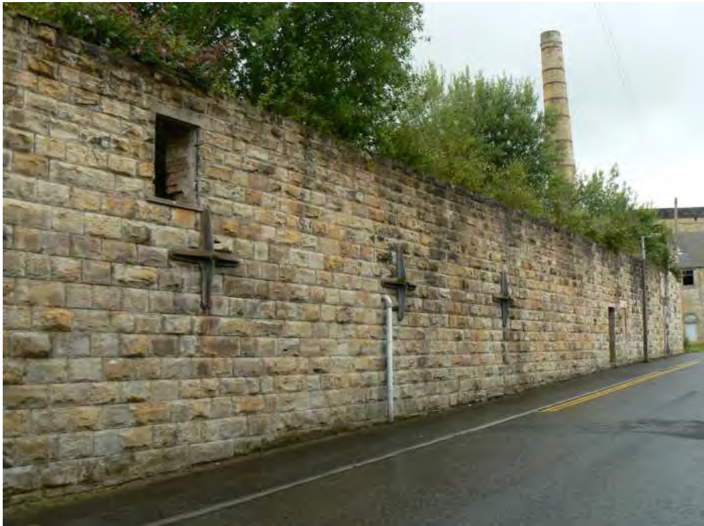
Plate 27: Surviving elements of Sandygate Shed, looking south-west along Wiseman Street
