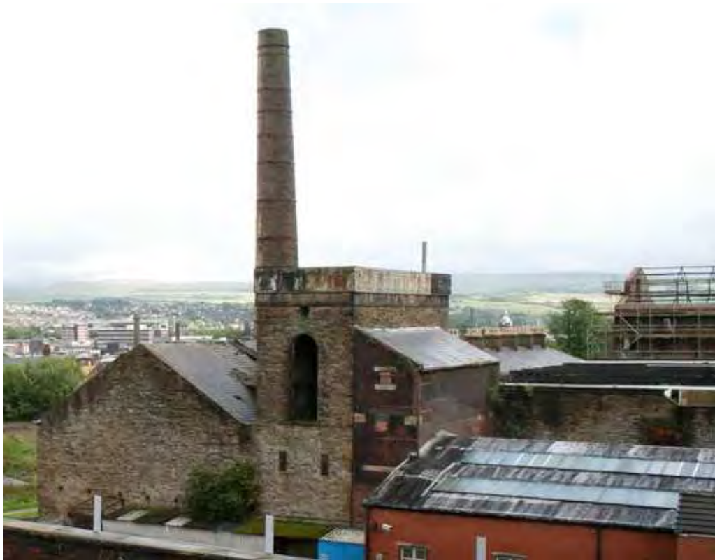
Plate 14: The north-west-facing elevation of the engine house
