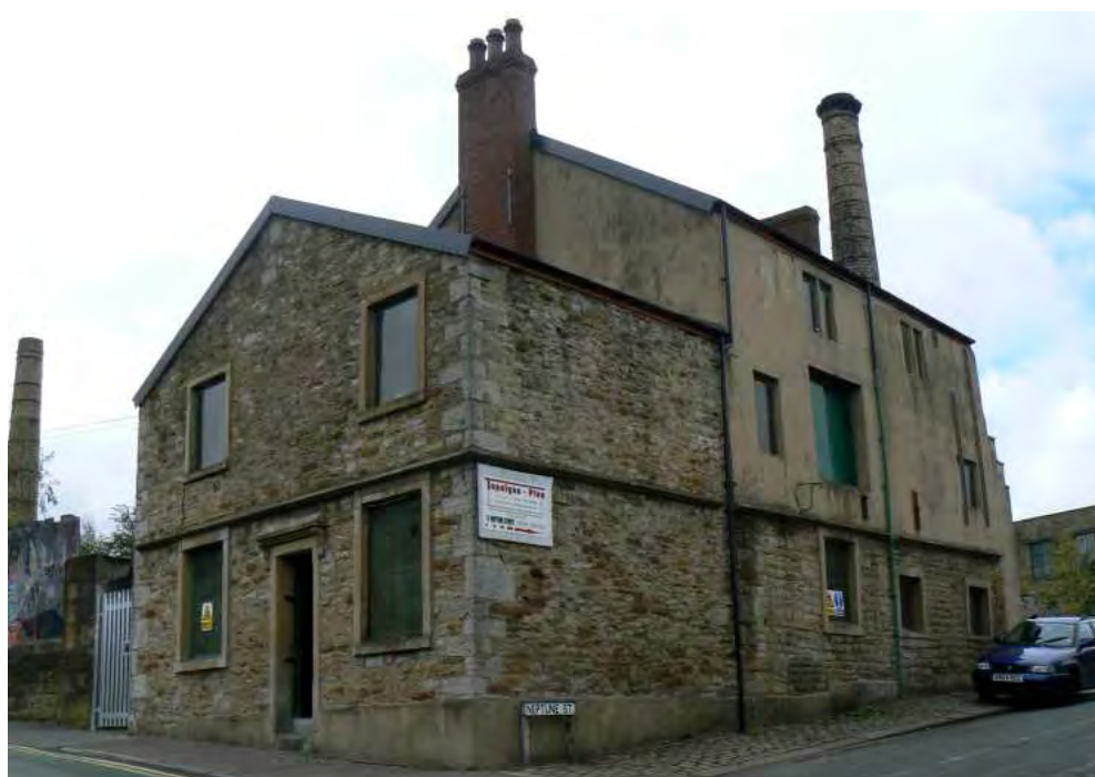
Plate 6: Neptune House, viewed from the south-west
