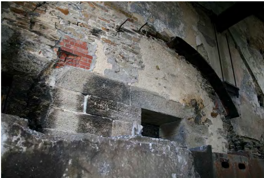
Plate 15: The flywheel guard and axle bearing in the engine house
