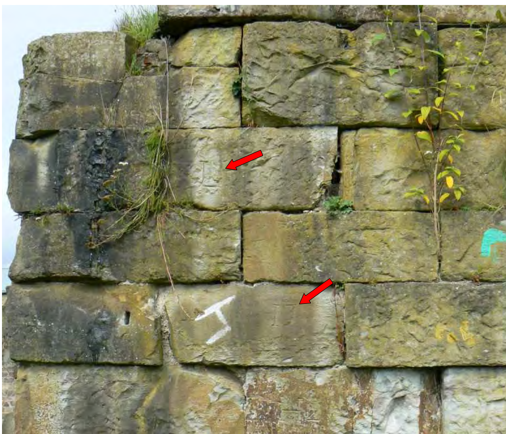
Plate 29: Engine-erector's marks in the foundation bed masonry
