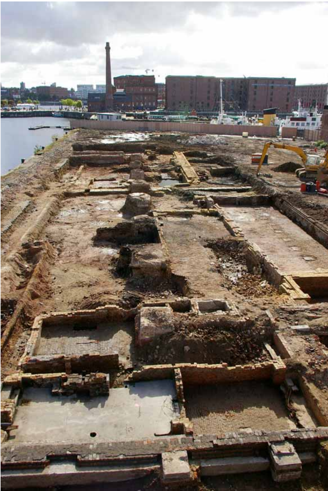
Plate 3: Warehouses at the north-west end of Area A
