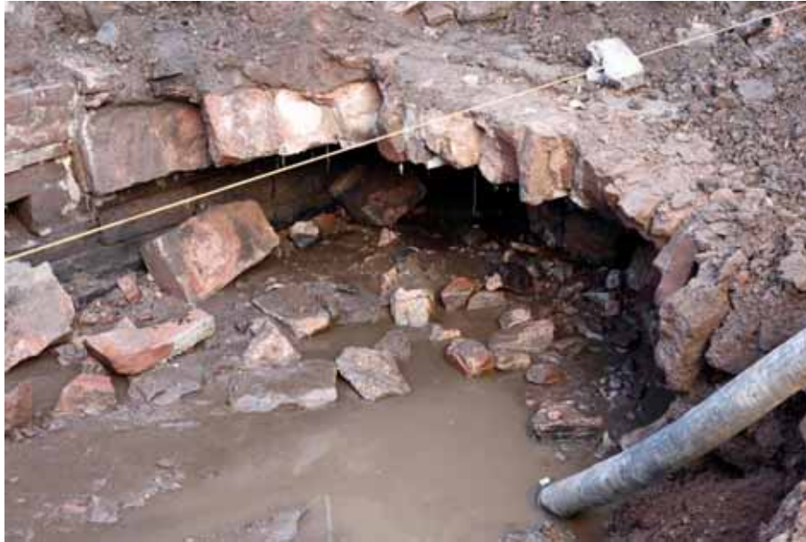
Plate 15: Excavated culvert in White House Gardens
