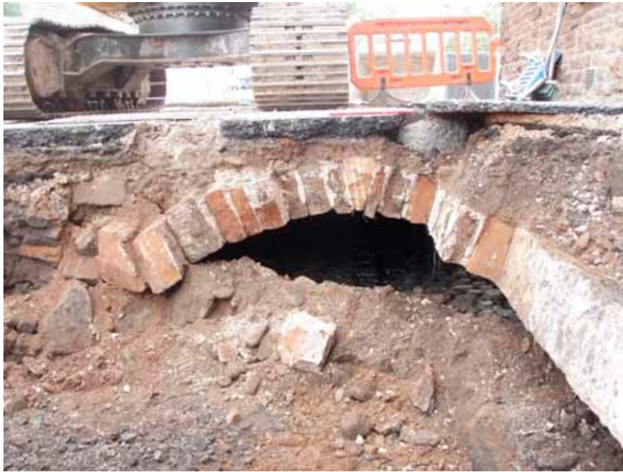
Plate 8: Excavated culvert at Friargate
