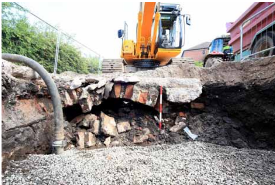
Plate 11: Excavated culvert at Somerfield Car Park
