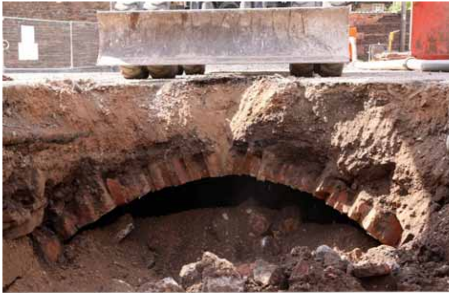
Plate 5: Excavated culvert at the rear of the Mansion House
