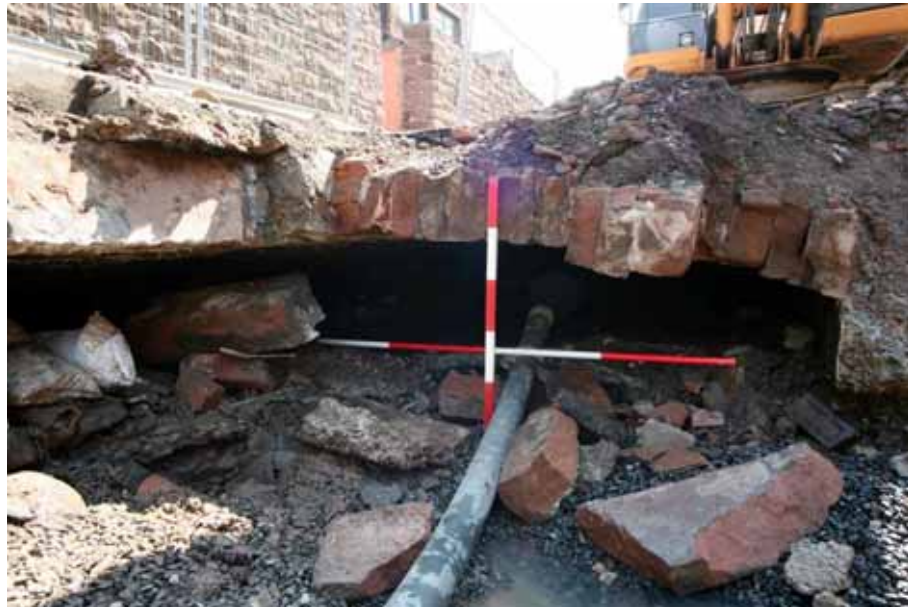
Plate 2: Excavated culvert below Watson Terrace
