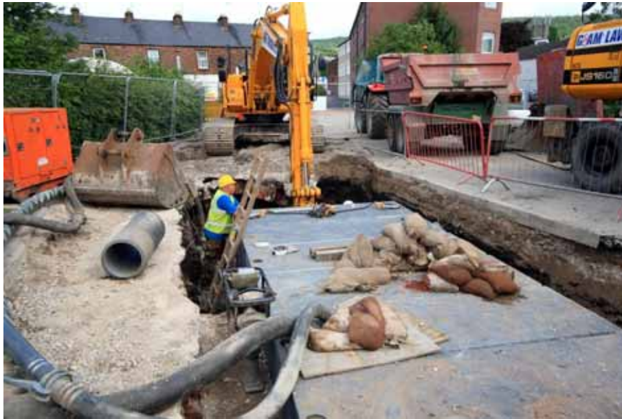
Plate 10: Excavation of the culvert at Somerfield Car Park
