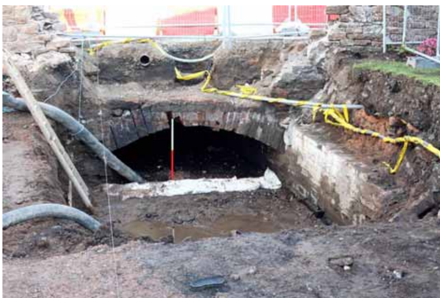
Plate 13: Excavation of the culvert at Roper Street to White House Gardens
