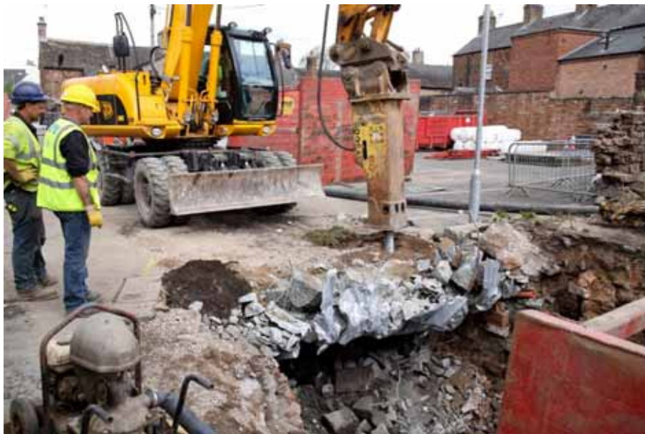
Plate 4: Excavation of culvert at the rear of The Mansion House
