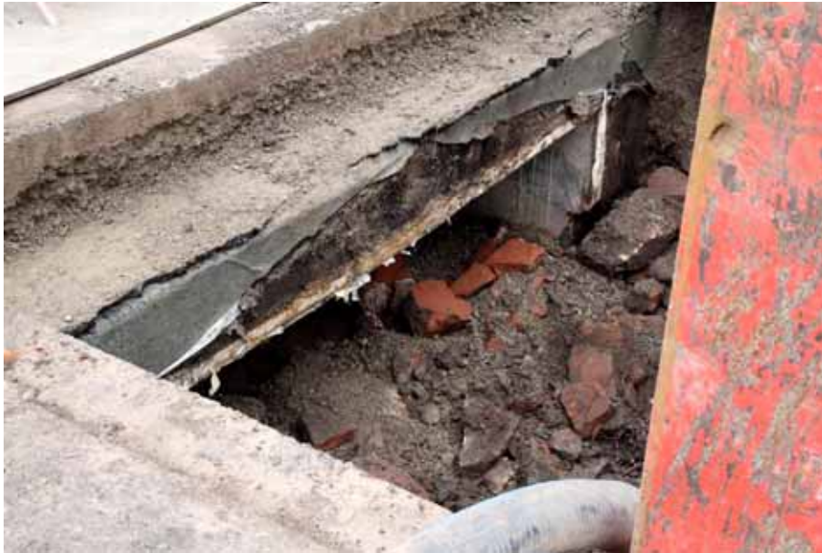
Plate 7: Excavated culvert at the front of the Mansion House
