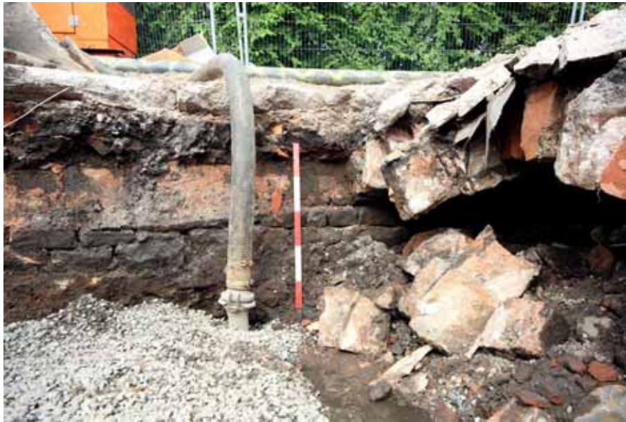
Plate 12: Imposts of the excavated culvert at Somerfield Car Park
