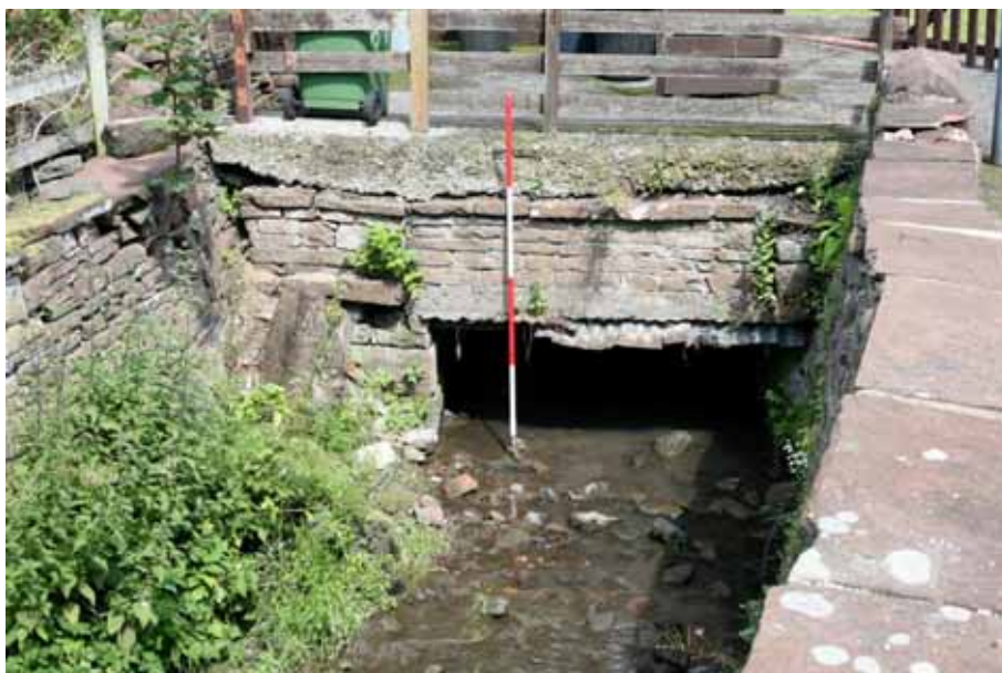
Plate 16: Thacka Beck exiting from the end of the culvert in White House Gardens
