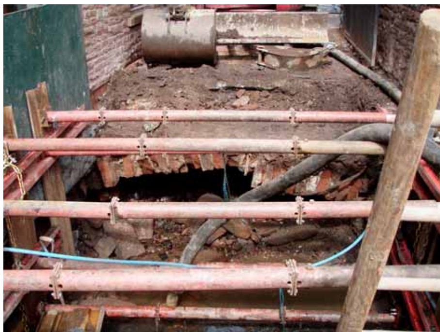
Plate 3: Excavated Culvert in Sandgate
