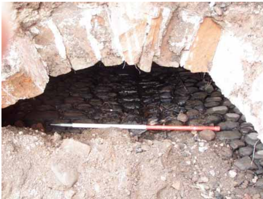
Plate 9: Floor of the excavated culvert at Friargate
