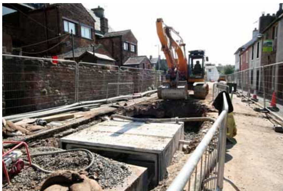
Plate 1: Excavation of the culvert in Watson Terrace
