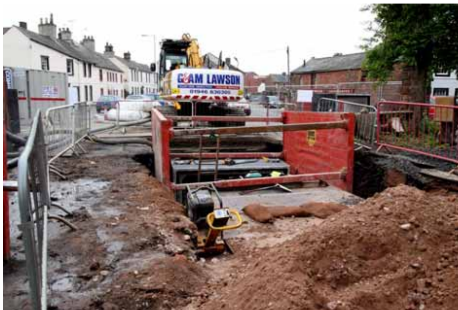
Plate 6: Excavation of culvert at the front of the Mansion House
