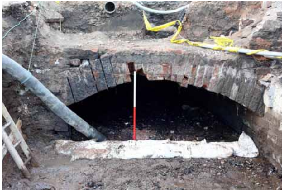
Plate 14: Excavated culvert passing below Roper Street
