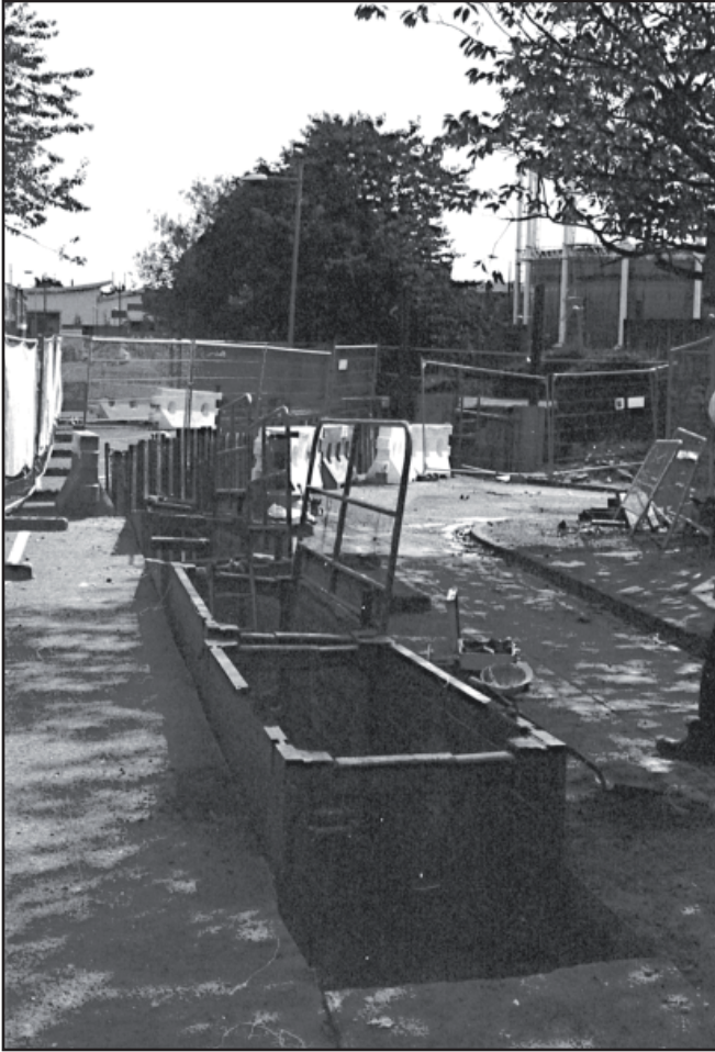
Plate 1: East facing view of the pipe trench
