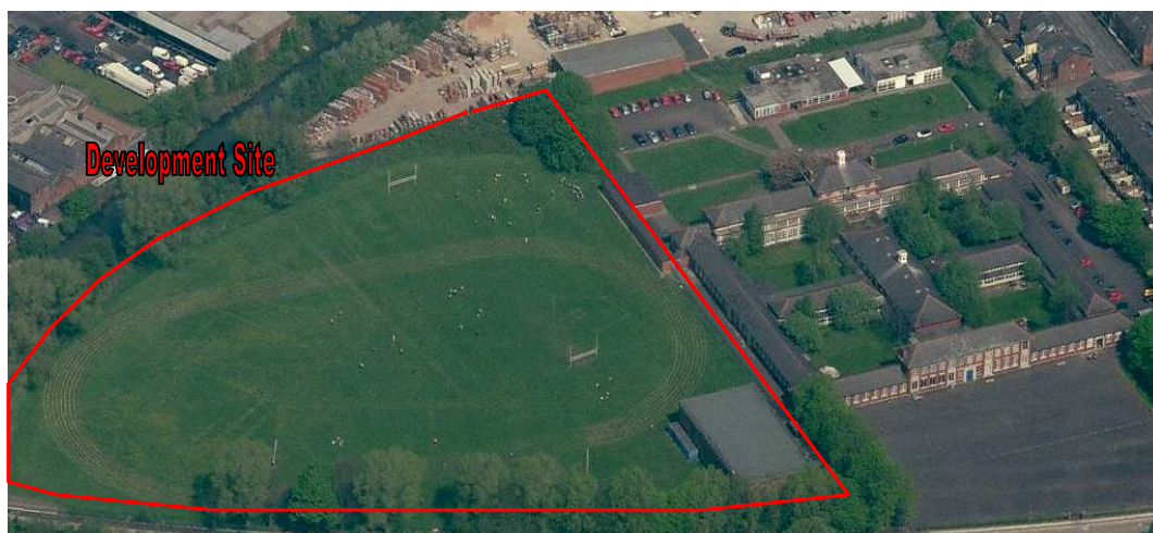
Plate 1: Recent aerial view of the proposed development site
