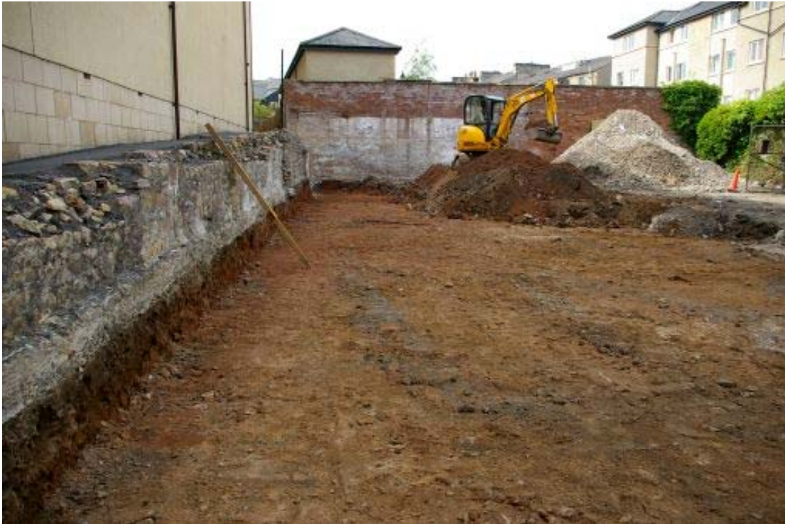
Plate 7: Working shot during reduction for raft base; facing south
