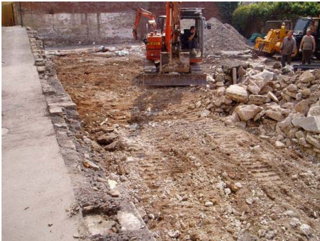
Plate 6: Working shot during removal of concrete; facing south-west
