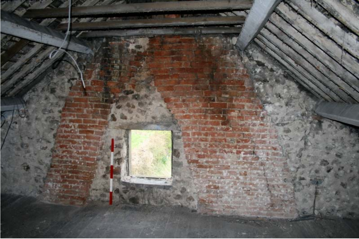
Plate 29: Raking flues, Room S2
