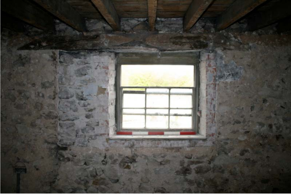
Plate 19: Remodelled window, east wall, Room F3
