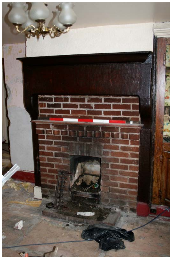
Plate 4: Fireplace in north-eastern part of Room G1
