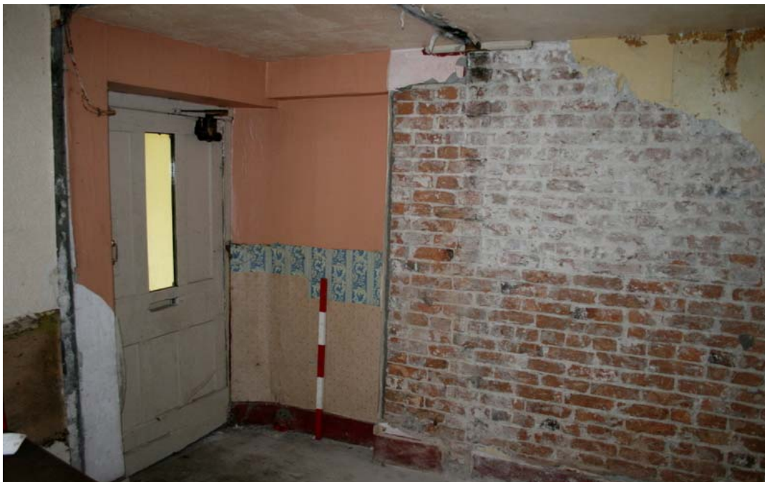
Plate 3: Door rebate and brick partition, Room G1
