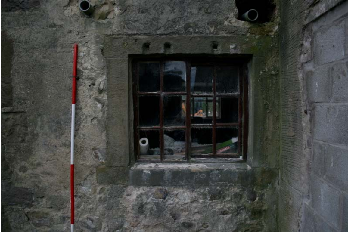
Plate 7: Horizontal sash window in north-western part of Room G1
