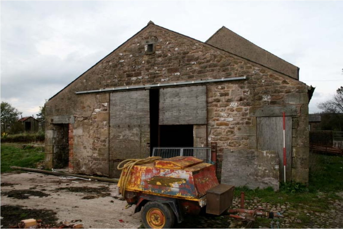
Plate 41: South elevation of cowhouse
