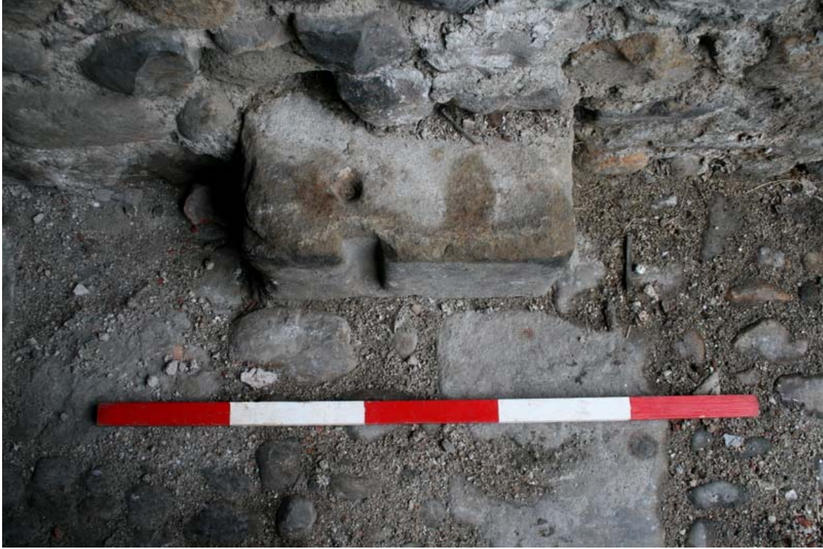
Plate 37: Sandstone pad for barn doors and winnowing boards
