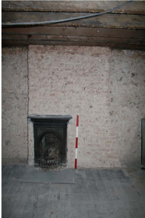
Plate 21: Fireplace, Room F3
