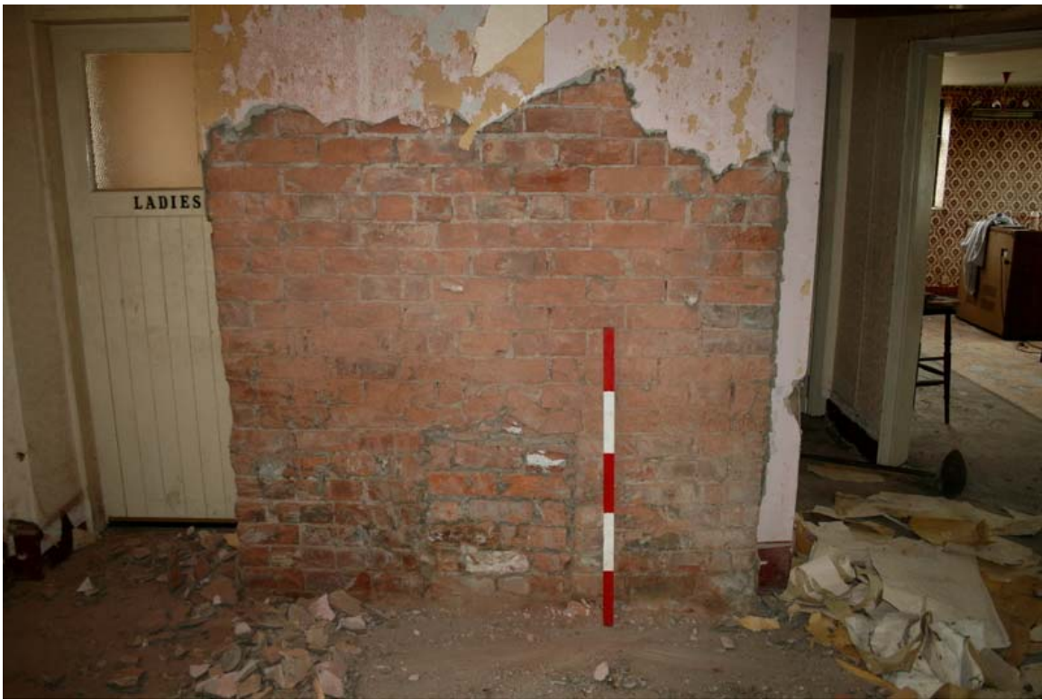
Plate 6: Blocked fireplace in north-western part of Room G1
