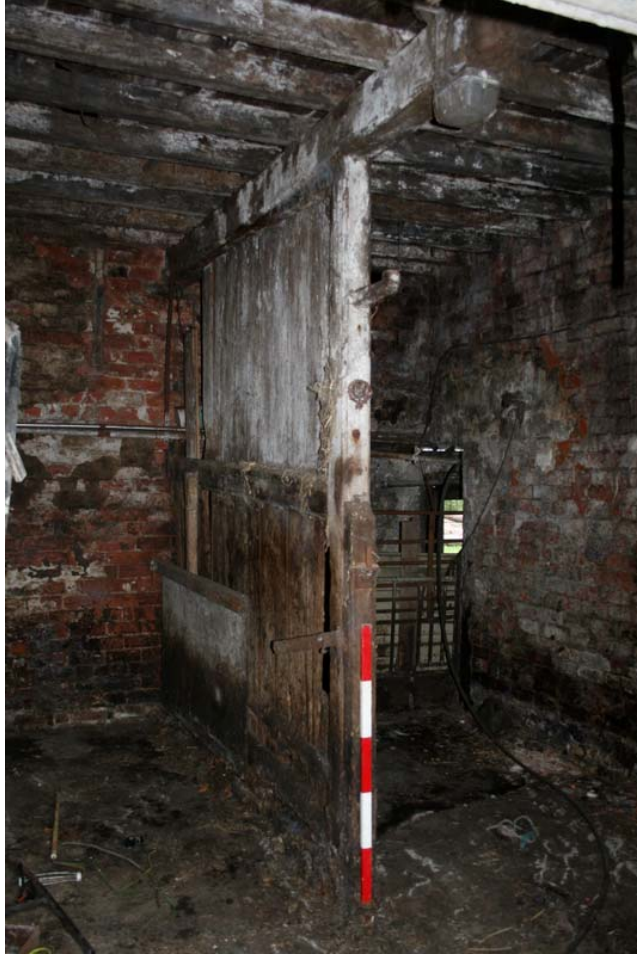
Plate 46: Timber stable stalling, hayloft
