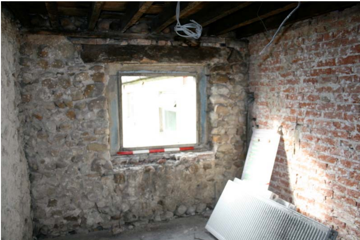
Plate 24: Original window aperture, Room F5
