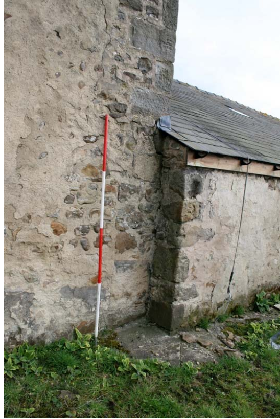
Plate 39: Junction of threshing barn and cowhouse
