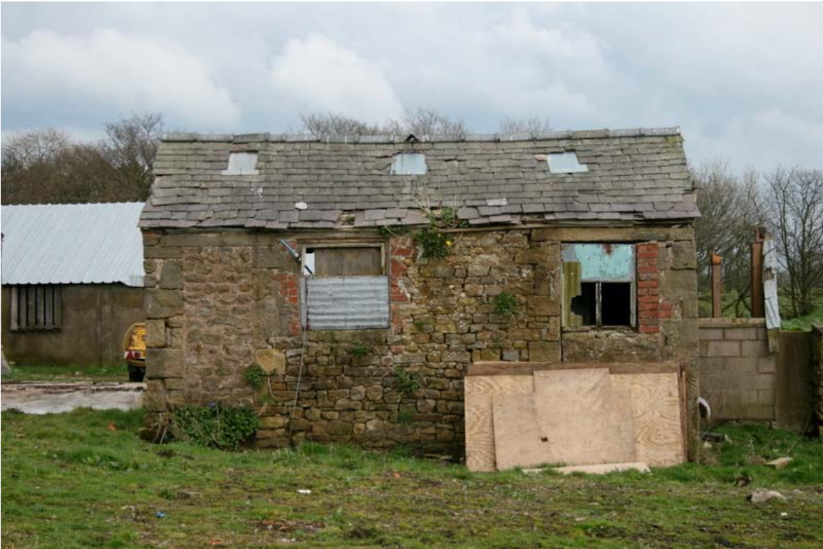
Plate 48: Western elevation of store
