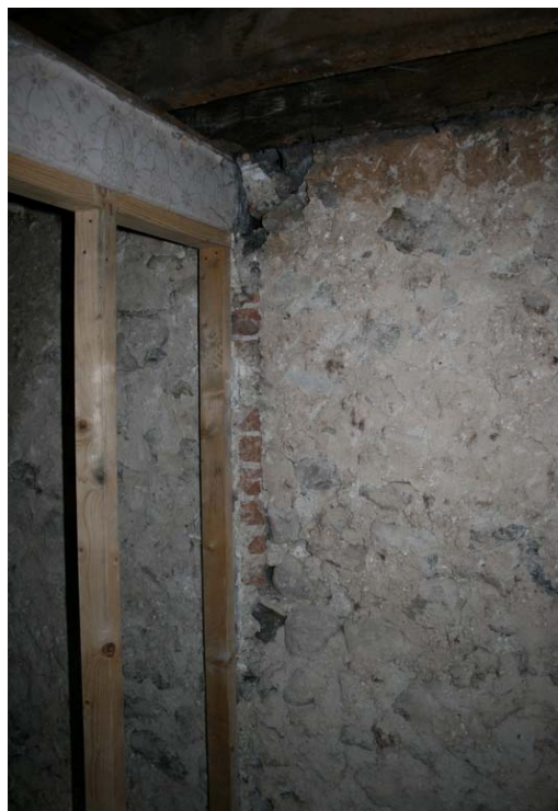
Plate 18: Wall scar of original brick partition, Room F3
