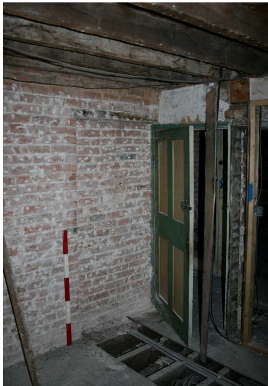
Plate 22: Door rebate, Room F3
