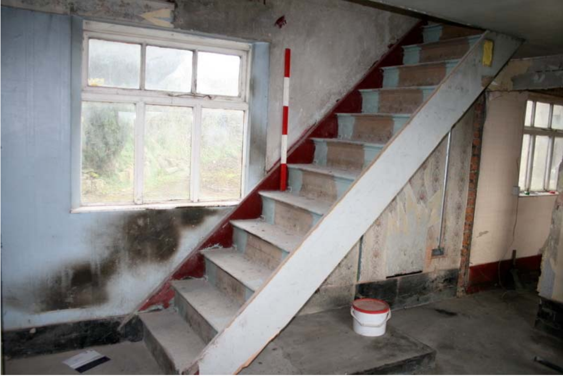
Plate 13: Extant stair in Room G4
