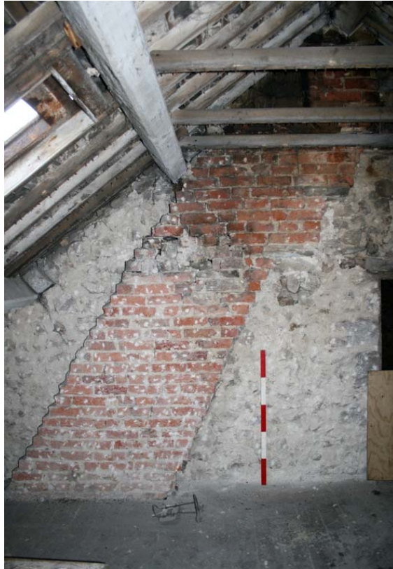
Plate 31: Raking flue with sandstone pads, Room S3
