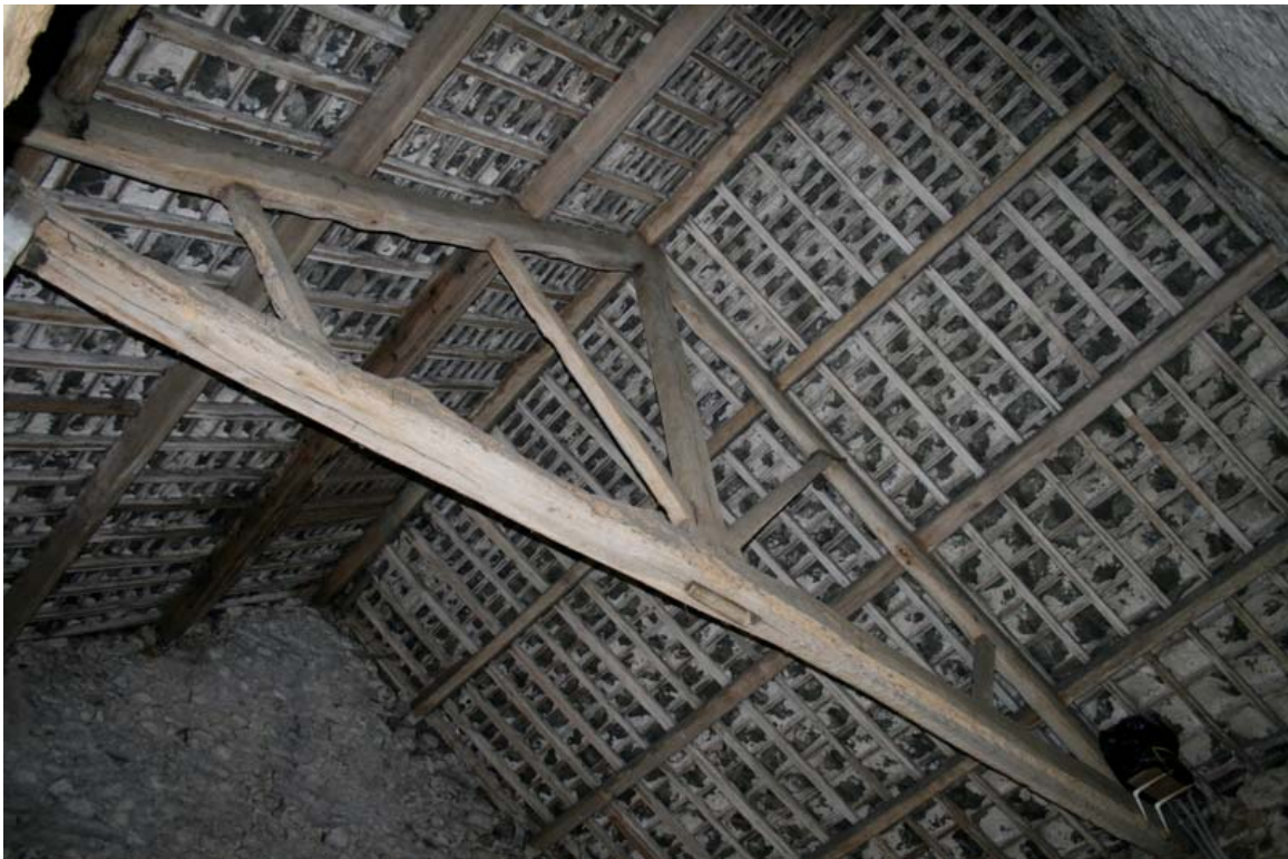
Plate 36: King post truss, and under-sealed slate roof, threshing barn
