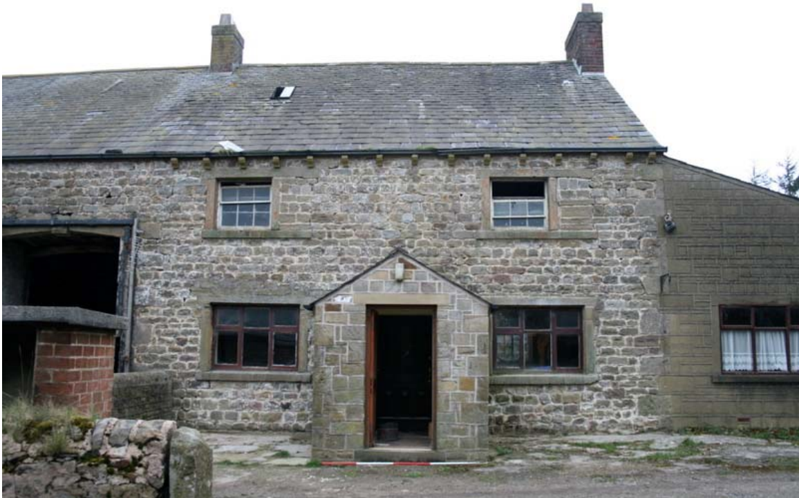
Plate 2: Façade of Cross Keys Inn
