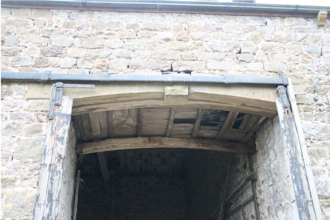
Plate 35: Dressed sandstone lintel and dropped keystone of threshing barn
