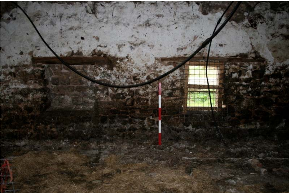
Plate 42: Keeping-hole and original window, west wall, cowhouse
