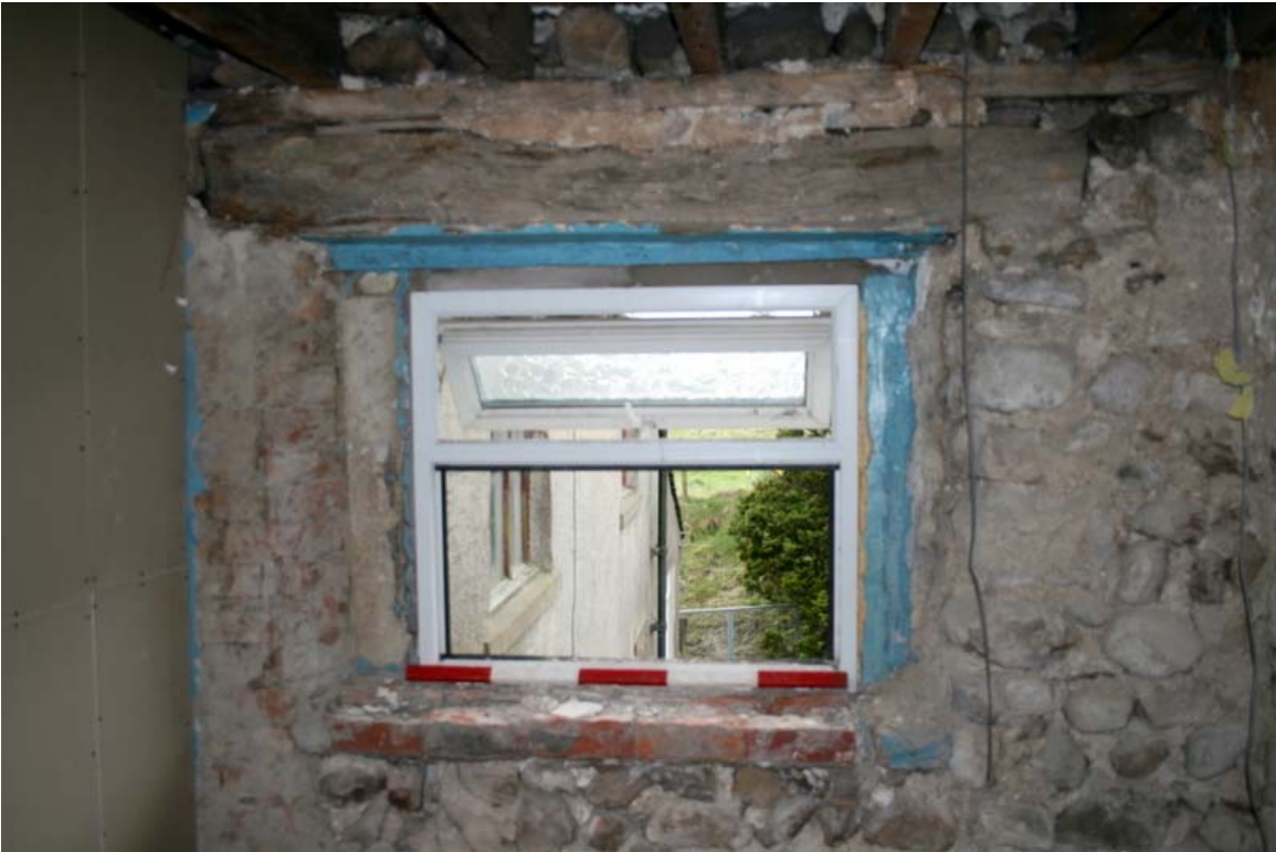
Plate 16: Window in west wall, Room F2
