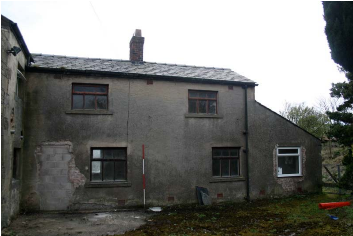
Plate 10: North elevation of western extension
