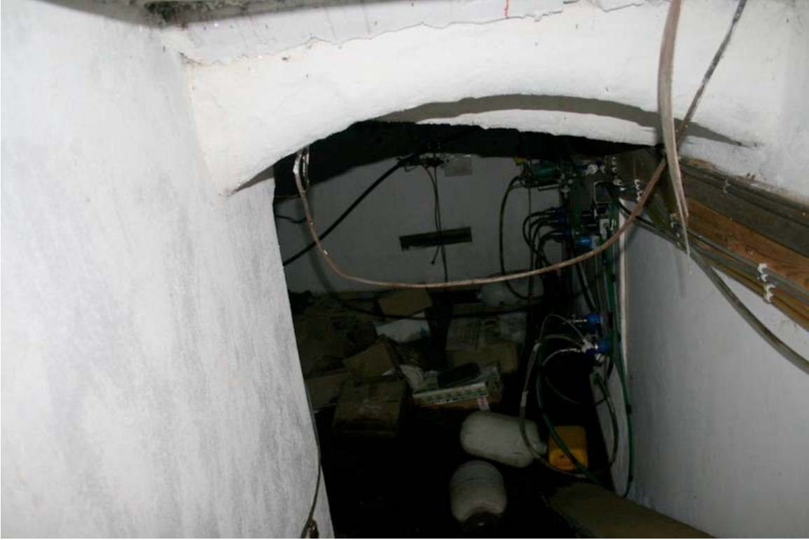
Plate 33: Entrance into brick-vaulted cellar
