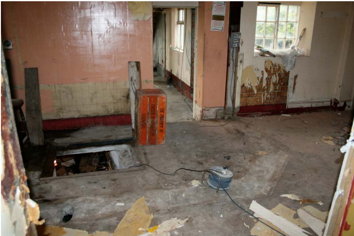
Plate 8: Floor scar for bar and entrance to cellar, Room G1
