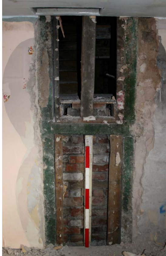
Plate 27: Blocked original stair window, Room F8
