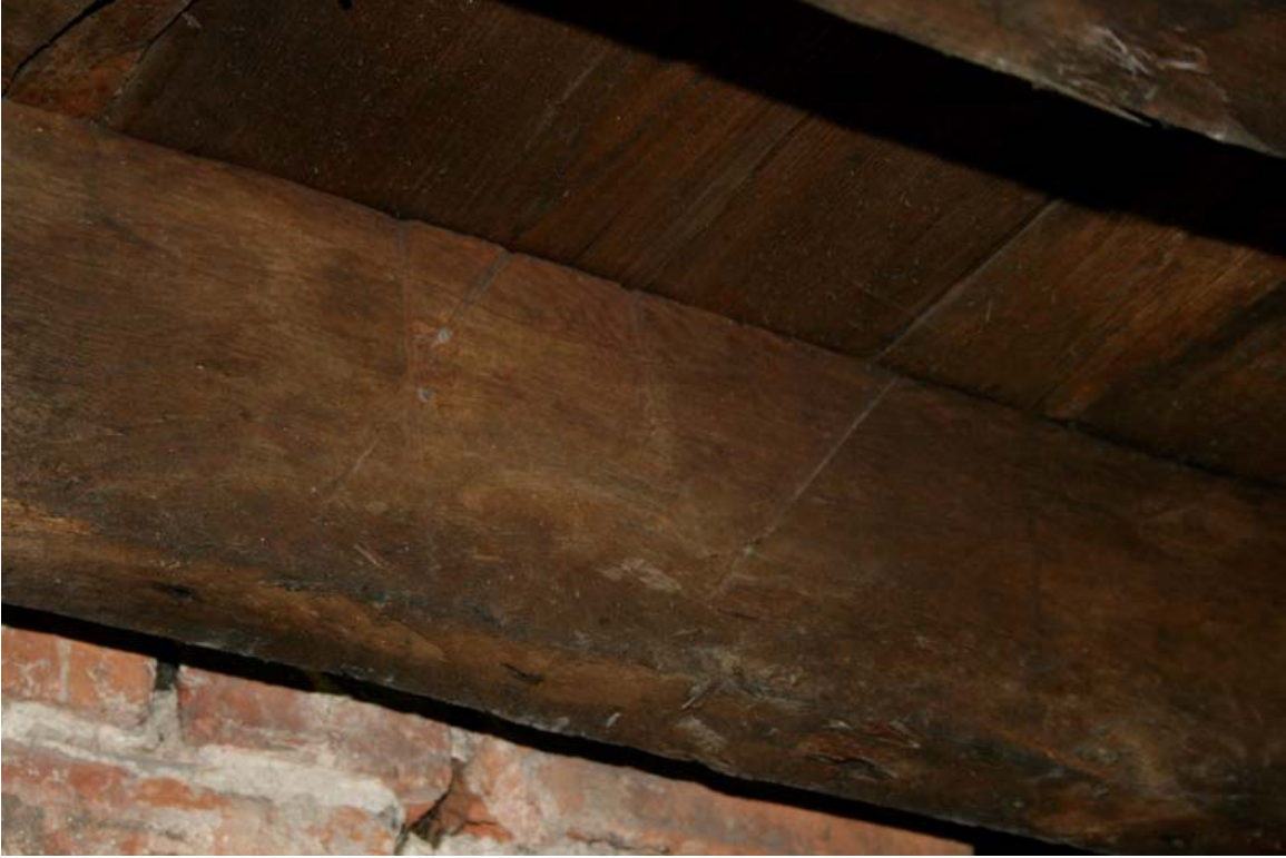
Plate 25: Baltic Timber mark, Room F5
