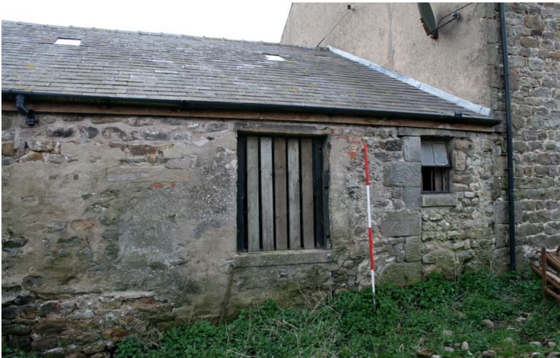
Plate 40: Front elevation of cowhouse, with blocked door and window
