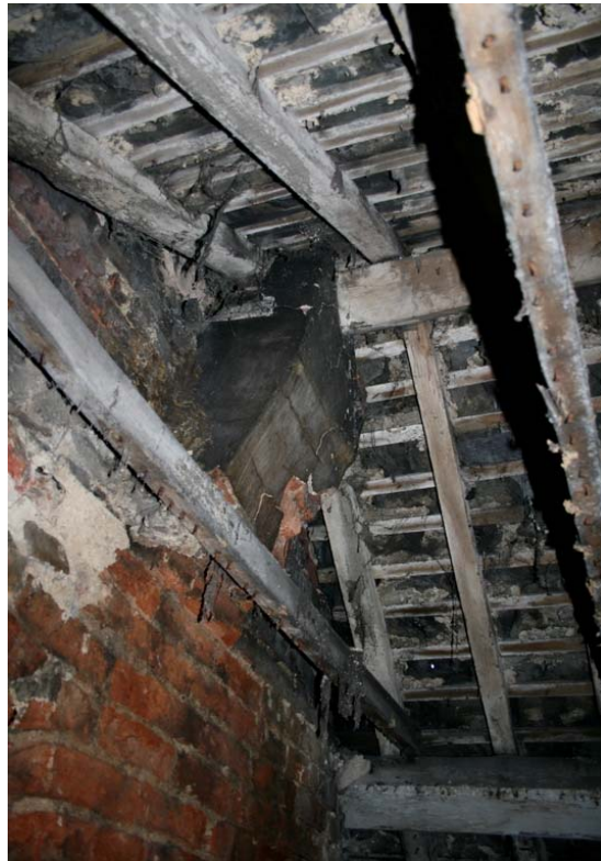
Plate 30: Corbelled stack, Room S2
