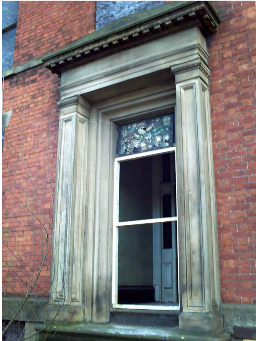
Plate 4: The aedicular doorway on the north elevation
