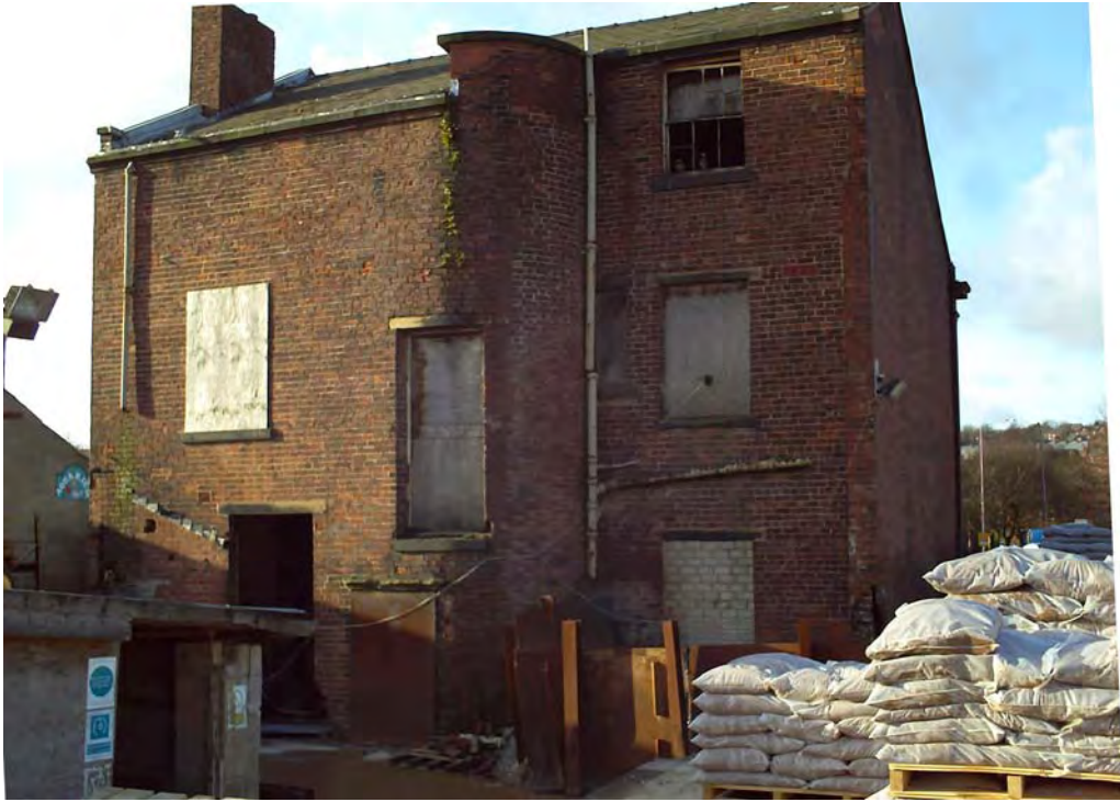
Plate 2: The rear (south) elevation of 53 King Street
