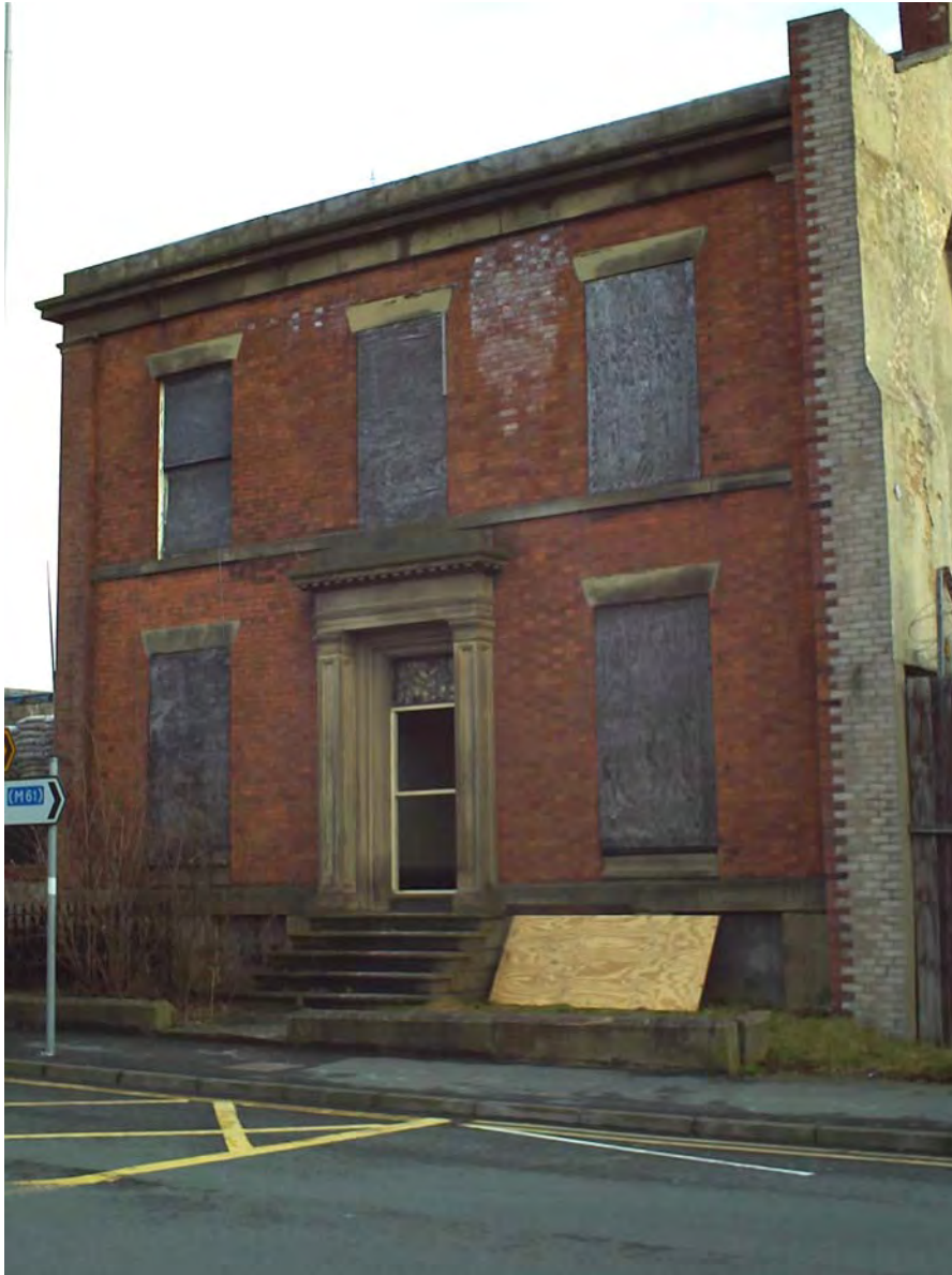
Plate 1: The front (north) elevation of 53 King Street
