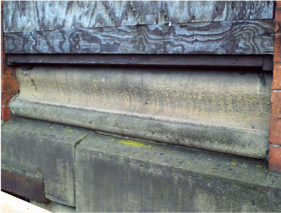
Plate 5: Detail of the moulded sills on the front elevation
