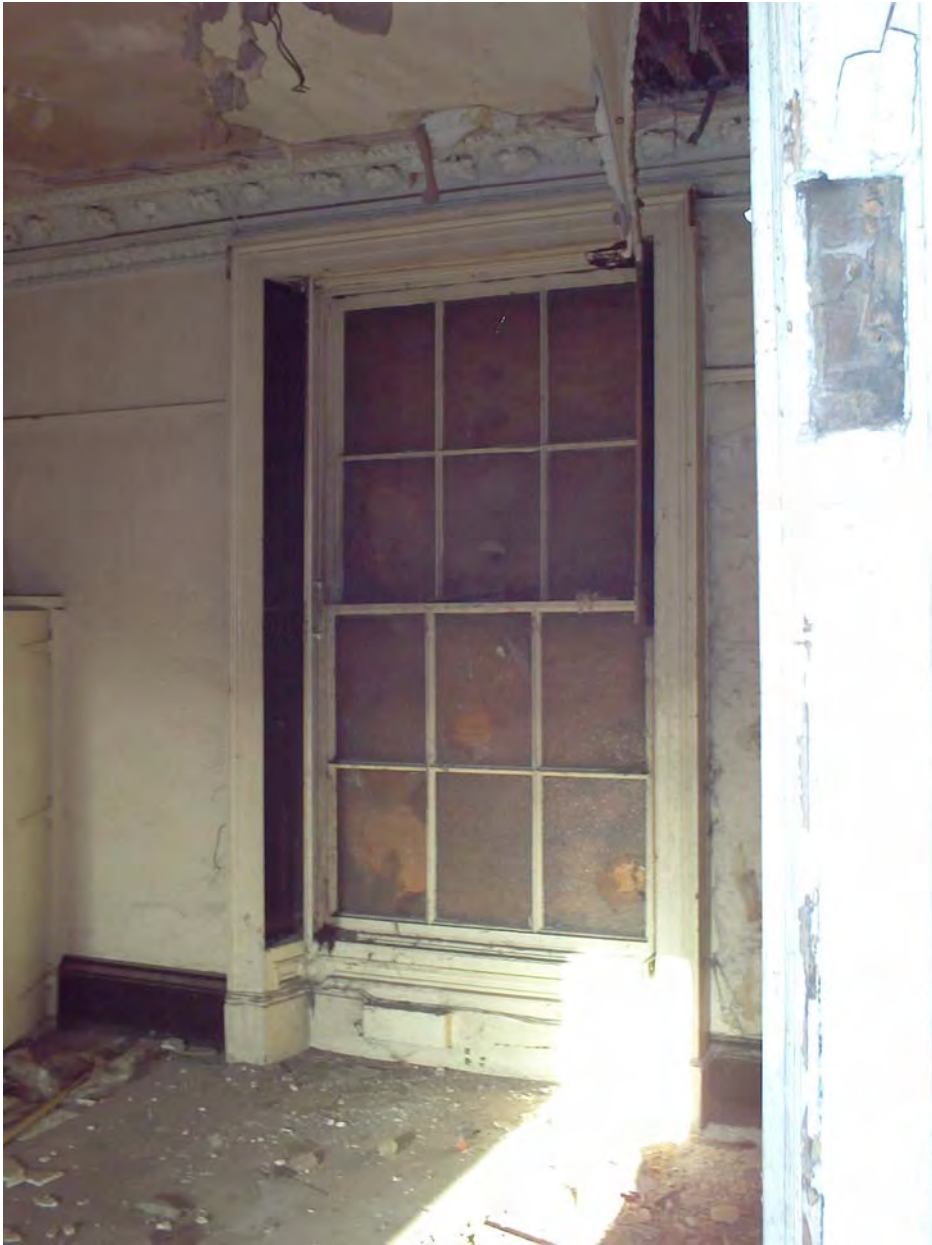
Plate 13: The sash window within room 5
