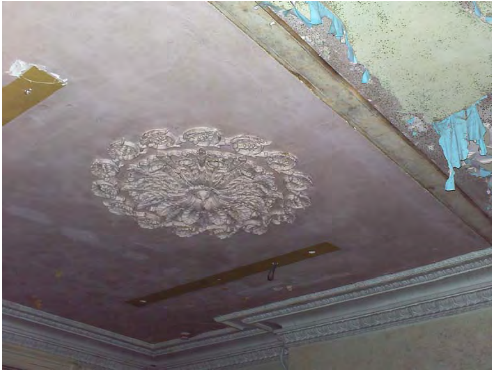
Plate 9: The ceiling rose in room 2, with the scar of the former partition to the right of the frame
