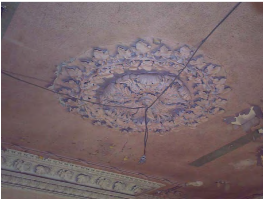
Plate 8: Detail of the ceiling rose in room 5
