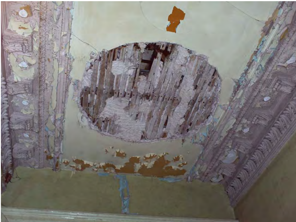
Plate 12: The scar of the former ceiling rose within room I
