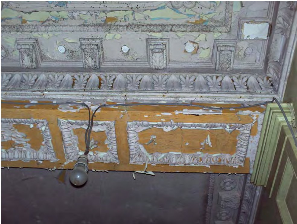
Plate 10: Detail of the various mouldings adorning the ceiling of the hallway (room 1 )
