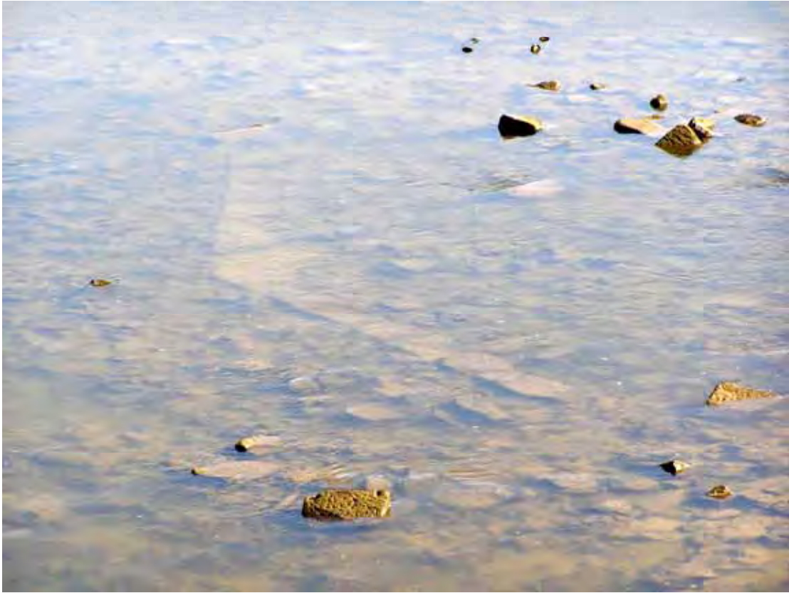
Plate 6: Exposed remnant of cutwater from the late-medieval bridge
