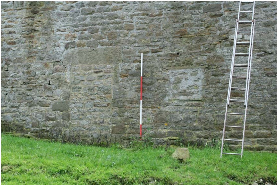
Plate 6: Blocked door and window on the north elevation of Barn A
